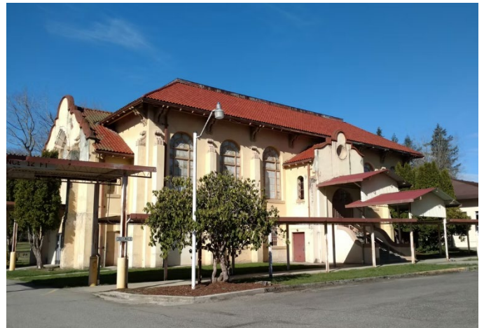
Hub Building– Source: A. Muia
