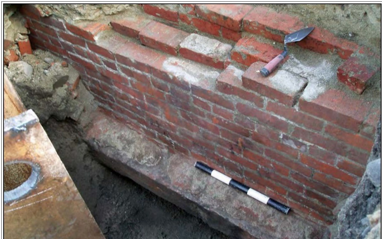
Photo C.6. Example of a historic building foundation
