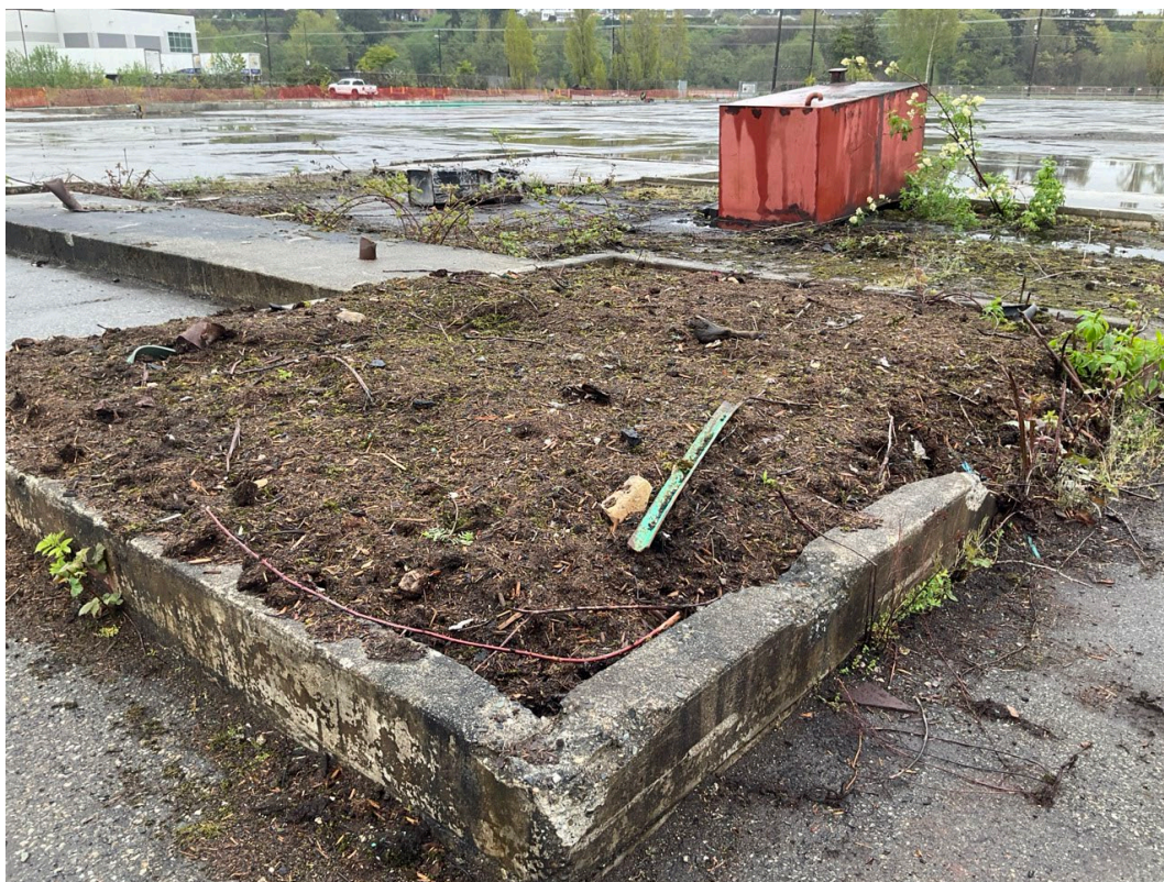
Photograph 13. Polygon D1: exposed soil and debris contained within a concrete berm.
