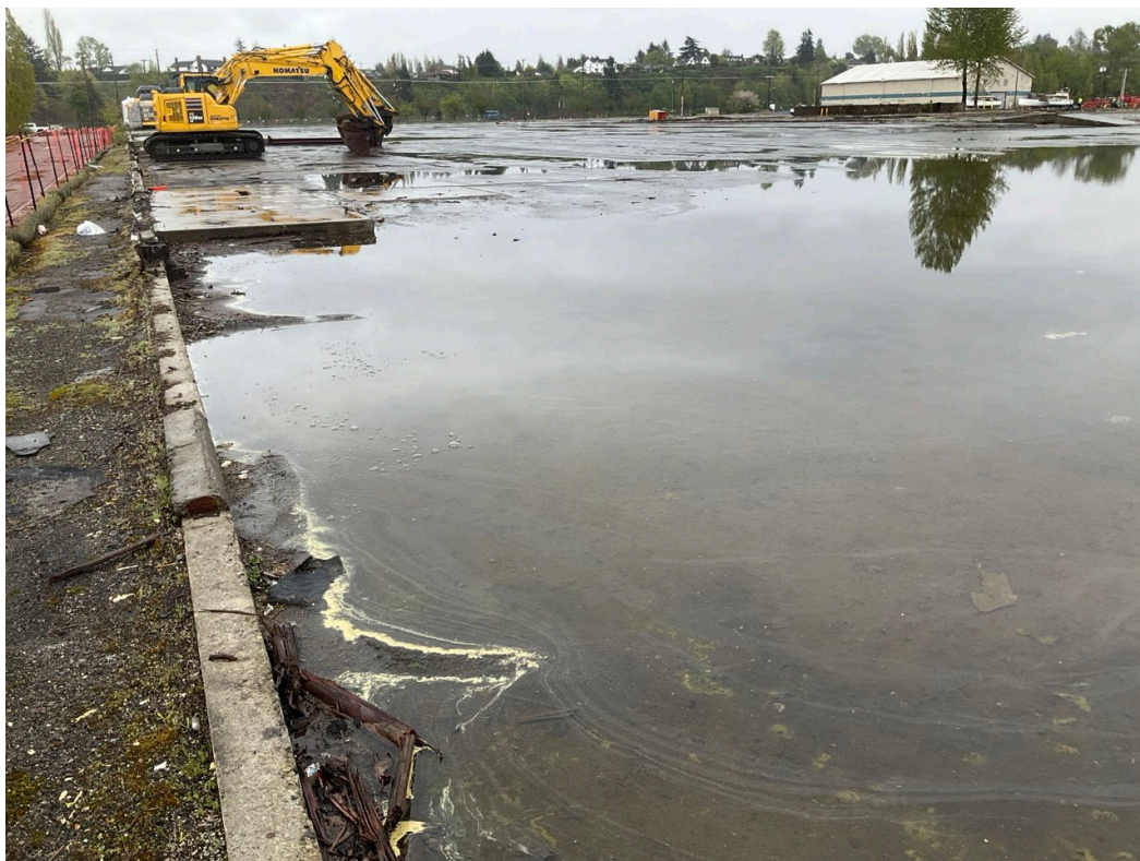
Photograph 23. Polygon F4: ponding near northwest parcel corner.
