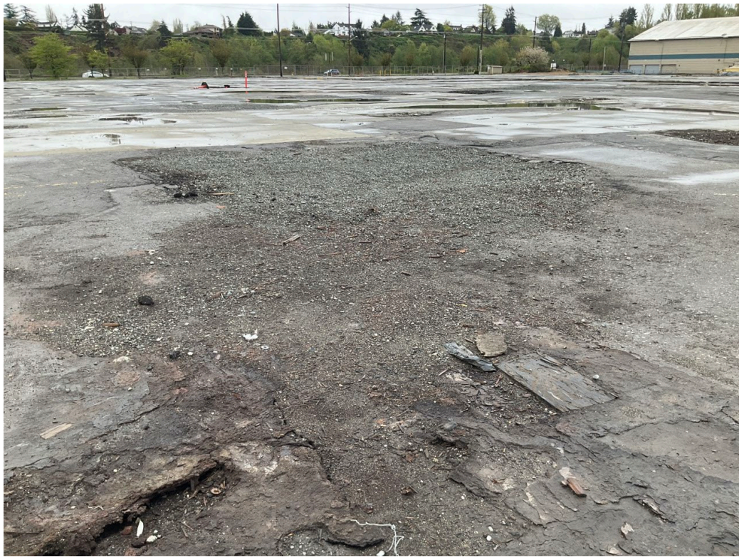
Photograph 9. Polygon C2 with crushed gravel.
