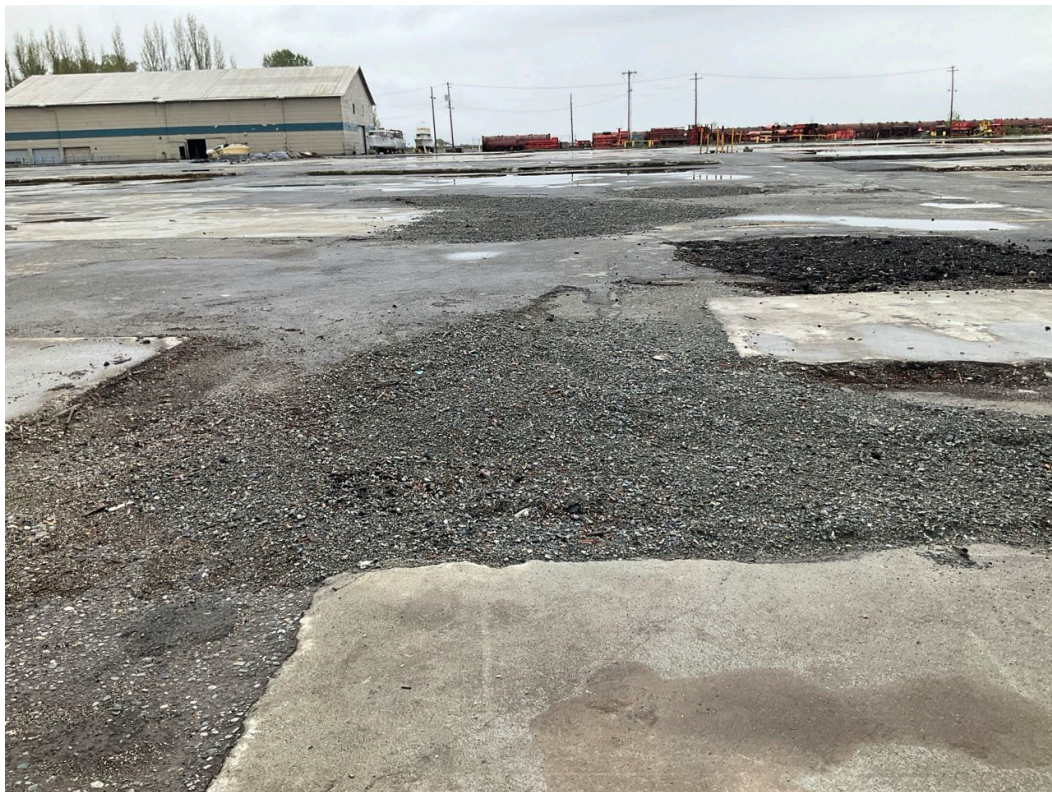
Photograph 10. Polygon C4 with crushed gravel.
