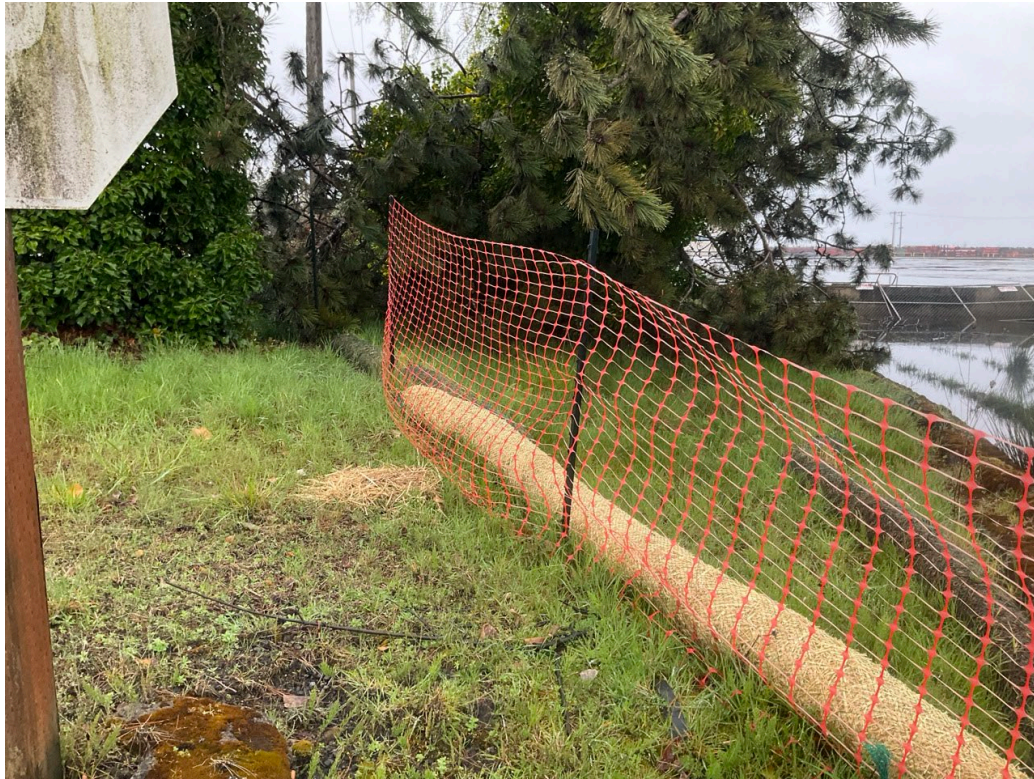
Photograph 17. Polygon E1: vegetated area near the north truck bay.
