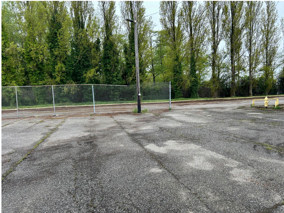
Photograph 2. Polygon A1 in southwest corner of the Site.
