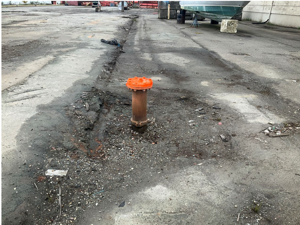
Photograph 15. Polygon D5: exposed soil between asphalt and foundation.
