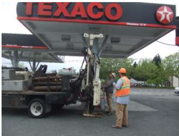
Photo 14. View of the soil boring – B6.
