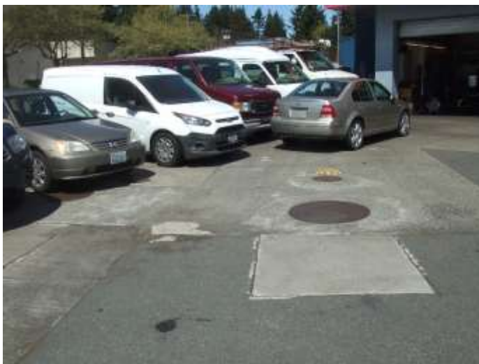
Photo 5. View of the UST pad looking north.
