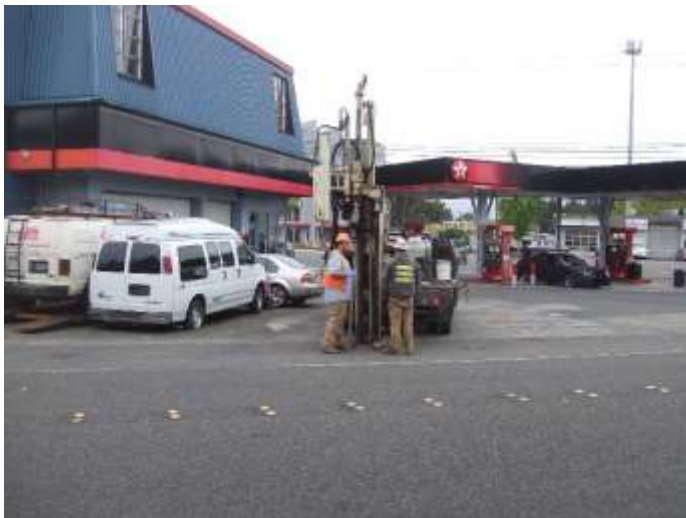
Photo 9. View of the soil boring – B1.
