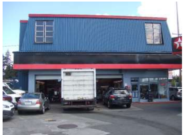
Photo 4. View of the repair shop looking north.
