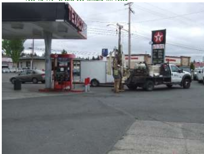
Photo 13. View of the soil boring – B5.
