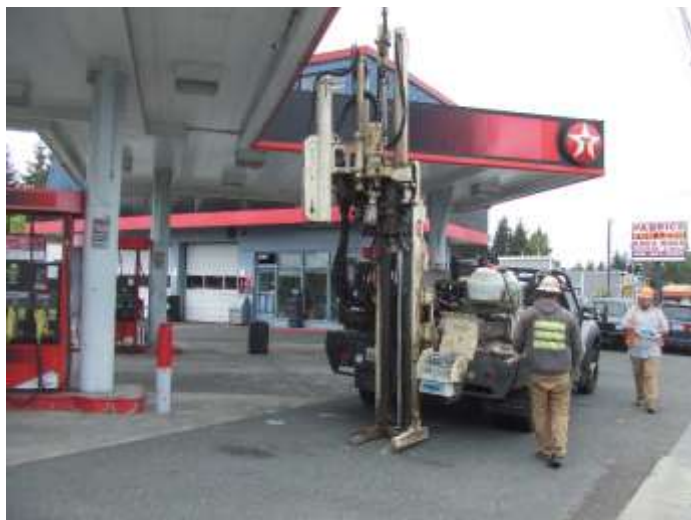
Photo 15. View of the soil boring – B7.
