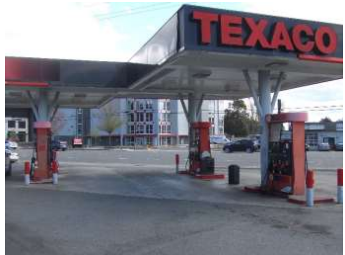
Photo 2. View of the two canopies and pumps looking east.
