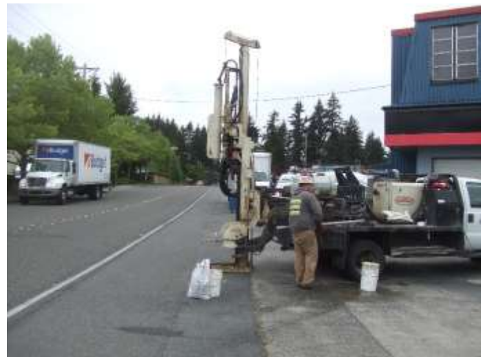
Photo 10. View of the soil boring – B2.
