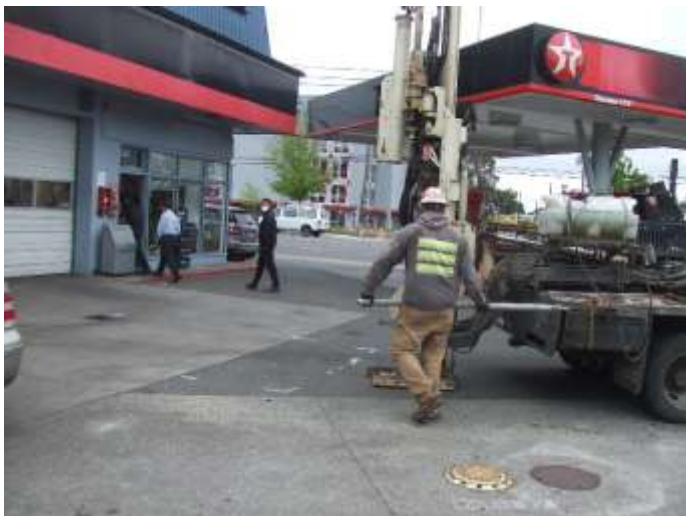
Photo 11. View of the soil boring – B3.
