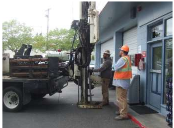
Photo 12. View of the soil boring – B4.
