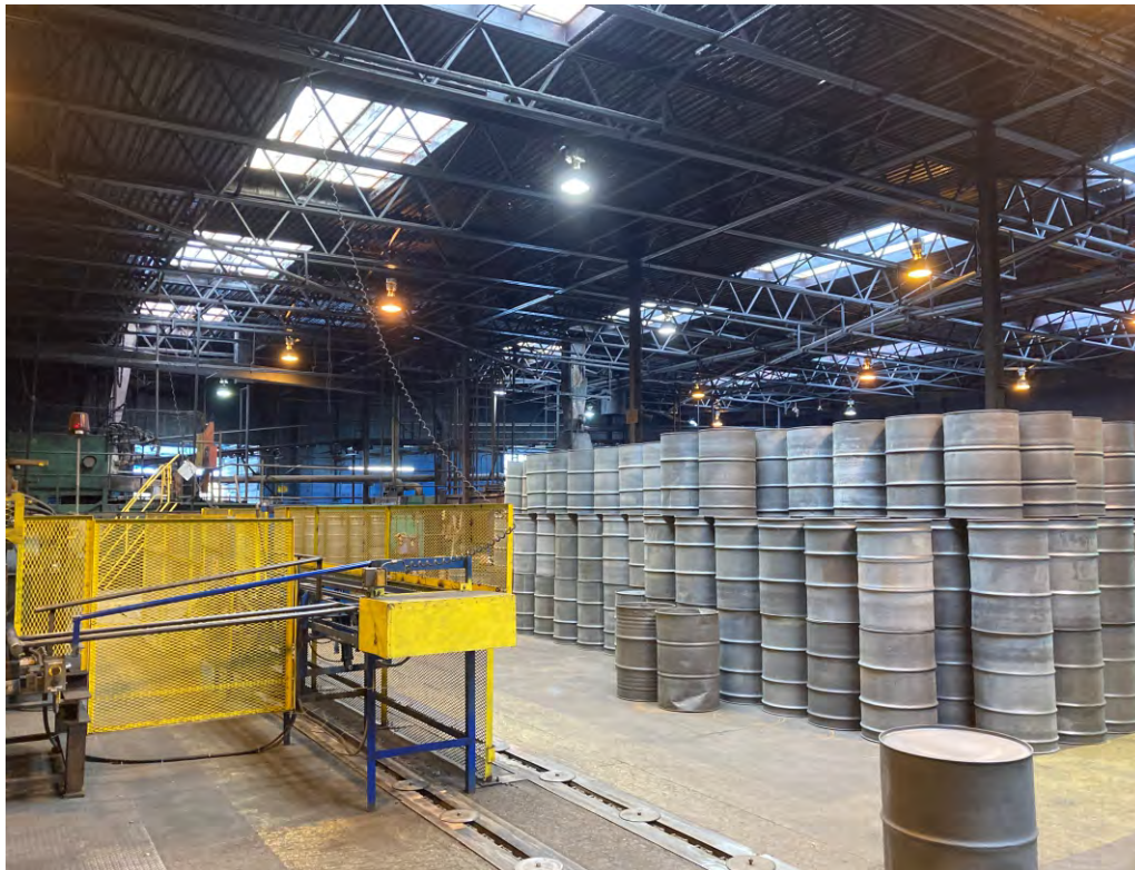
Fig. 7b - General View of Building Interior (10-2021 #1345)
