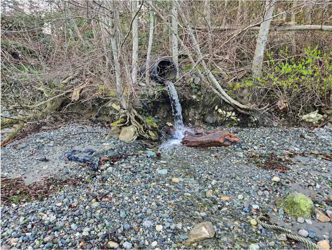
Culvert that collects the water from small waterway formed by the flow from the two pipes up slope and discharges it onto the beach along Guemes Channel.
