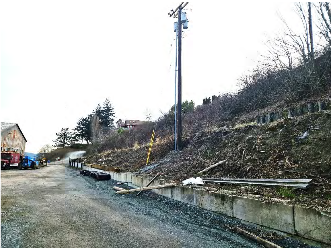
Slope mostly cleared of vegetation between the main shorefront work area and the mid-slope access road.
