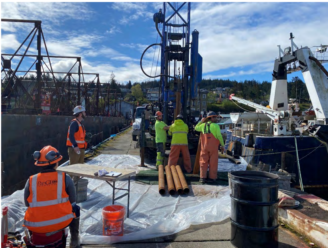
Drill rig operating over location PG-1.
