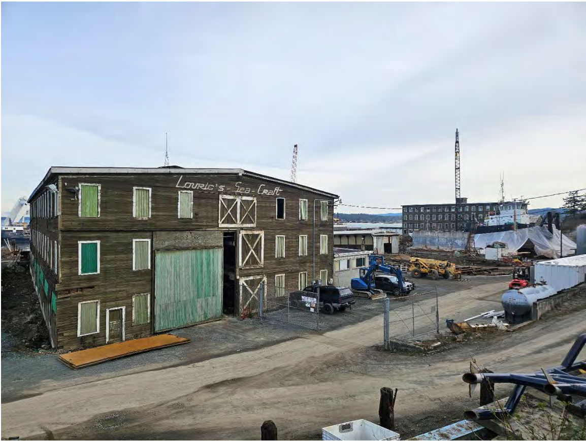
The front of the west warehouse, looking northeast.
