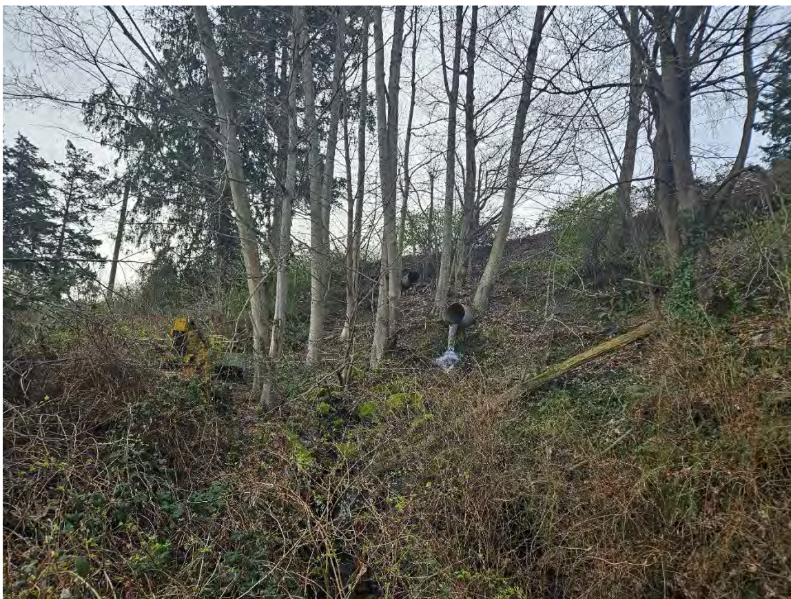
Two pipes that discharge water from off-site onto the west end of the subject property.
