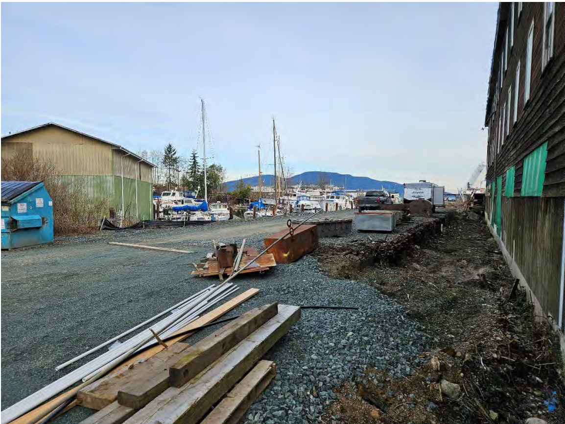
Storage area underlain by a beached barge along the west side of the west warehouse, looking north.
