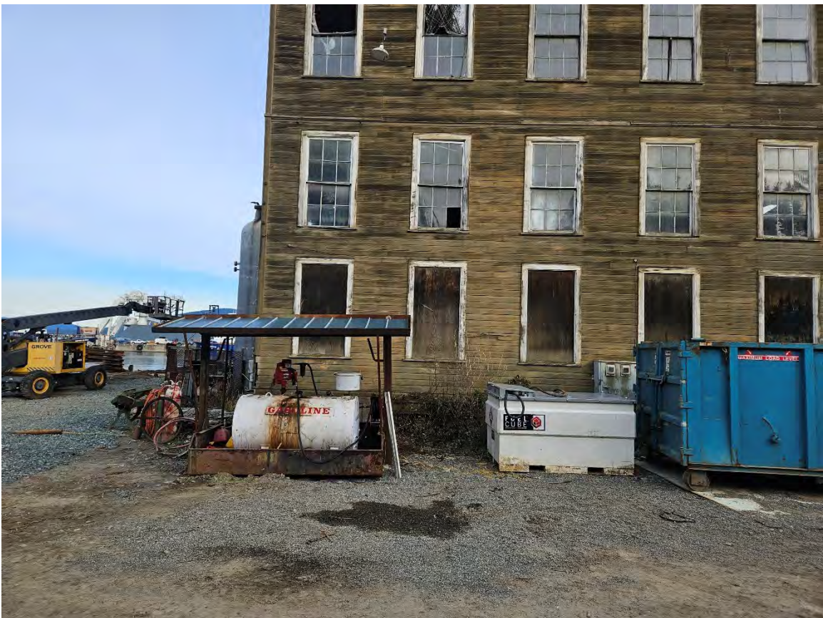
The current fueling area on the south side of the east warehouse.
