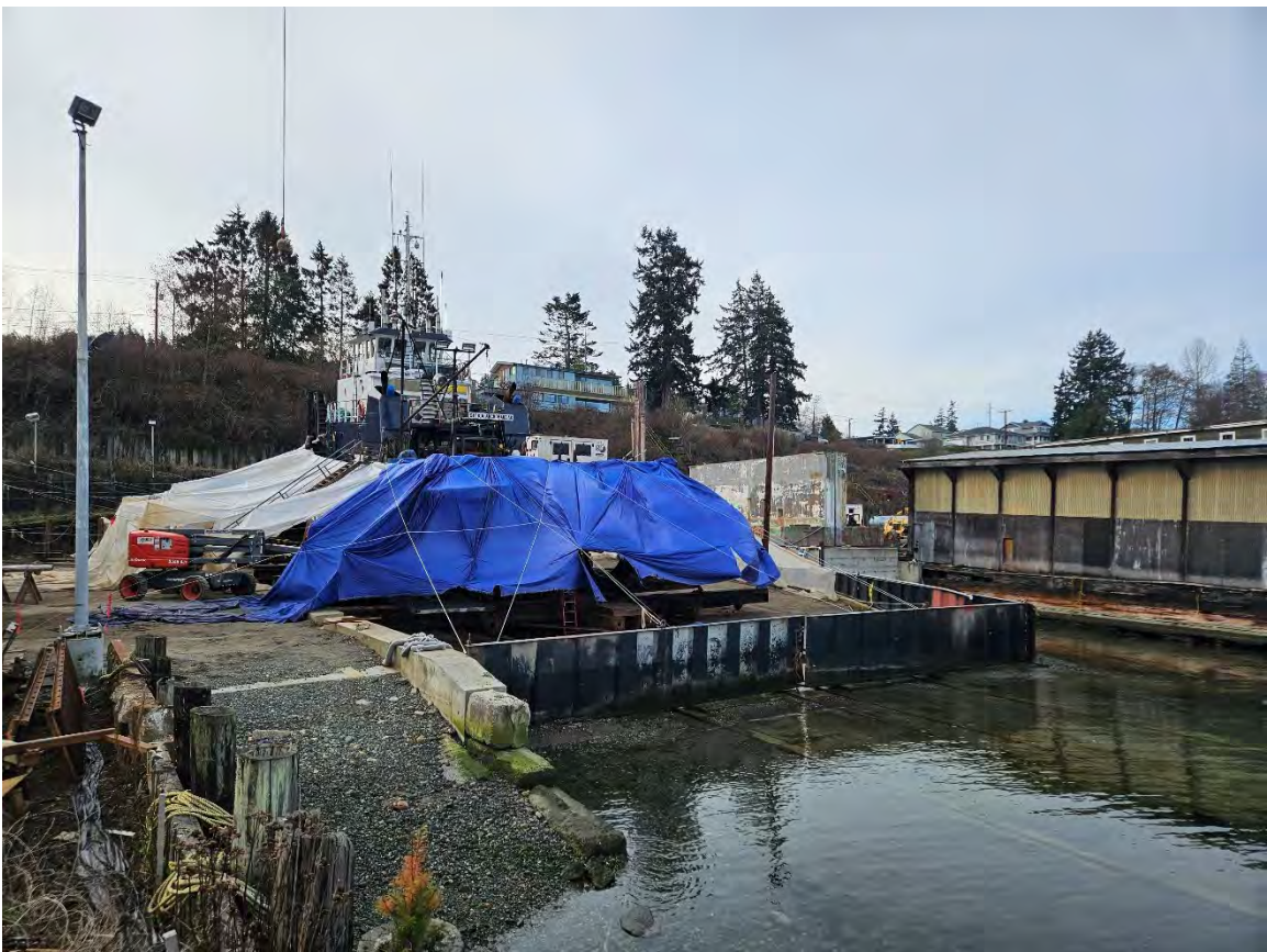
Ship being actively painted and repaired on the east railways. Note the stormwater/process water retention gates in use.
