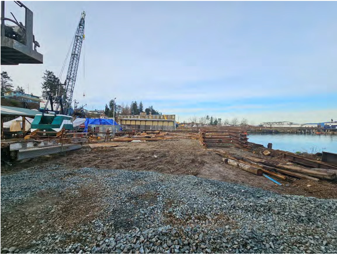
View of the former soil stockpile area (removed in 2023), looking westward.
