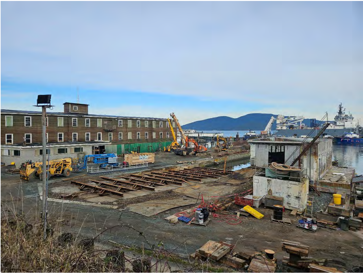
View of the west marine railways. Note the partially sunken barge (former wood shop) to the right.
