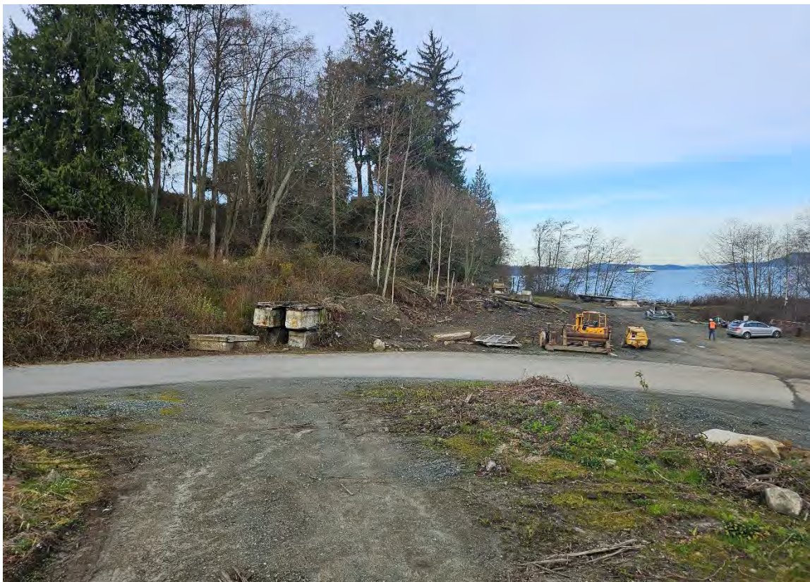
Soil stockpile at the base of the main (west) driveway, looking west.
