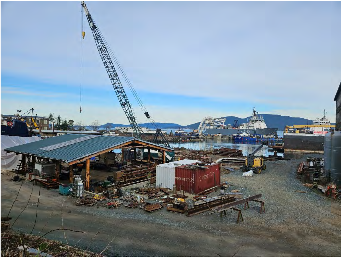
View across the metal fabrication shed and former soil stockpile area (beyond the shed), looking northwest.
