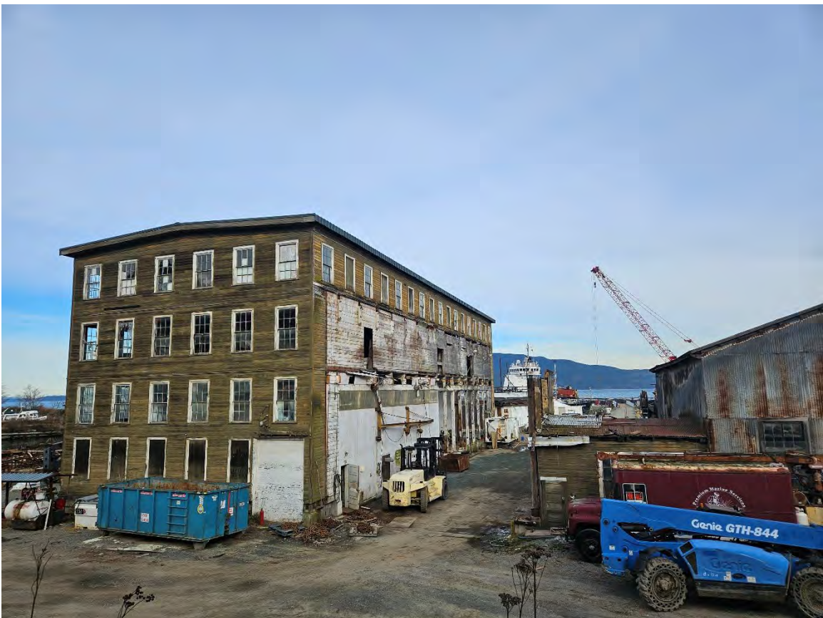
The east warehouse building, looking northwest. The tin building is in the right edge of the photo.
