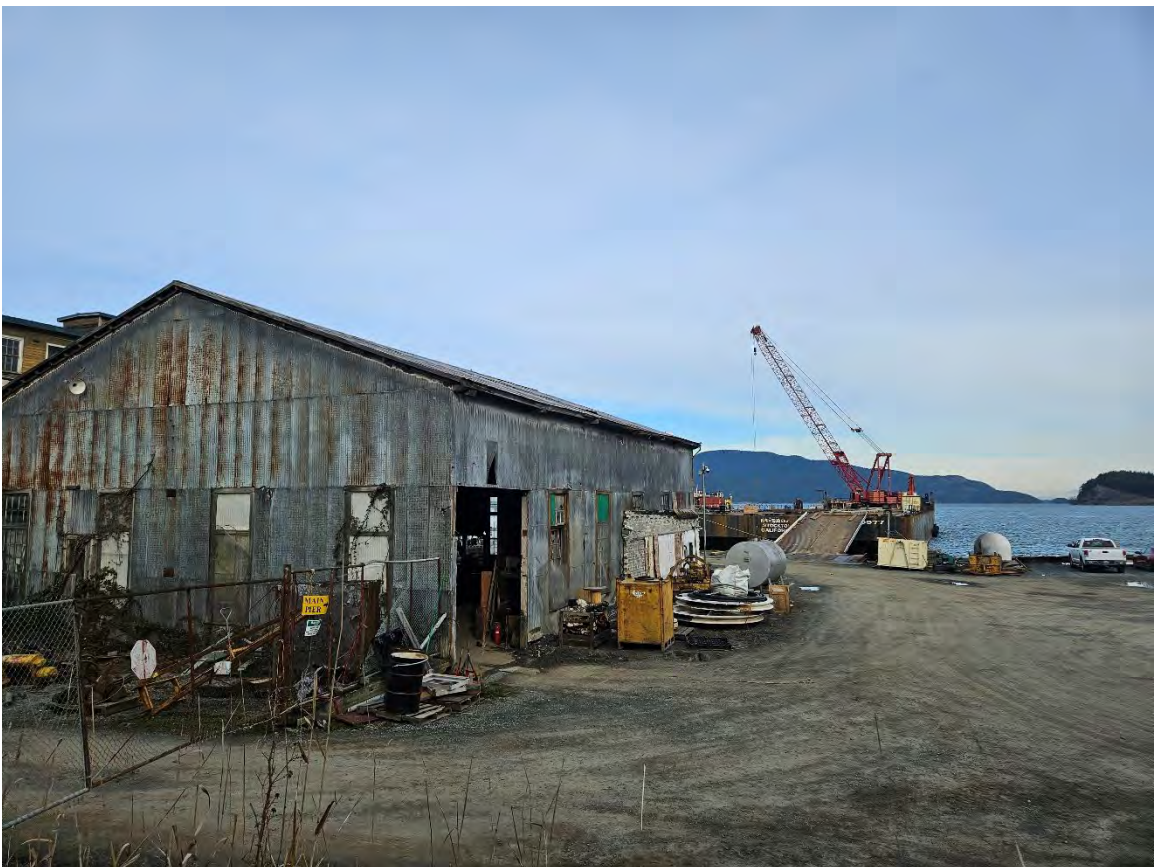
View of the east side of the tin building, looking north. Lovric's eastern property boundary extends through the gravel driveway in this photo.
