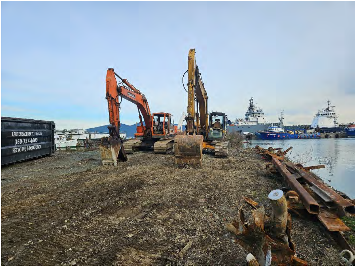
Location of the former paint storage shed northeast of the west warehouse.
