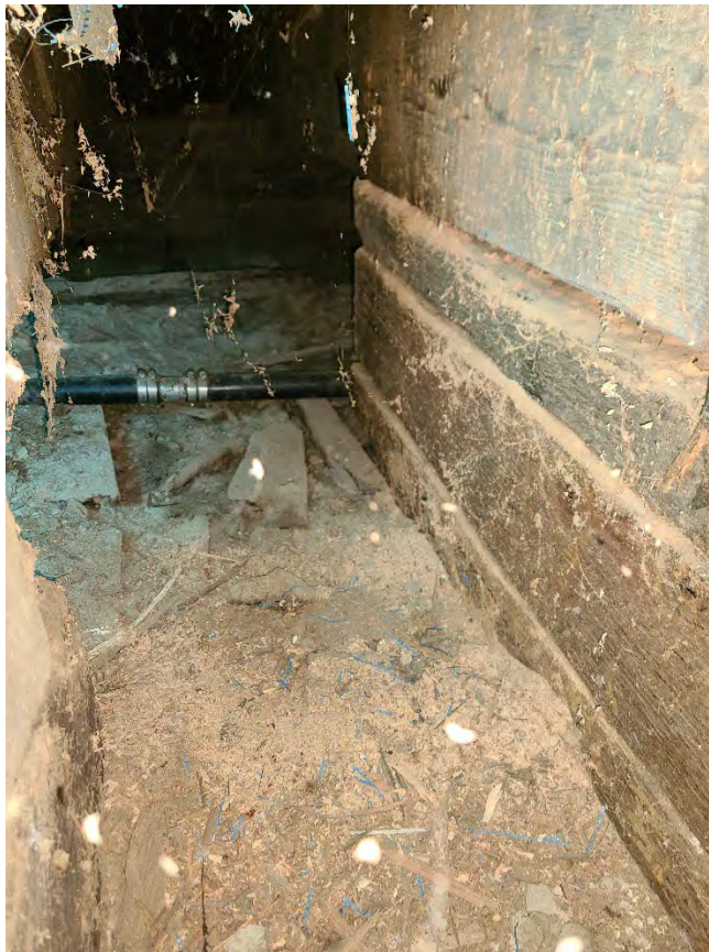
Additional view underneath the west warehouse taken by Reid Middleton engineers (6/30/2022).
