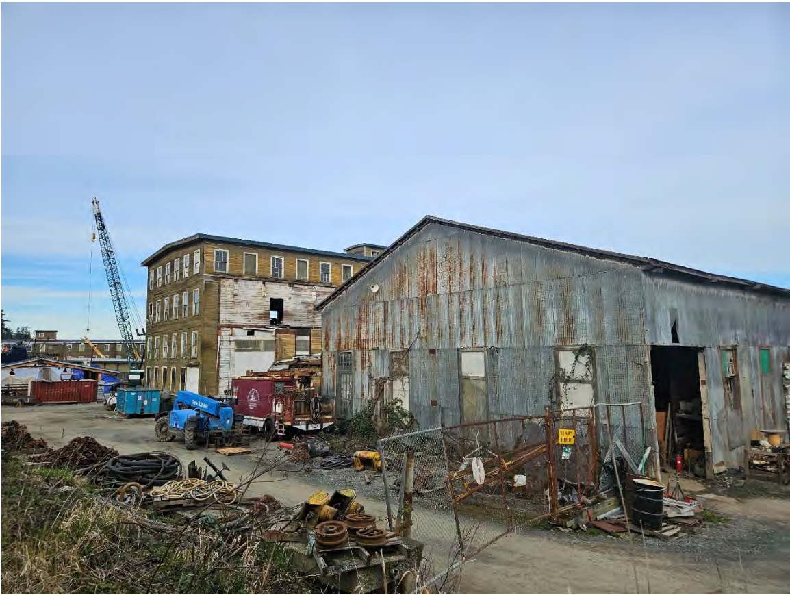
The front of the tin building, looking northwest.
