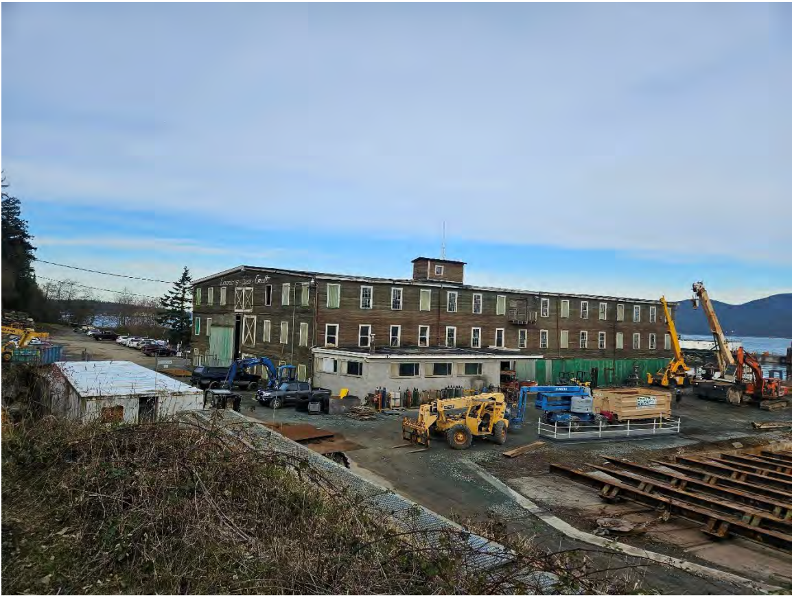
View of the west warehouse, looking west. The western marine railway is in the right side of the photo.
