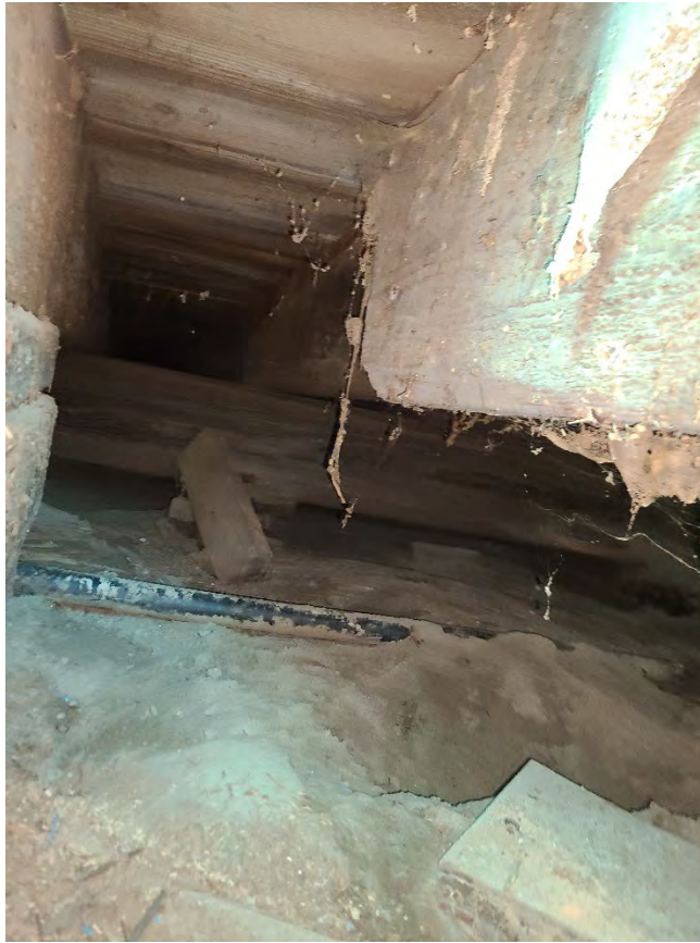
View underneath the west warehouse taken by Reid Middleton engineers (6/30/2022).
