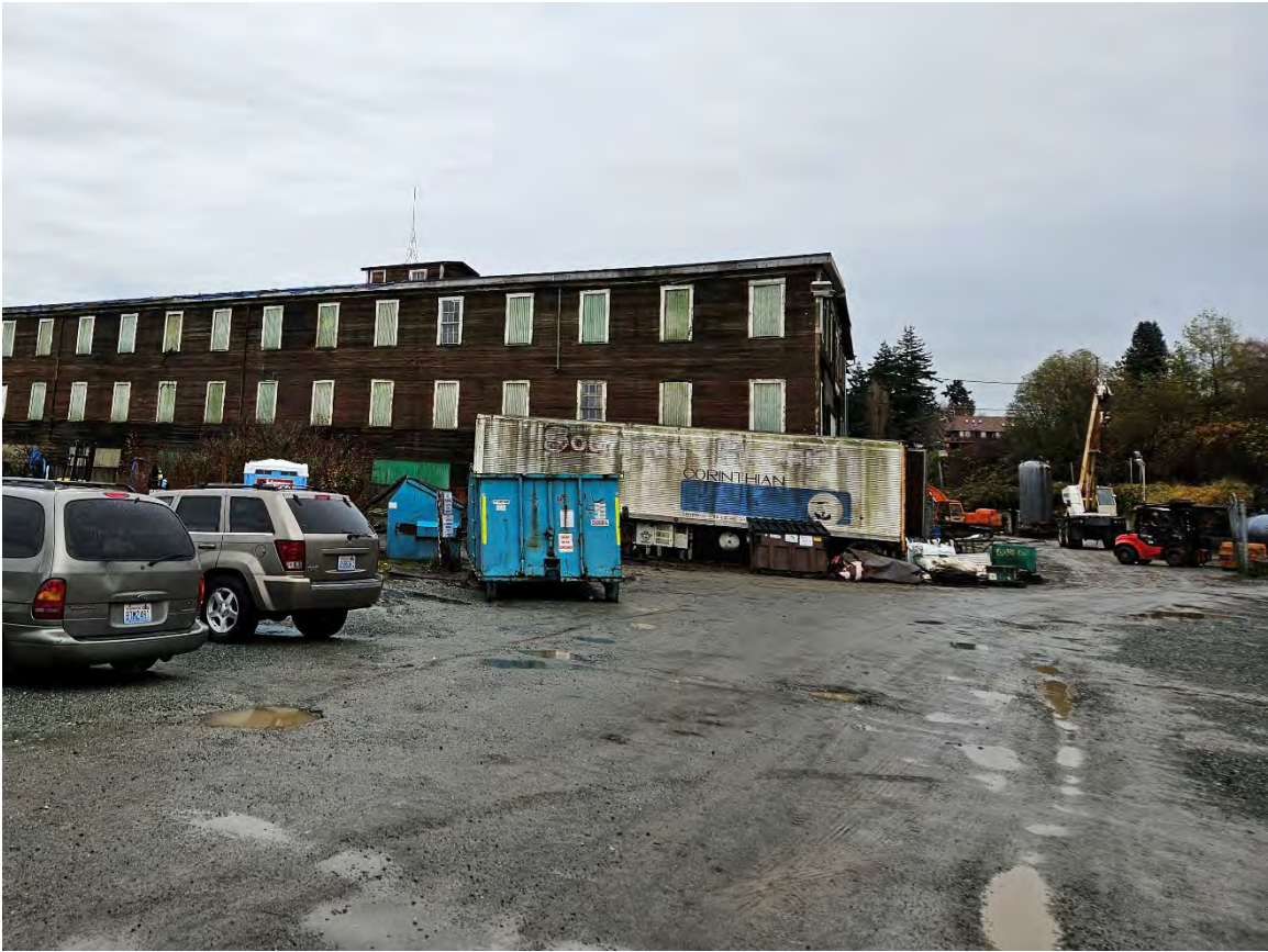
Semi-trailer of hazardous waste after it was moved alongside the west warehouse (12/5/2023).
