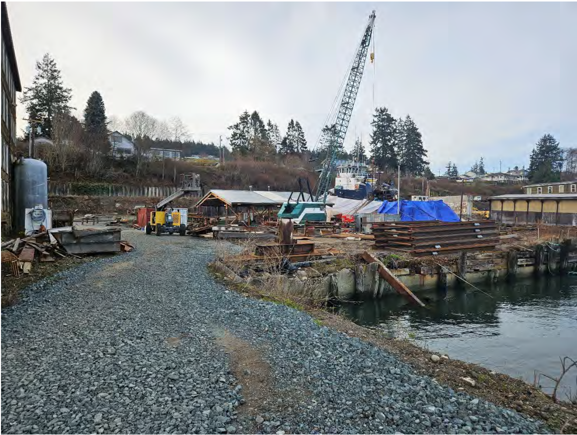
View of the west side of the east warehouse, looking south towards the metal fabrication shed.
