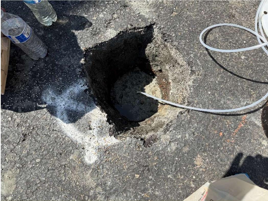
Installation of hydrated bentonite seal at GP-32S.
