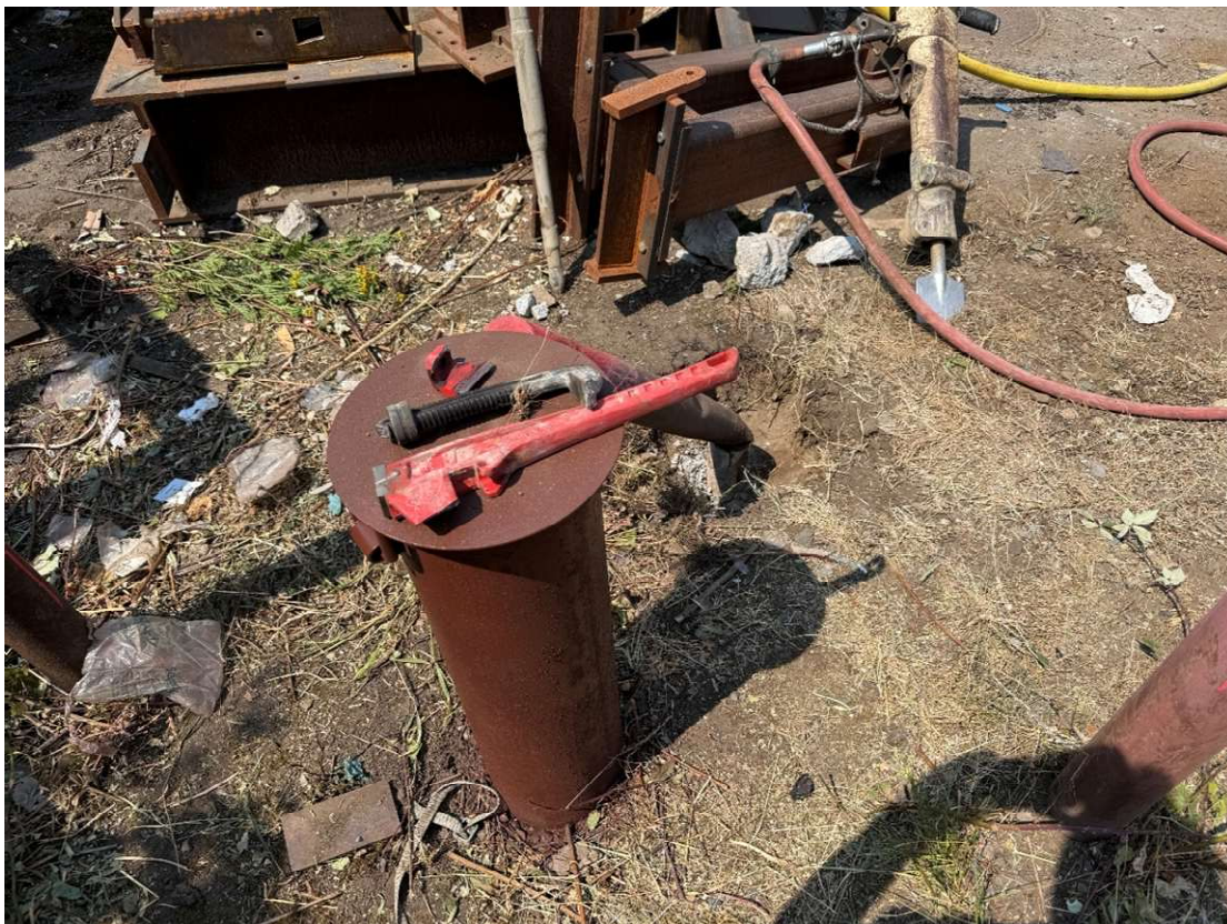
Lid hinge weld repaired, and repainted MW-24 monument.
