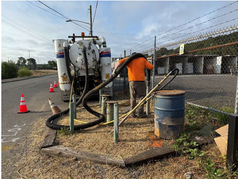
Excavation for supplemental gas probe GP-11S using vector truck and air knife.
