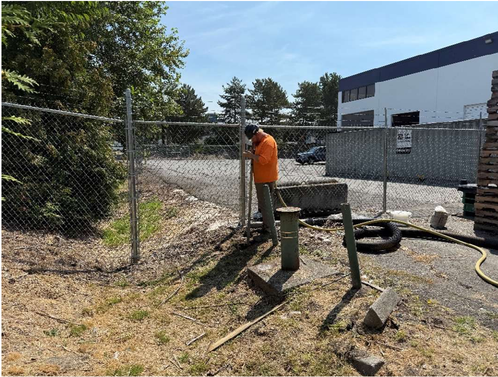
Excavation for supplemental gas probe GP-15S using vactor truck and air knife near GP-15 and drainage feature.
