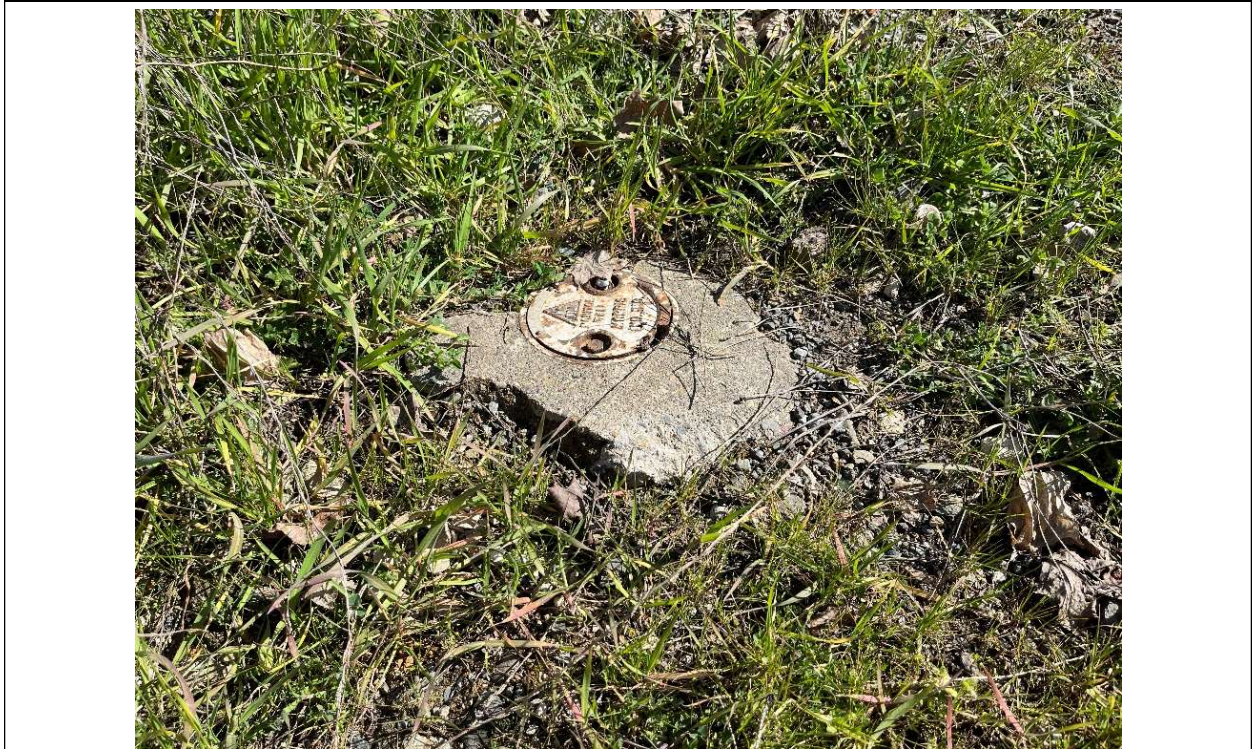
GP-28 monument prior to repairs.
