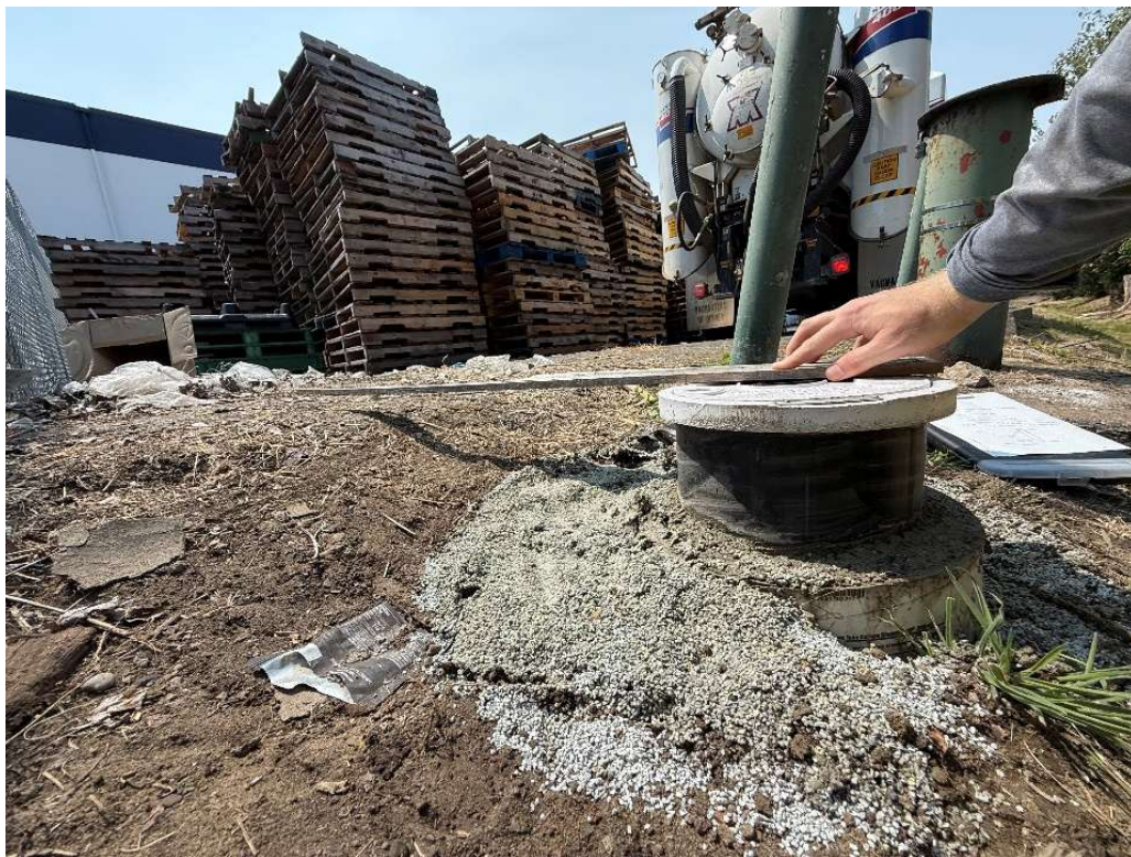
Completed supplemental probe GP-15S with sonotube, installed 1 to 2 inches above paved surface.
