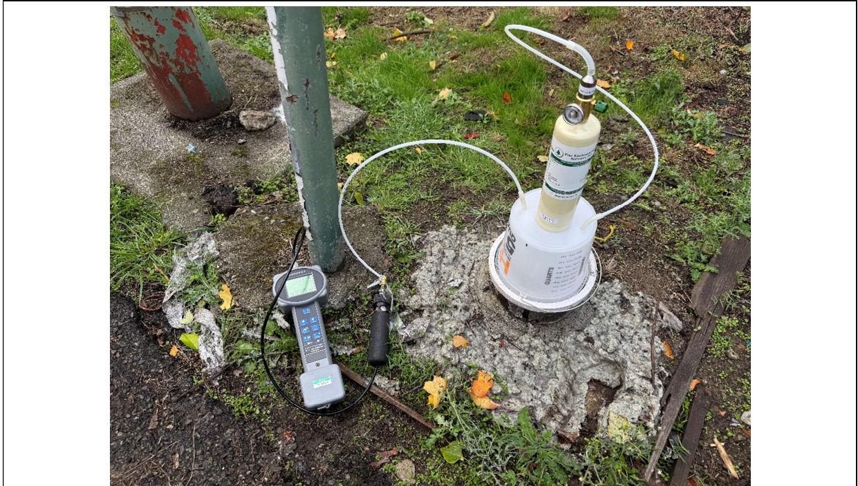
Helium leak detection testing at GP-15S.
