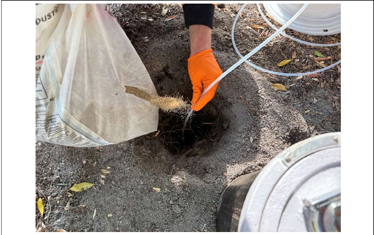
Installation of GP-13S. Wire mesh screen and LDPE tubing lowered into excavation, filter pack sand being placed above and below screened interval.
