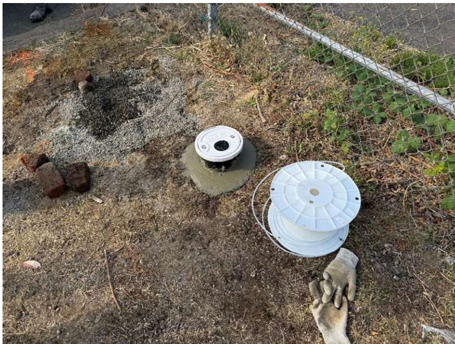
Completed supplemental gas probe GP-11S with flush-mount monument set slightly above ground surface.
