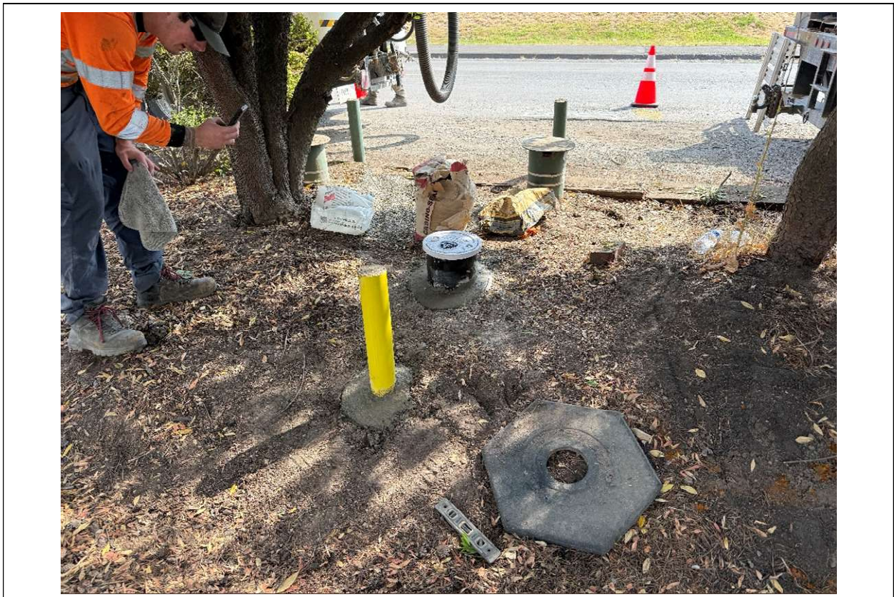
Completed supplemental probe GP-13S and installed protective bollard.
