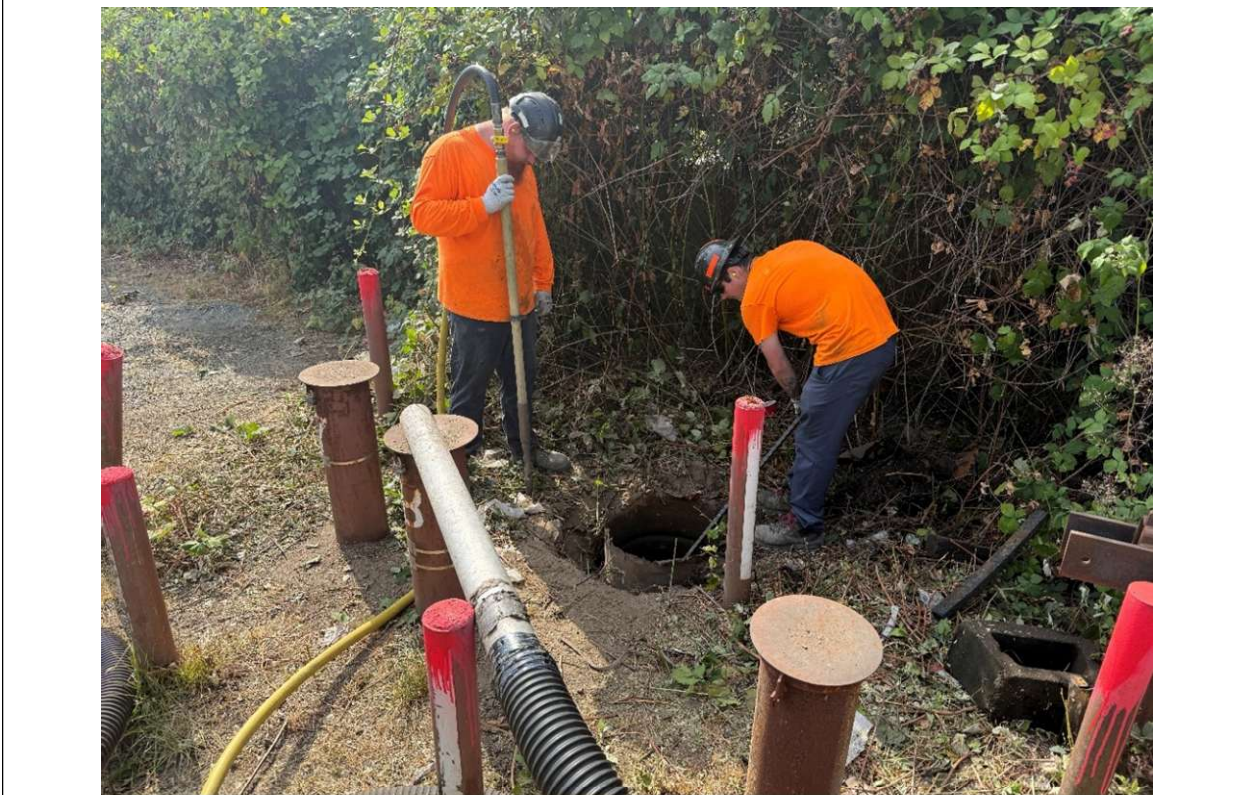
Removal of embedded and sheared drum at MW-24 location using air knife and vector truck.
