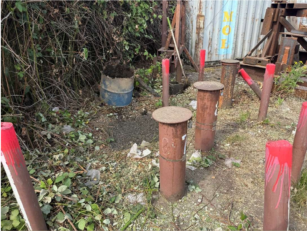
Pea gravel backfill of embedded drum depression.
