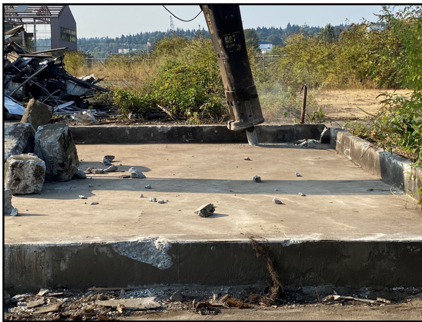
Photo CAA-02: Facing South, Slab Demolition Photo of the CAA Date Taken: 8/24/2023
