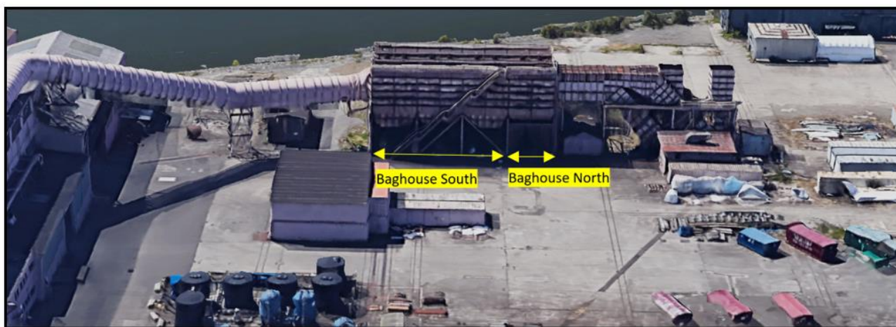
Photo 8: Baghouse Dangerous Waste Management Unit, Facing West, Adapted from Google Earth, 2008 Imagery
