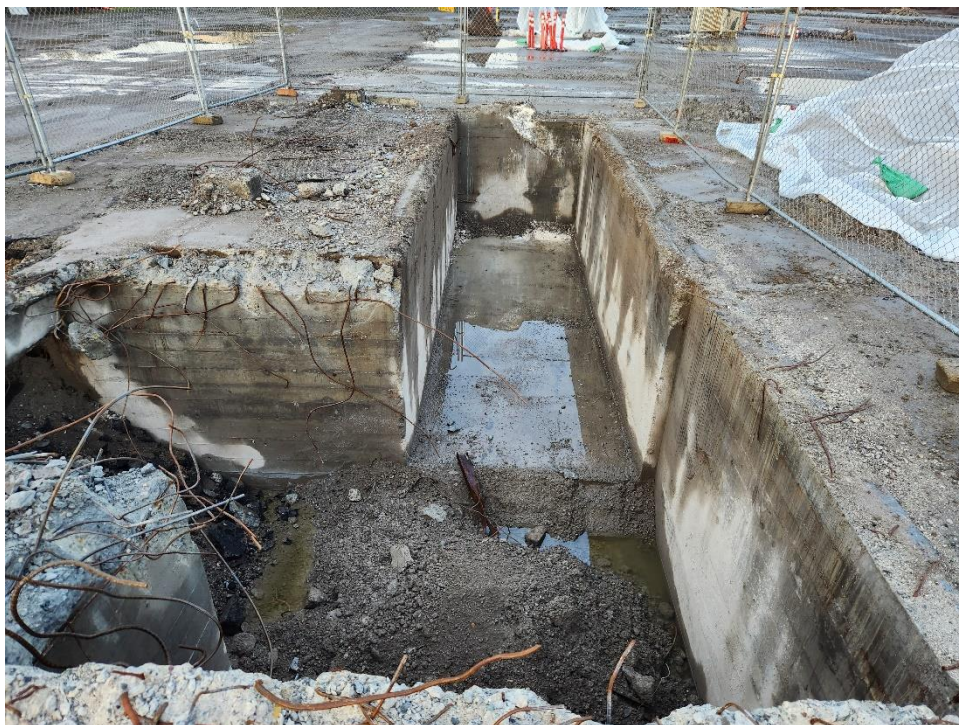
Photo 4: Powerhouse vault, west of the Powerhouse, following soil removal from the portion of the vault extending east-west. The vault contains a concrete base and sidewalls. Soil was stockpiled on plastic pending profile approval as TSCA waste to a subtitle C landfill. View to the west.
