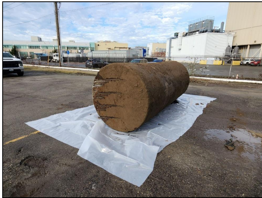
Photo 04, Facing North, Admin Building Heating Oil Tank Excavation, 1/29/2024
