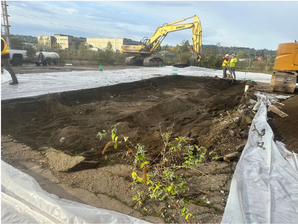
Figure 3. Overview EOD, view southwest.
