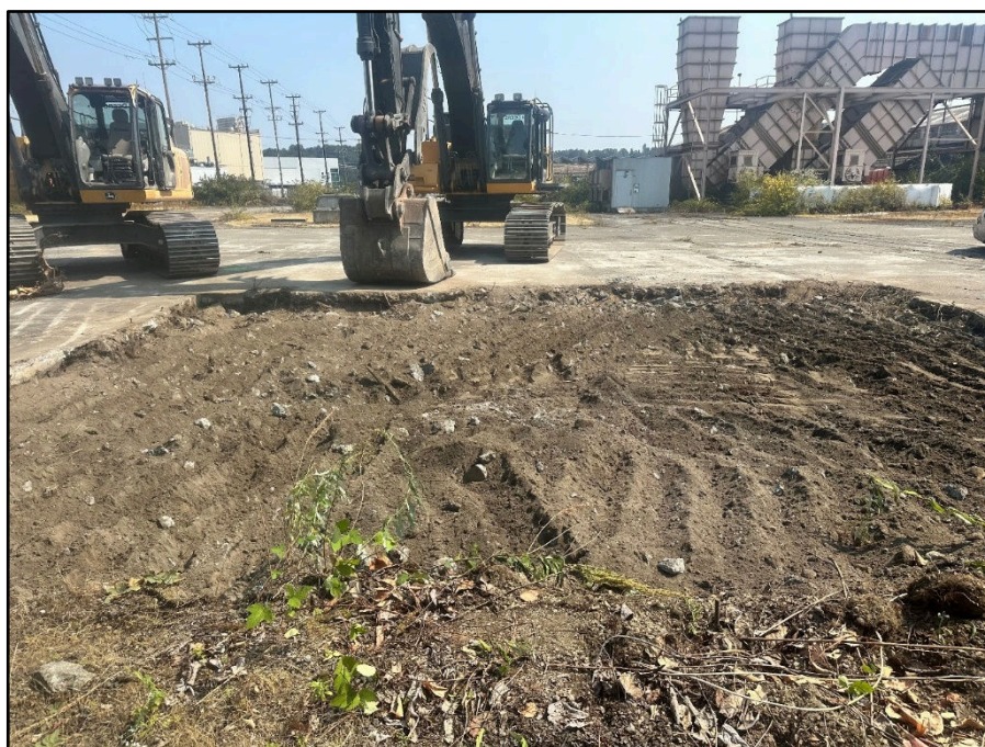
Figure 5-10. Overview Central Accumulation Area/Oil Shed, facing east
