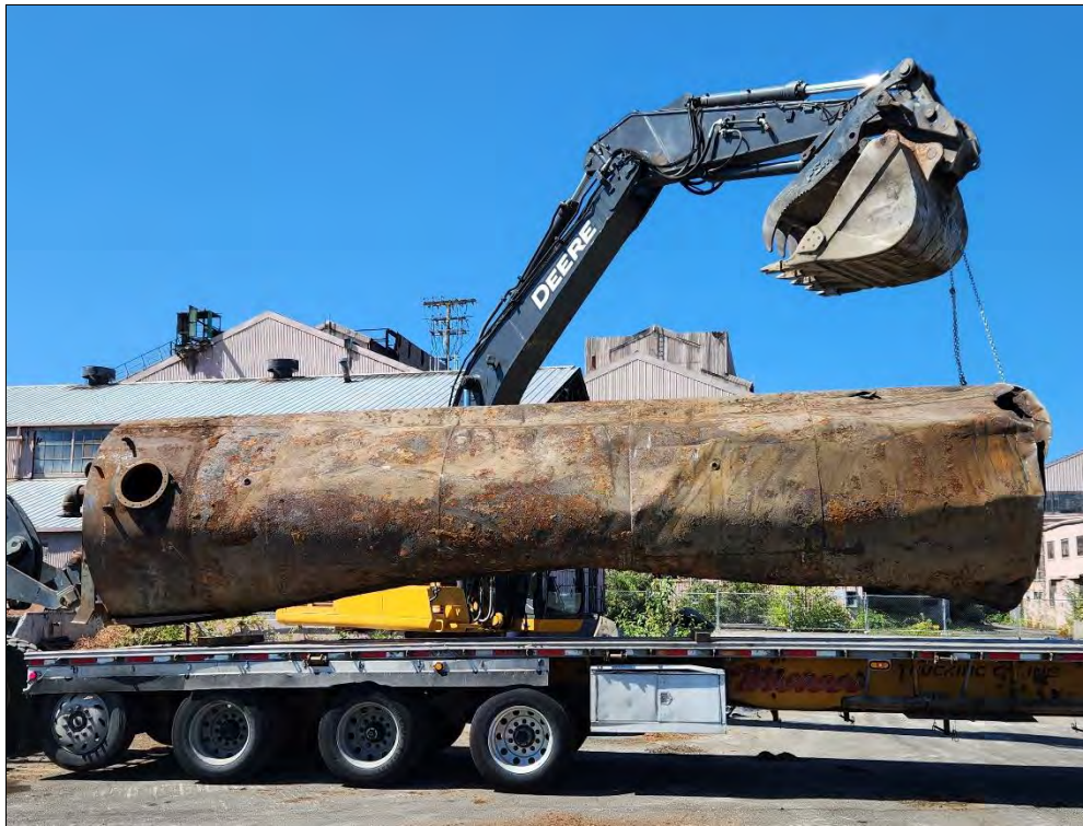
Photo 15: South Tank Vault, loading a tank for recycling. View to the west.
