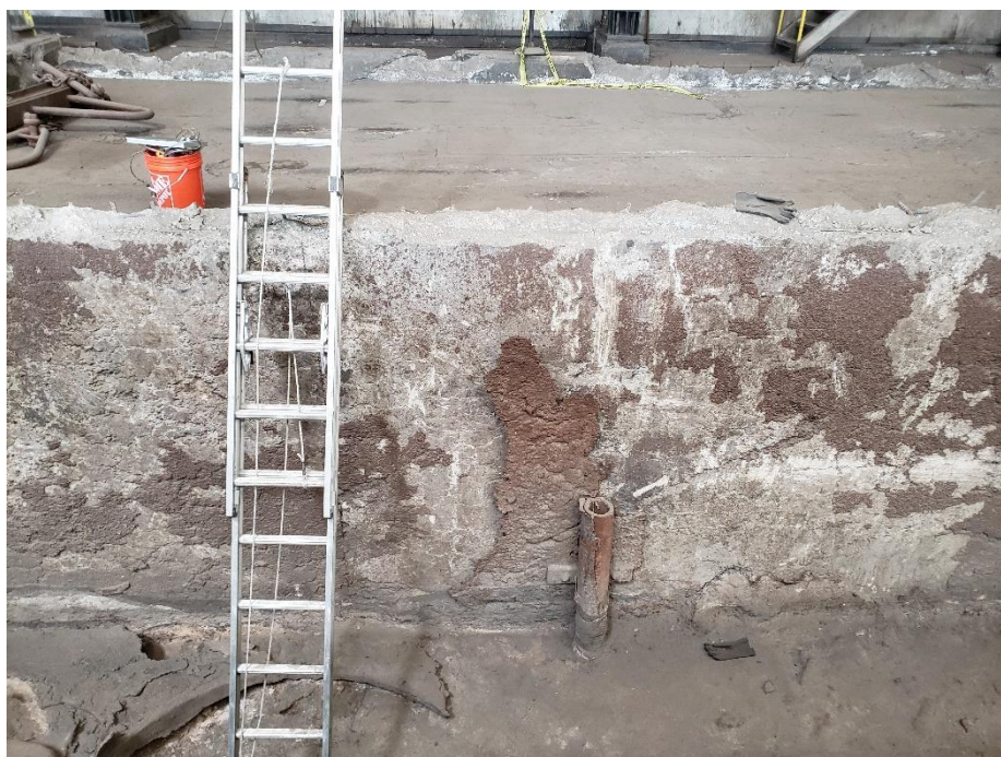
Photo 8: Sample HE-18-Pit-WC-2. Sample not marked in photo, but was collected from the rust colored slag-like material located along the north wall of the HE-18 pit (Ingot Mold Pit). View to the N.
