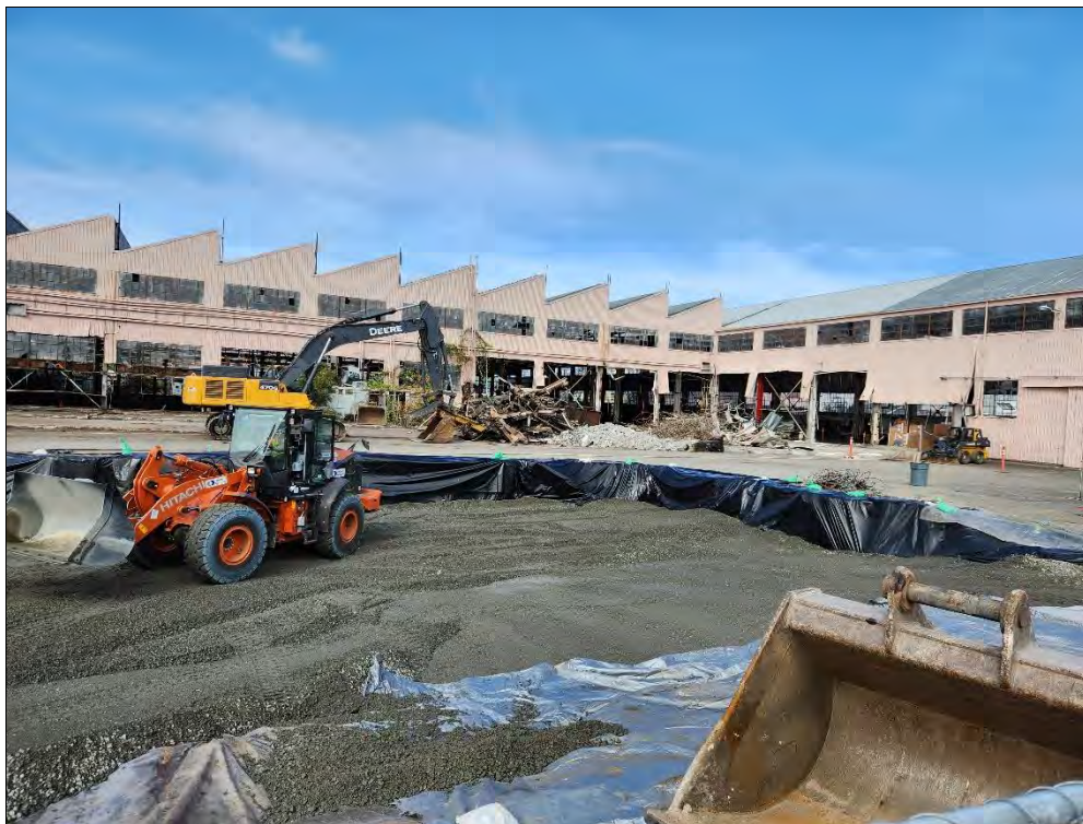
Photo 10: North Tank Vault, backfilling the tank excavation. View to the west northwest.
