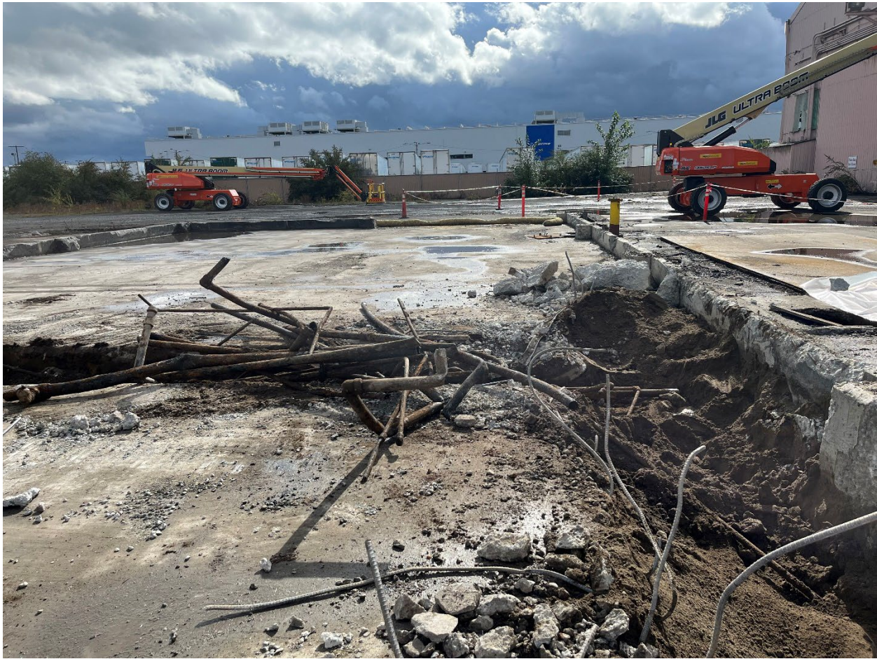
Figure 8. Pipes excavated from roughly 20 cm below surface.
