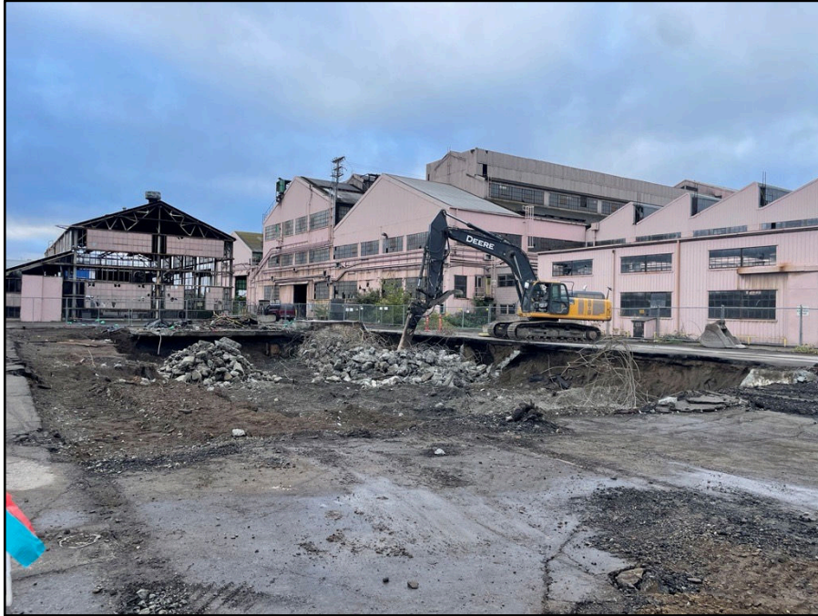
Figure 5-3. North Vault concrete wall removed, facing northwest.
