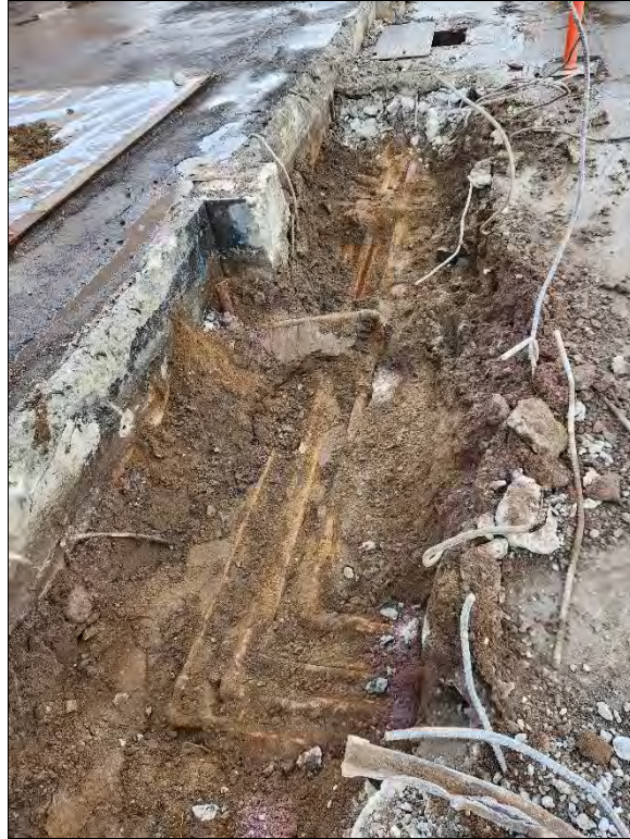
Photo 21: South Tank Vault, product piping running north towards a utilidor. View to the north.
