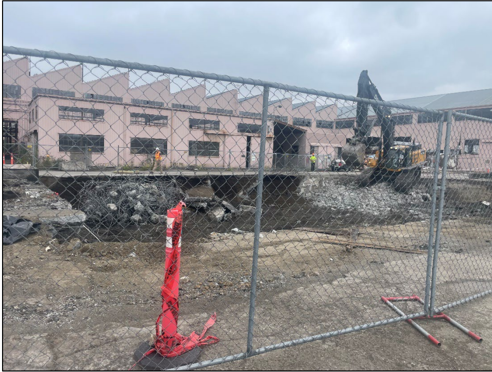
Figure 1. Overview of North Tank (NT) at Start of Day (SOD), 8/29/23 Facing West
