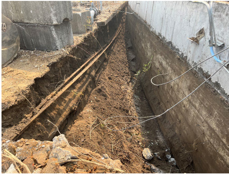
Figure 5. Eastern wall of the South Vault after removing the concrete wall.
