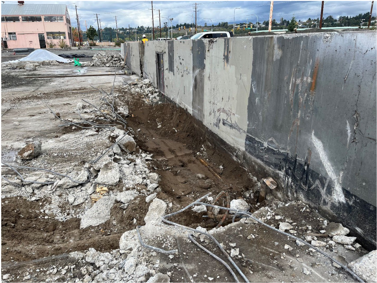
Figure 6. Eastern wall of Aluminum building excavation during pipe routing work.
