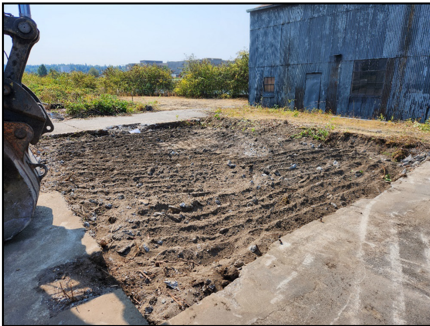
Photo CAA-03: Facing Southwest, Photo of the CAA sub-slab soil Date Taken: 8/24/2023
