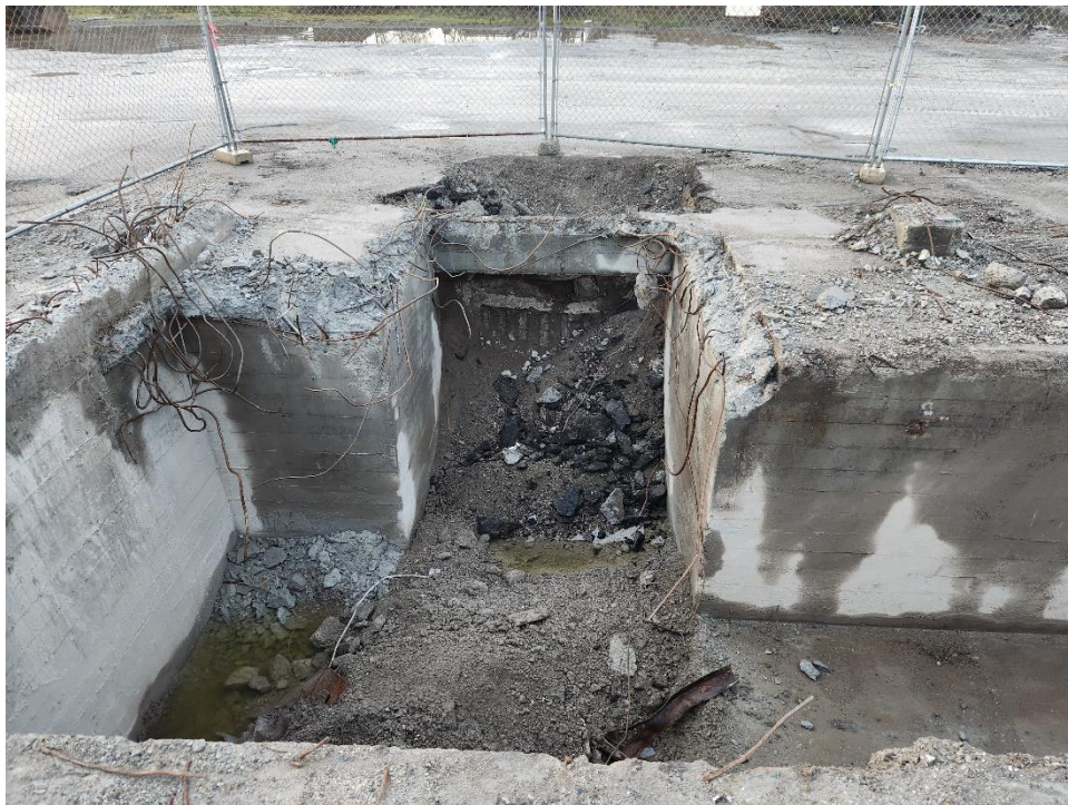
Photo 6: Powerhouse vault, west of the Powerhouse, following soil removal from the portion of the vault extending east-west. The vault appears to end after the steel I-beam visible in the top portion of this picture, and the fill material distinctly changes to a very dense gravel. No concrete sidewall was present at the south end of the vault. View to the south.
