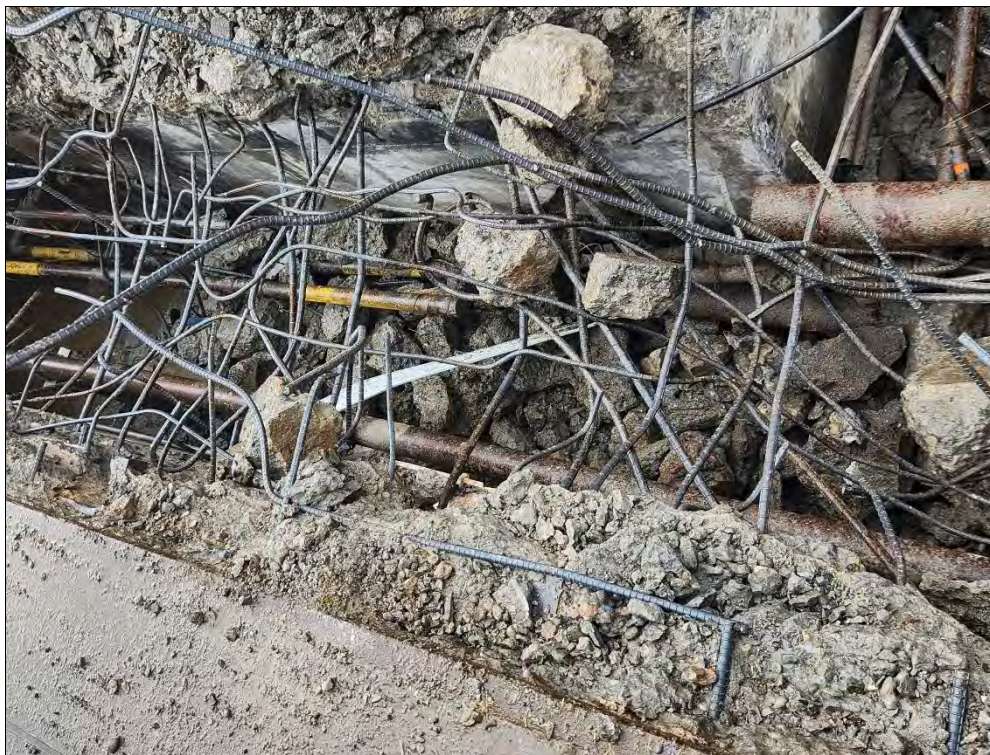
Photo 22: South Tank Vault, product piping in the utilidor following removal of the concrete top. Note there are more pipes visible in the utilidor than were visible running towards the former tanks. Several of the pipes had been cut and/or capped at some point in the past. View to the south southwest.
