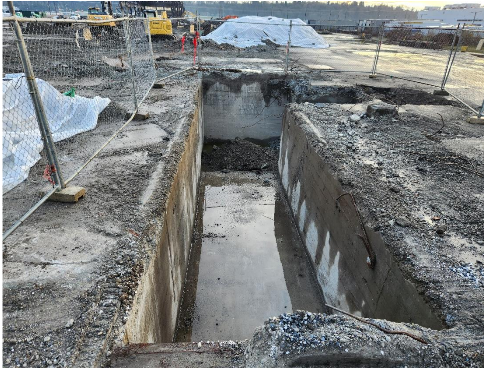
Photo 5: Powerhouse vault, west of the Powerhouse, following soil removal from the portion of the vault extending east-west. View to the east.
