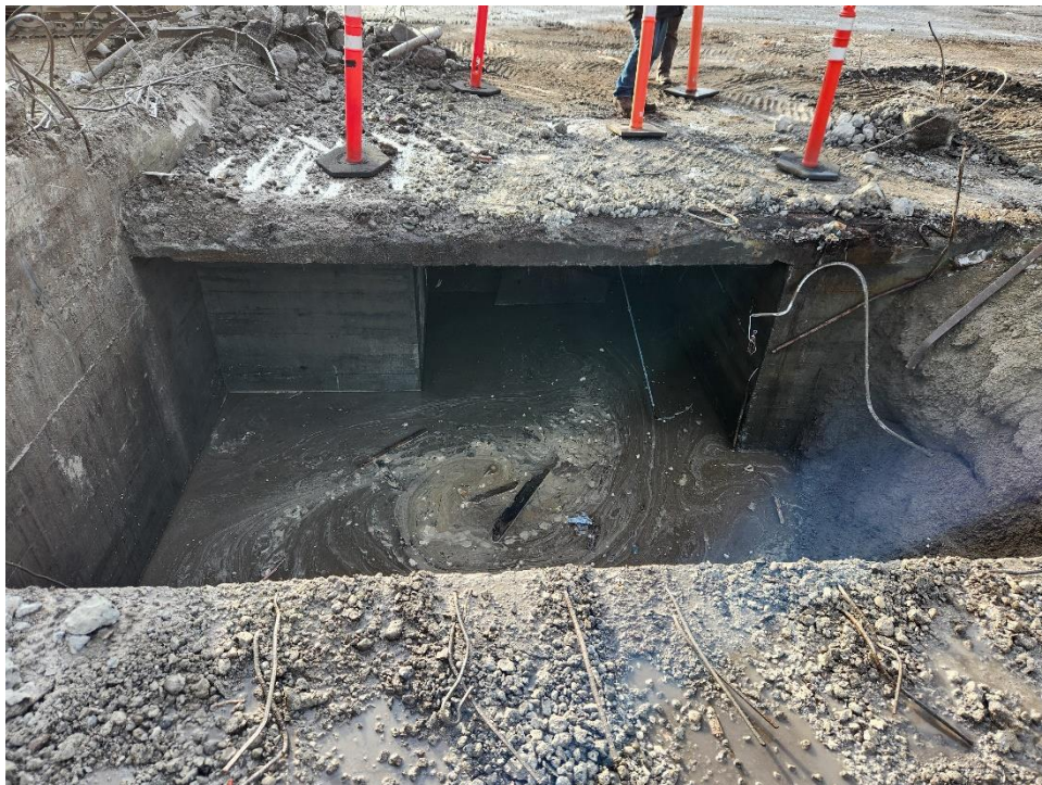
Photo 2: Powerhouse vault, west of the Powerhouse, after initial discovery. View to the south.
