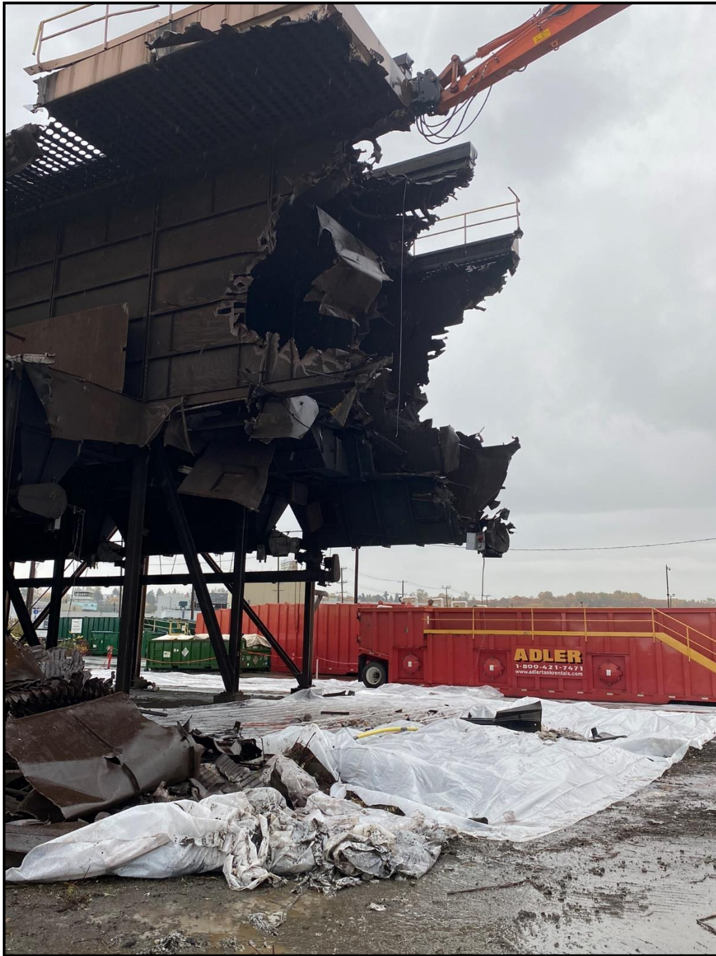
Photo BH-07: Facing East, Active Demolition of Baghouse Structure Photo Taken: 11/10/2023
