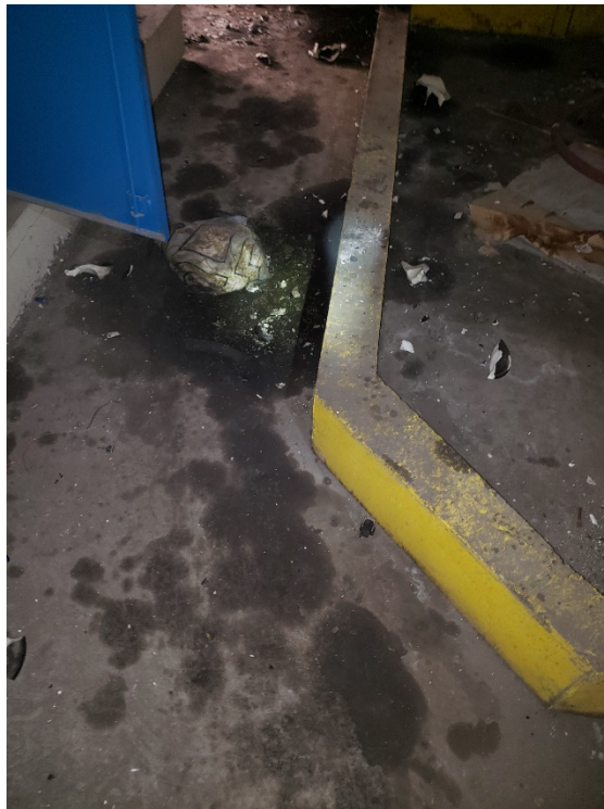
Photo 5: First level spill area prior to cleanup actions.
