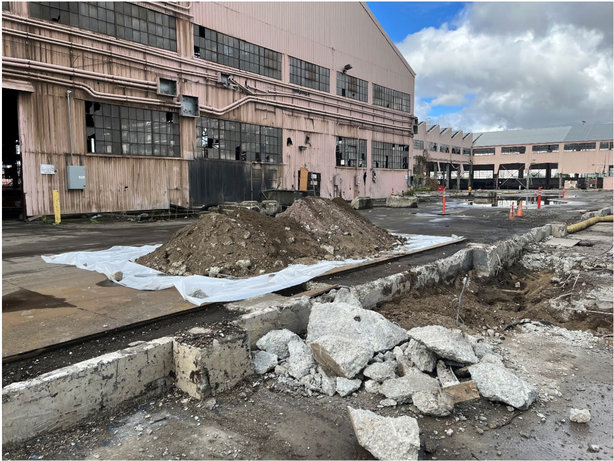
Figure 5. Western wall of Aluminum building foundation with soil pile.
