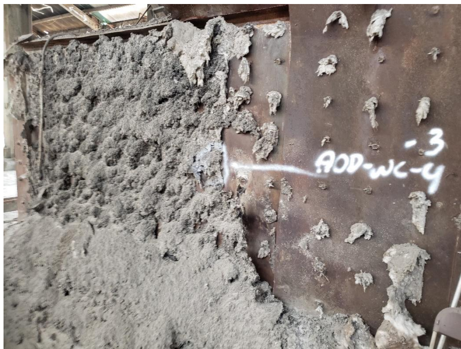
Photo 3: Sample AOD-WC-3 and -4, along the south wall of the AOD Pit. View to the S.
