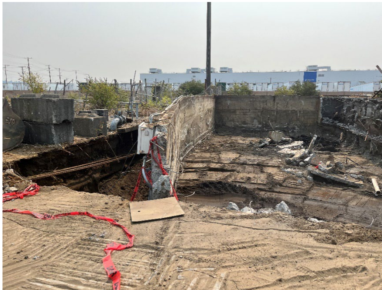
Figure 6. Overview end of day, view South Vault.
