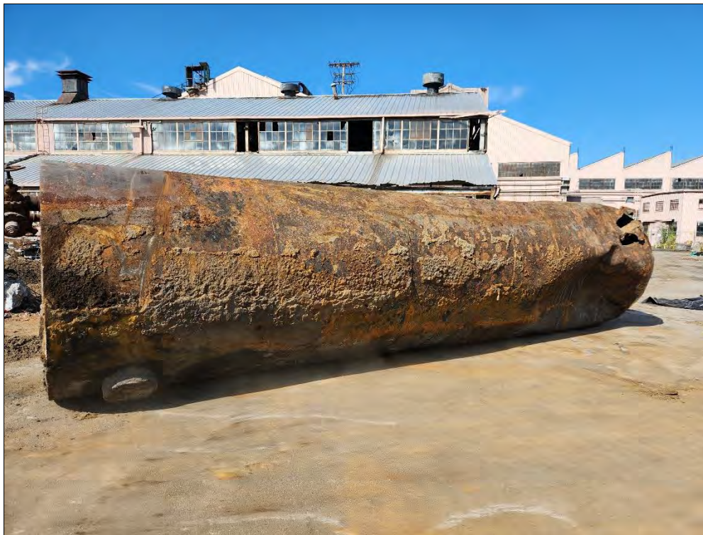
Photo 14: South Tank Vault, tank staged for transport. Note the condition of the tanks from the South Tank Vault in comparison to those from the North Tank Vault. View to the west.
