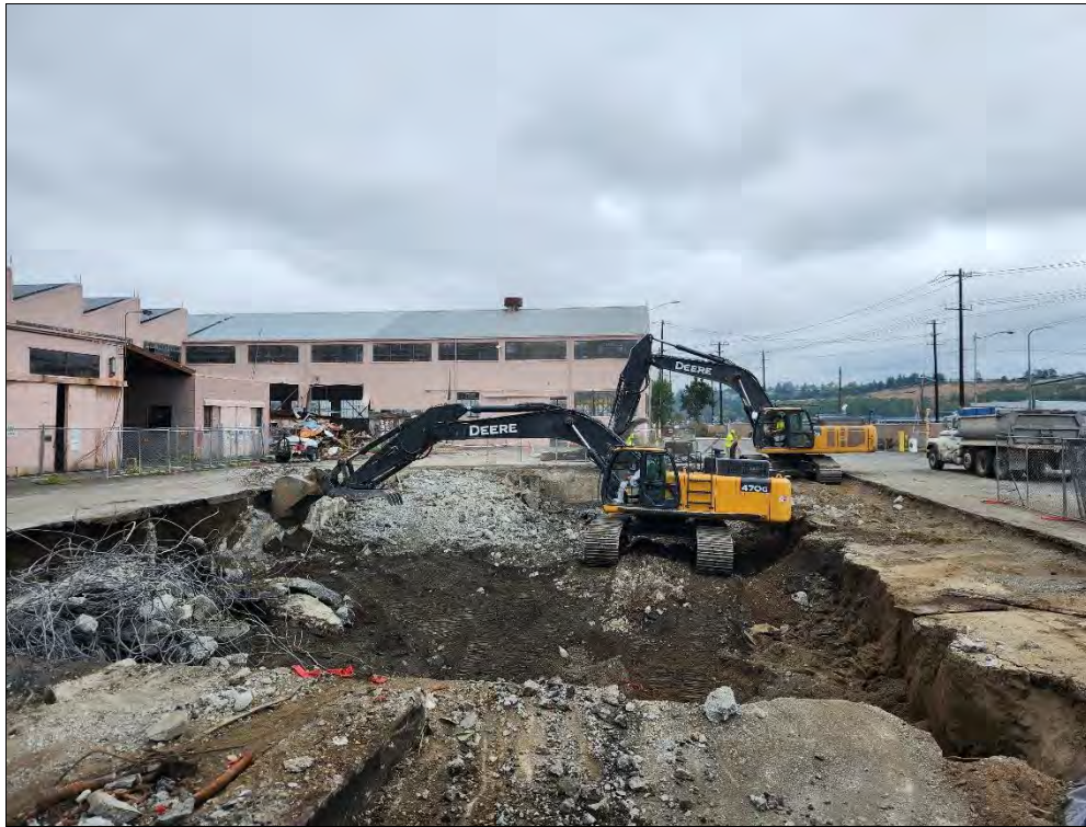
Photo 9: North Tank Vault, removal of the concrete vault structure. View to the north.
