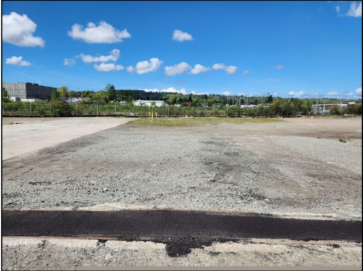
Photo TSA-04: Facing Waste, Backfilled Footprint of Tote Storage Area Date Taken: 4/22/2024
