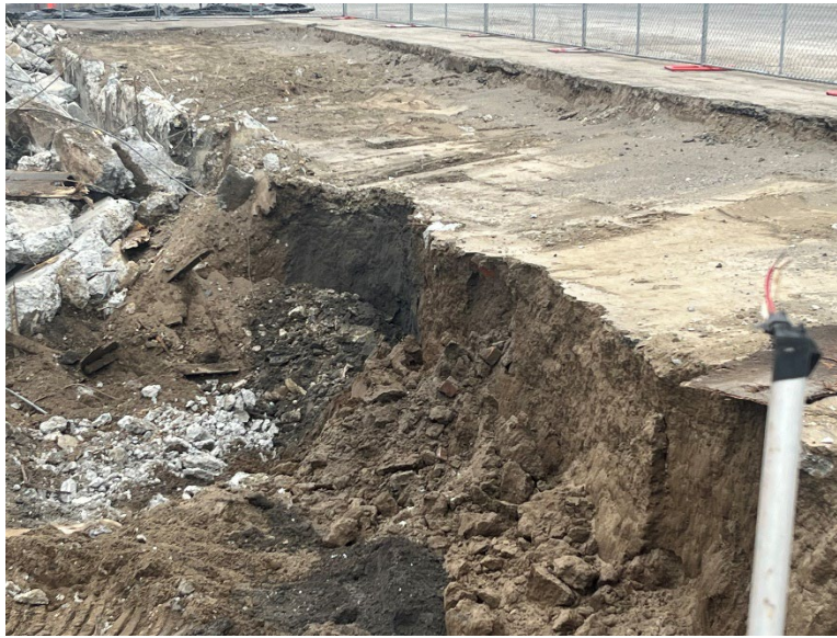
Figure 3. Eastern wall of the North Vault.
