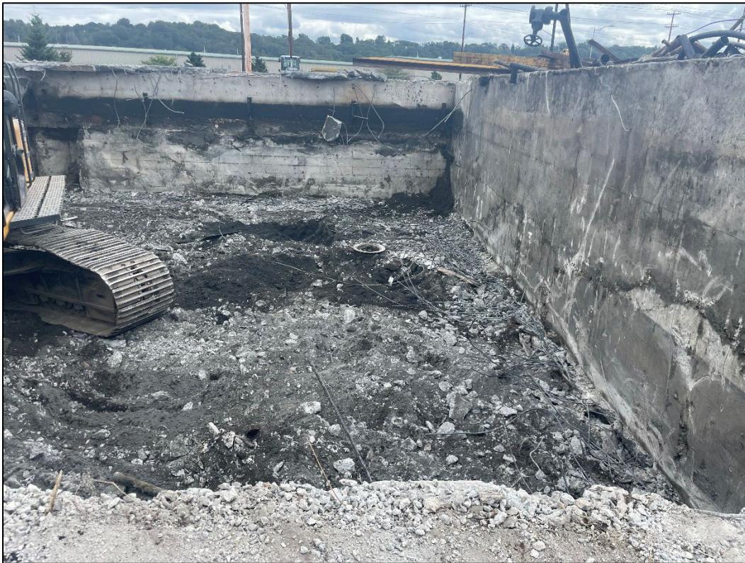
Figure 10: NT-SS-9 Overview, facing E
