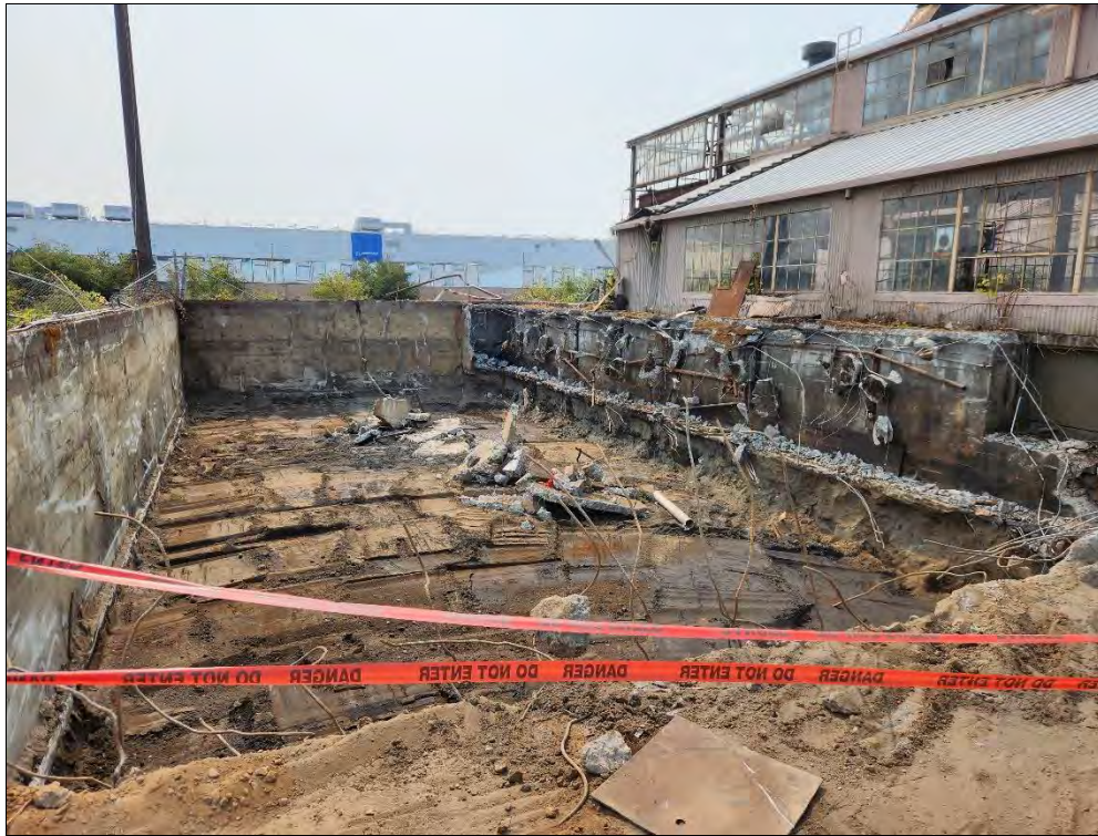
Photo 17: South Tank Vault, emptied of tanks and backfill, prior to removal of the concrete vault. View to the south southwest.
