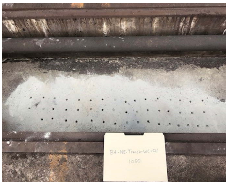
Photo 10: Sample location BH-NE-Trench-WC-01.
