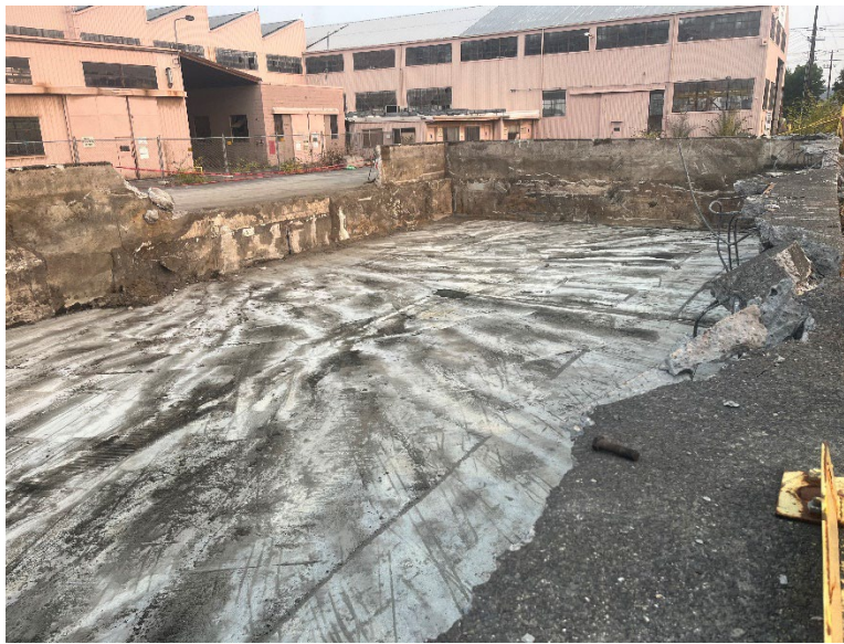
Figure 1. Overview start of day, view North Vault.
