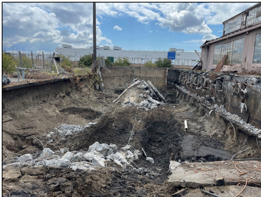
Figure 5-6. North and South UST Systems, facing northwest
