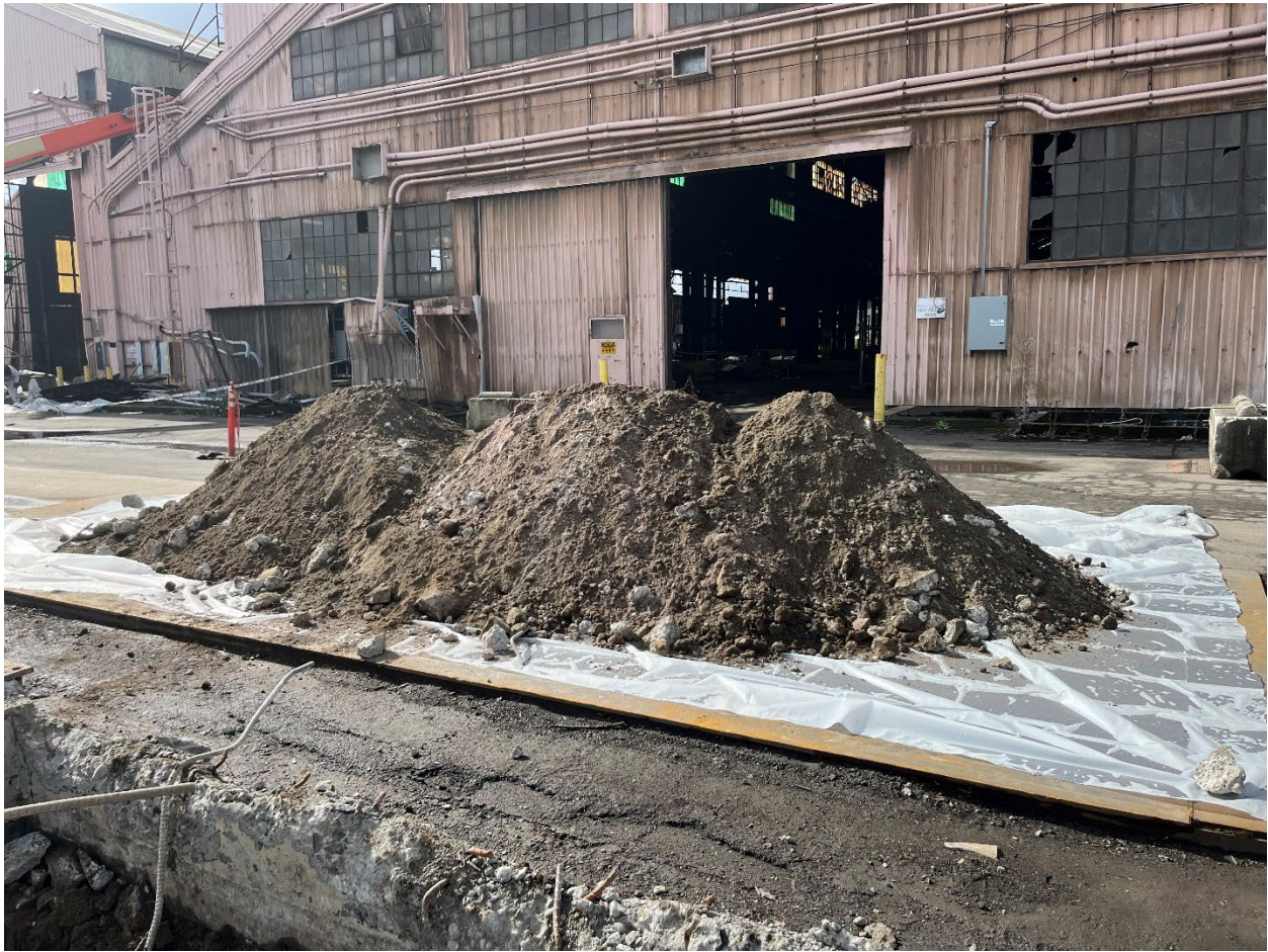
Figure 7. Soil removed during excavation and sampling.
