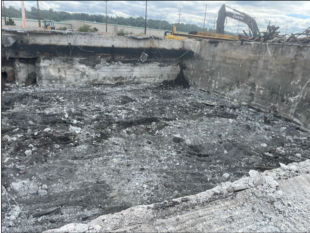
Figure 5: Overview at start of soil sampling showing cleared section, facing E
