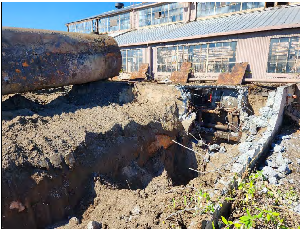
Photo 12: South Tank Vault, removal of UST-15. View to the southwest.
