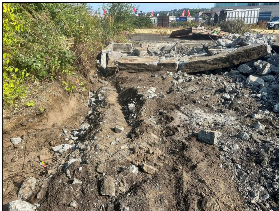
Figure 5-9. Overview Central Accumulation Area/Oil Shed, facing south
