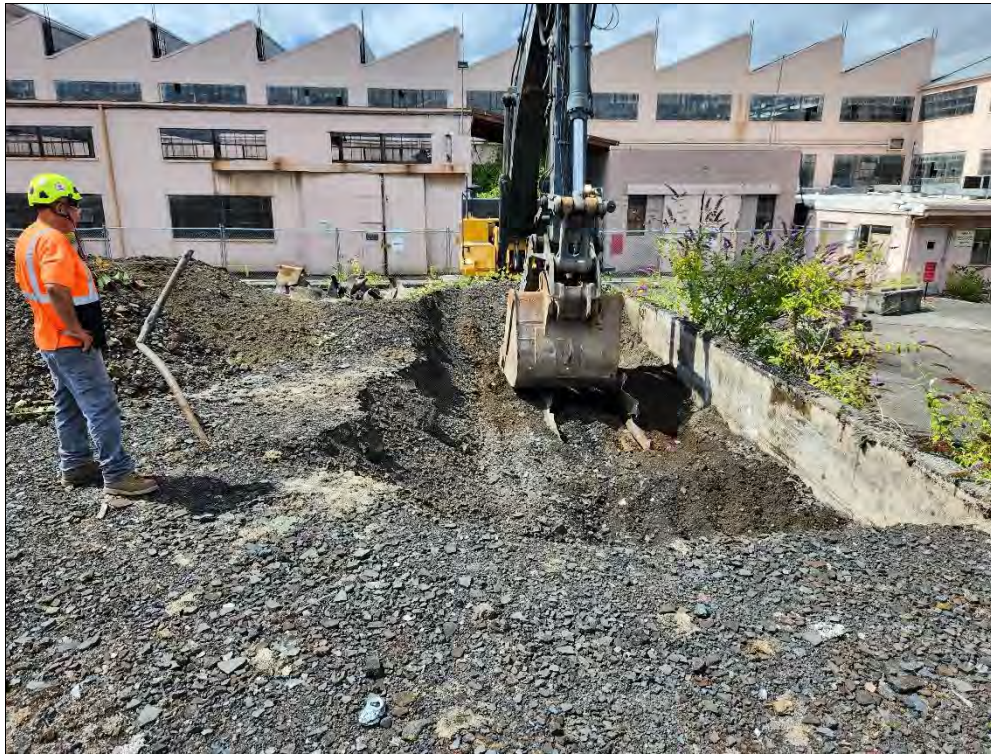
Photo 1: North Tank Vault, exposing UST-26 in preparation for removal. View to the west.
