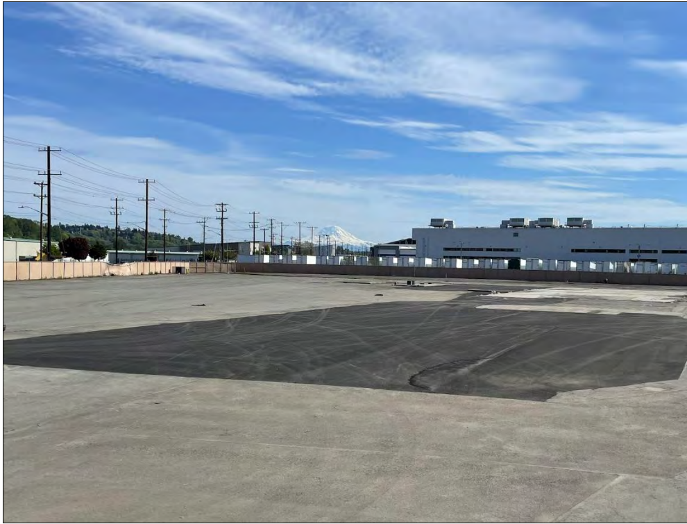
Photo 11: North Tank Vault, following final paving and site restoration. View to the south southwest.
