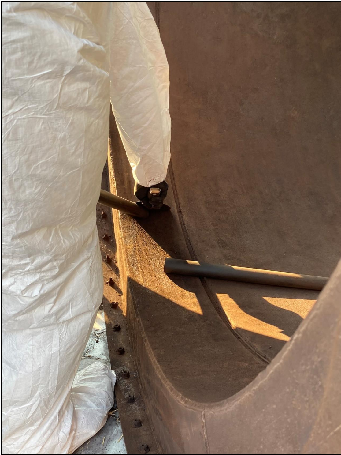
Photo BH-05: Active Scraping and Vacuum Removal of Baghouse Dust in the Duct Interior Photo Taken: 9/22/2023
