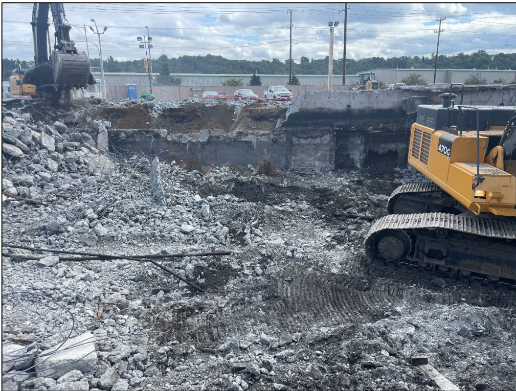
Figure 20: UST-29 Overview, facing NE
