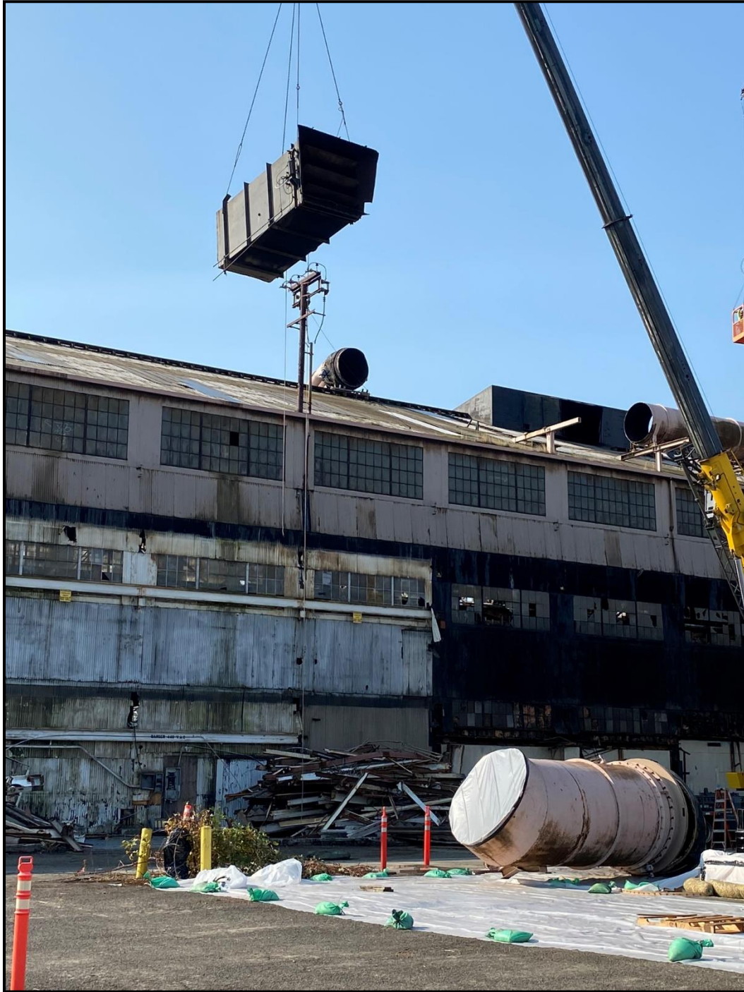
Photo BH-03: Facing Southwest, Active Removal and Lowering of the Baghouse Tunnel Photo Taken: 9/22/2023
