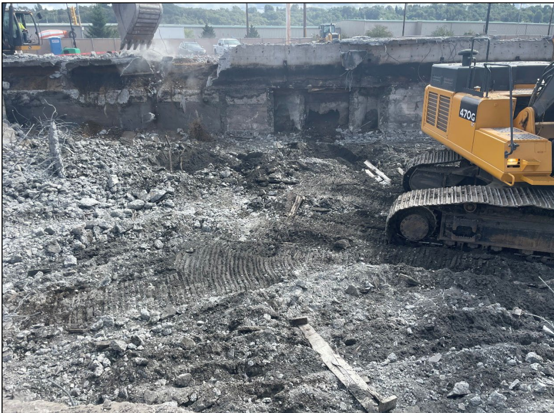
Figure 16: UST-31 Overview, facing NE
