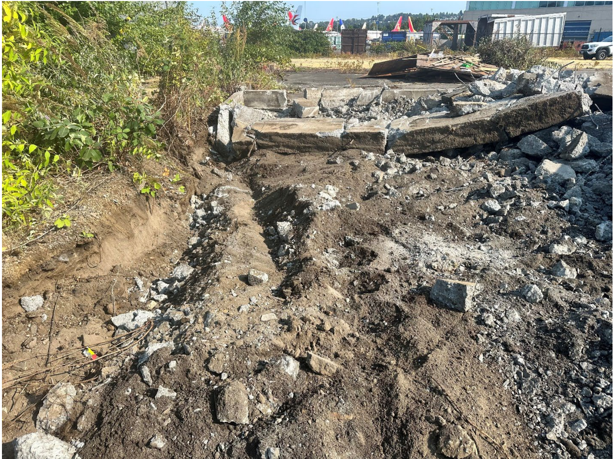
Figure 1. Overview start of day, view north.
