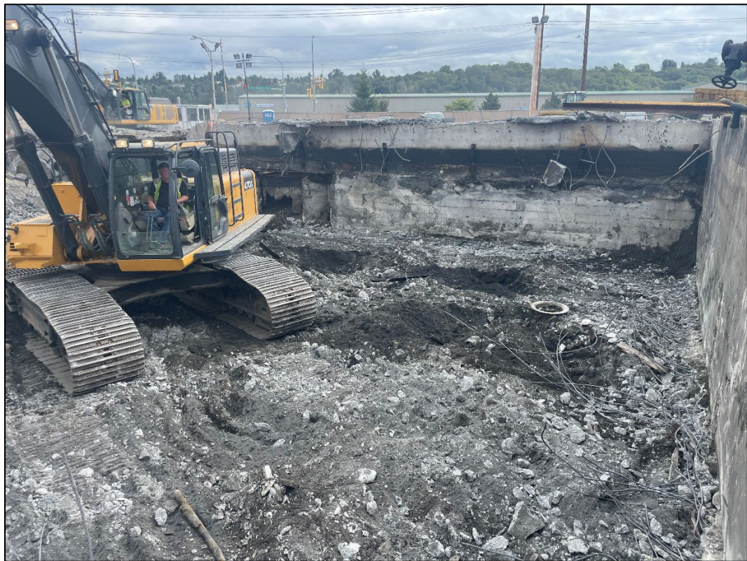
Figure 12: NT-SS-8 Overview, facing E
