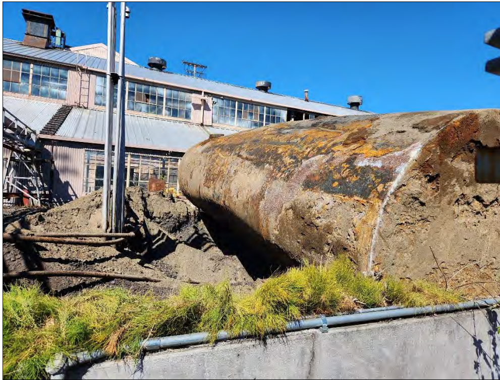
Photo 13: South Tank Vault, tank prepared for removal. View to the west.
