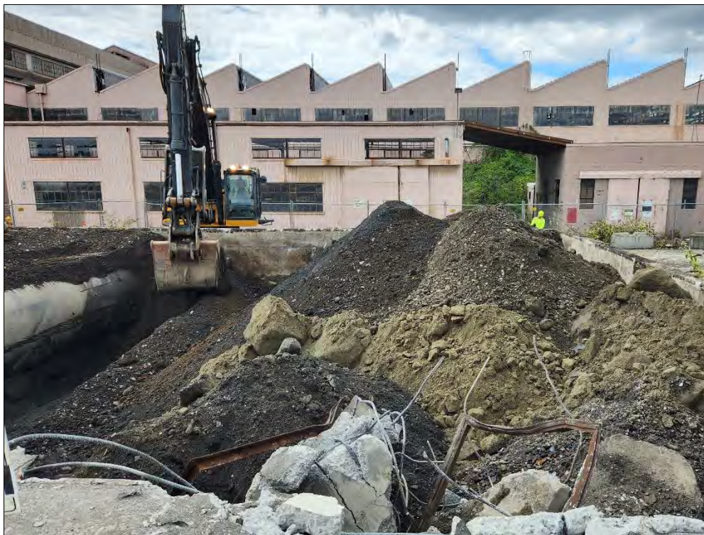
Photo 2: North Tank Vault, exposing UST-28 in preparation for removal. View to the west.
