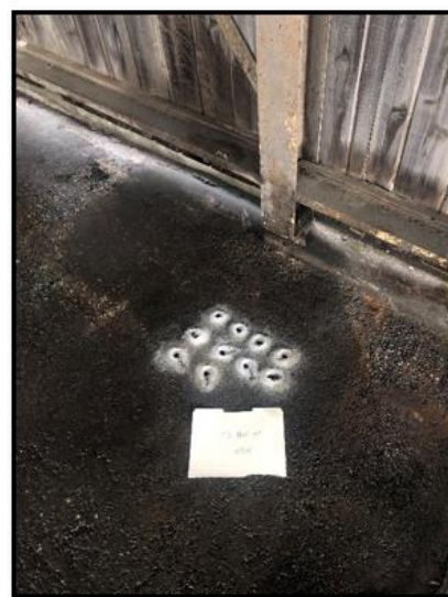
Photo 6: Tote Storage Area NW Quadrant, 03 June 2020
