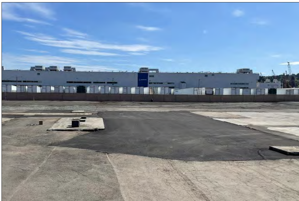
Photo 24: South Tank Vault, following final paving and site restoration. View to the south.
