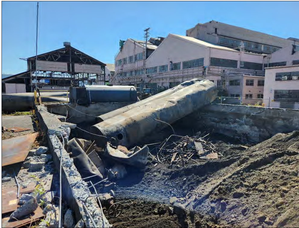
Photo 3: North Tank Vault, last two tanks prepared for removal. View to the south southwest.
