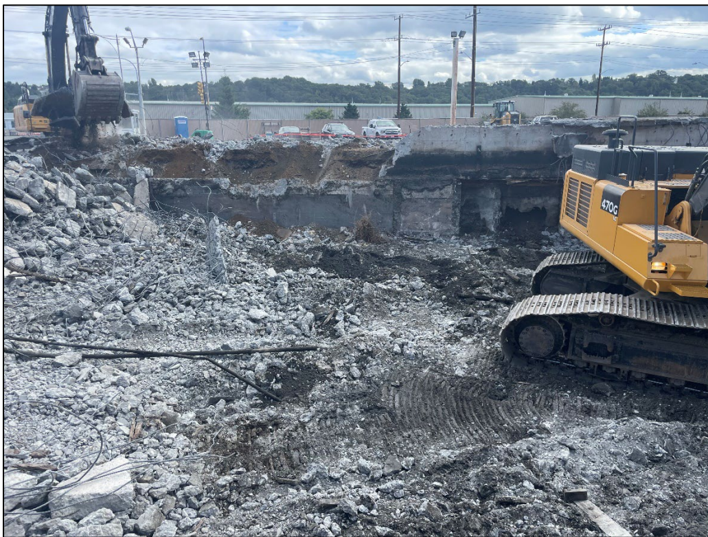
Figure 18: UST-30 Overview, facing NE
