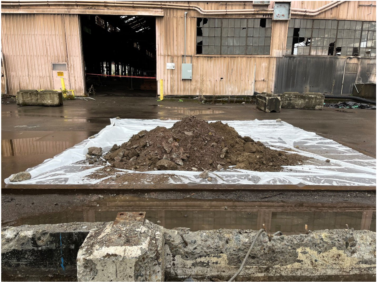
Figure 4. Western wall of the Aluminum building foundation.
