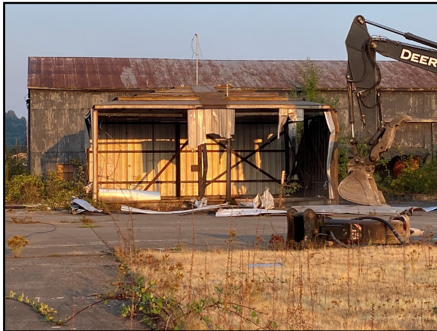
Photo CAA-01: Facing West, Pre-Demolition Photo of the CAA (forefront building) Date Taken: 8/24/2023
