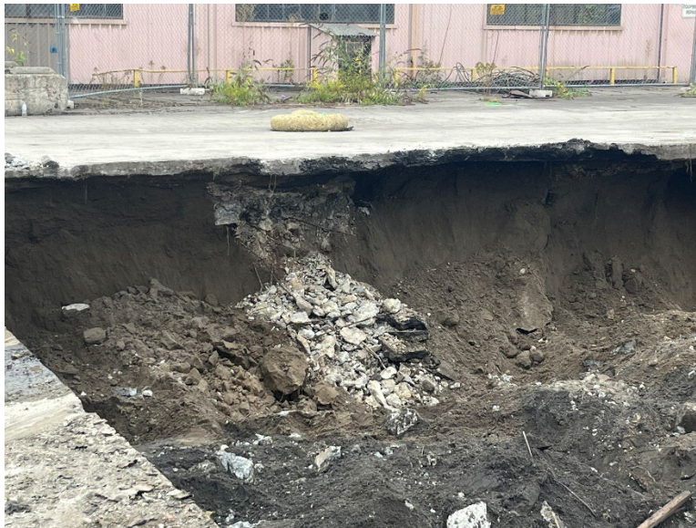
Figure 4. Western wall of the North Vault.
