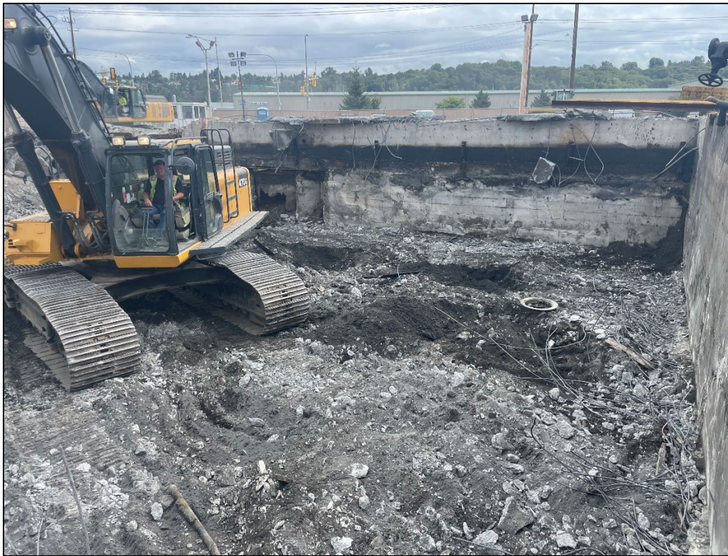
Figure 8: NT-SS-10 Overview, facing E
