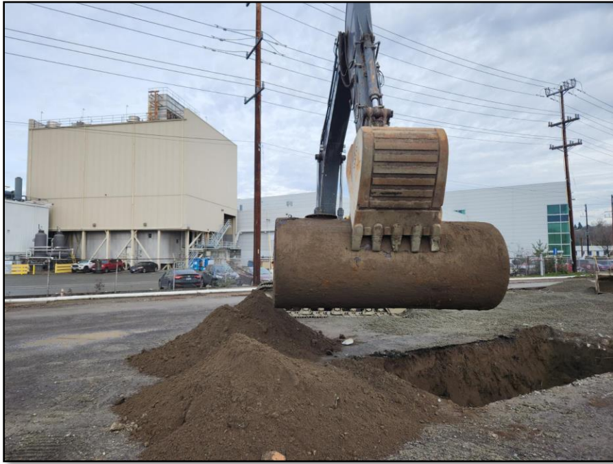
Photo 03, Facing Northwest, Admin Building Heating Oil Tank Excavation, 1/29/2024
