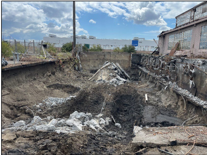
Figure 15. South Tank (ST) Overview, facing South
