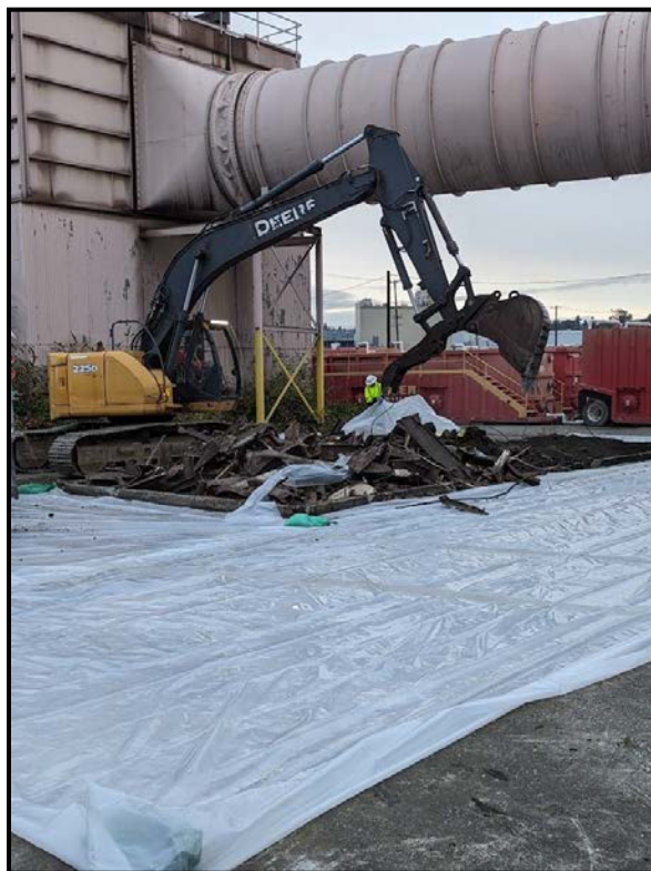
Photo TSA-02: Facing Northeast, Active Demolition of the Tote Storage Area Date Taken: 10/24/2023
