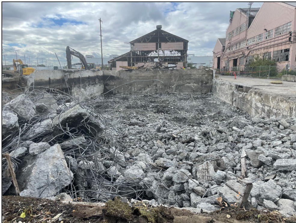
Figure 4: Overview of North UST System at start of soil sampling, with part of concrete foundation removed, facing S
