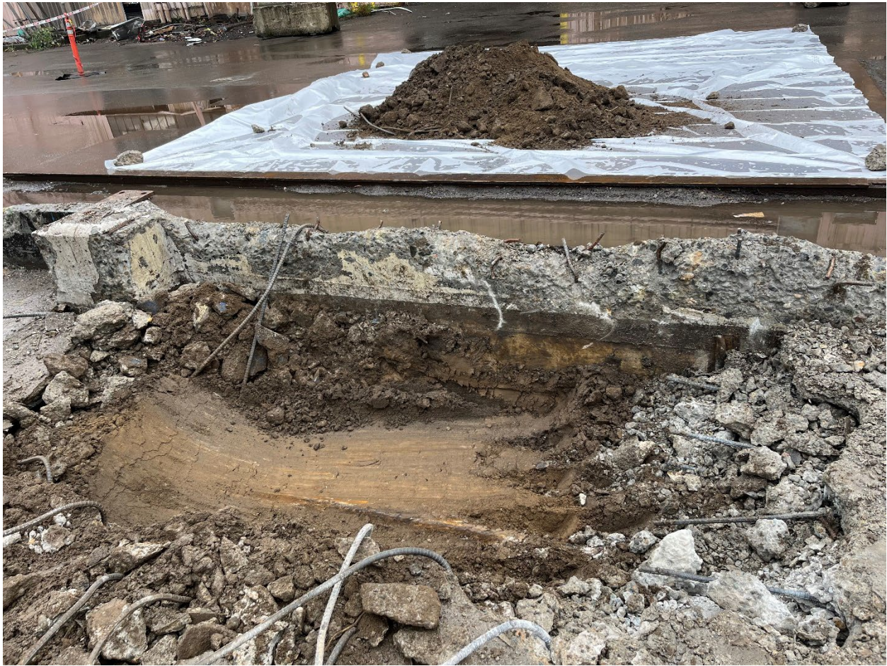
Figure 3. Start of the western wall of the Aluminum building foundation excavation.
