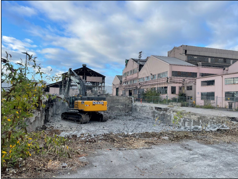
Figure 3: Overview at start of day, construction crew removing concrete foundation from North UST System; facing S
