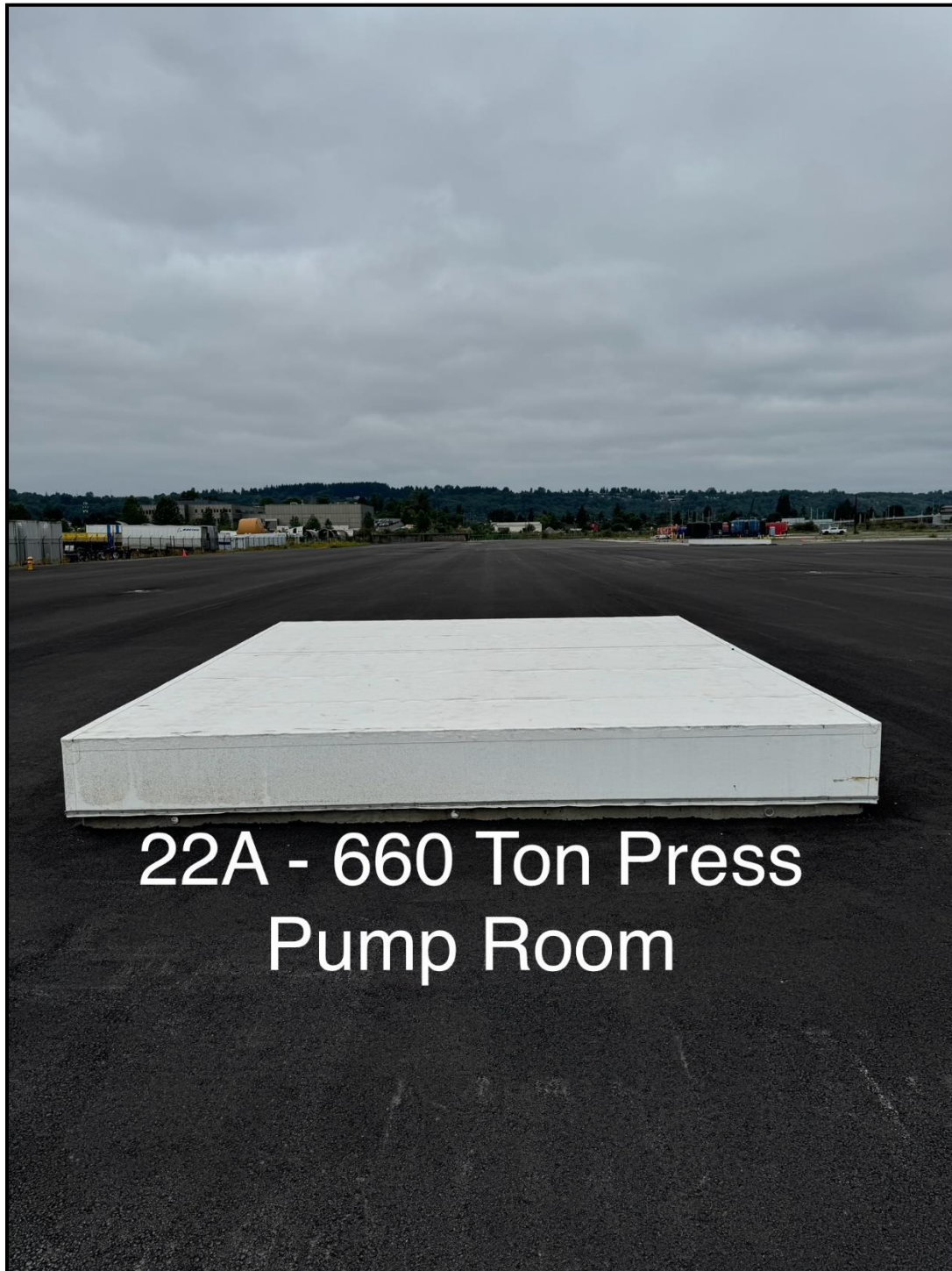
Photo 09, Facing West, 660 Ton Press Pump Room Pit Cover
