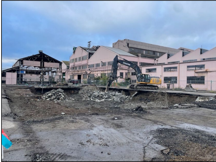
Figure 3. NT Overview at SOD, 8/30/23, Facing West
