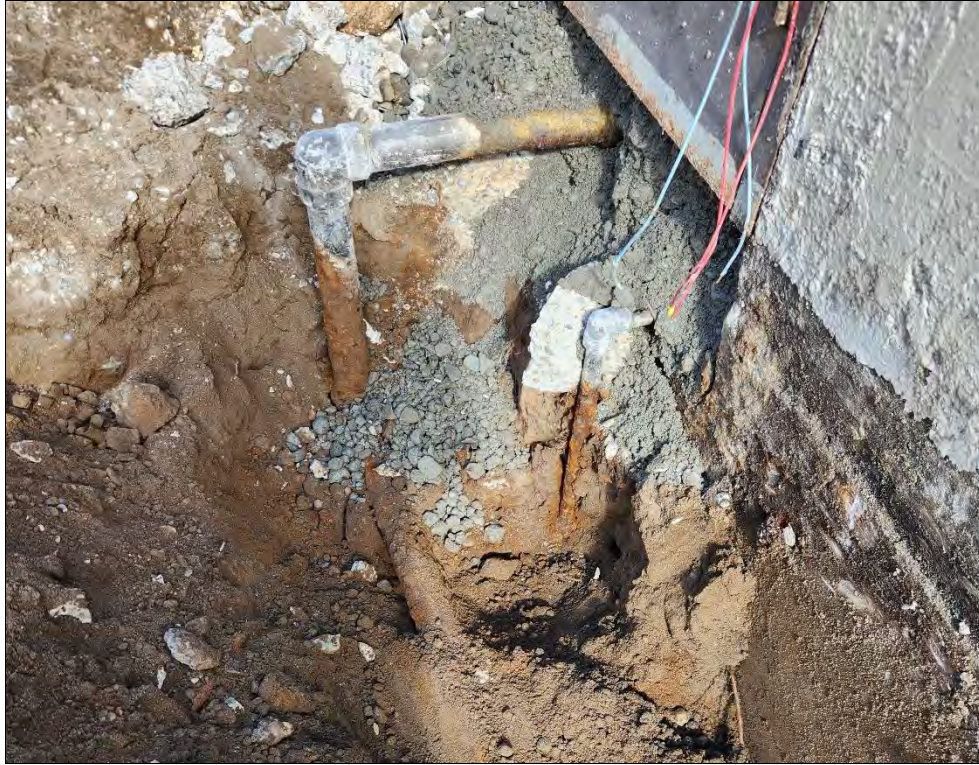
Photo 19: South Tank Vault, single product line visible entering the foundation underneath of the former Aluminum Building, along with a small electrical conduit. View to the north northeast.
