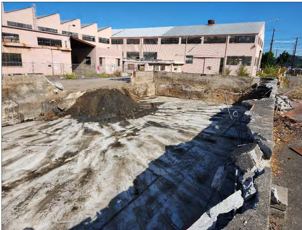
Photo 6: North Tank Vault, emptied of tanks and backfill, prior to removal of the concrete vault. View to the northwest.
