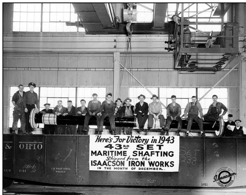
Figure 2-12. Workers at Issacson Iron Works in 1943 (University of Washington Libraries 2022 Digital Collections, IND0085)
