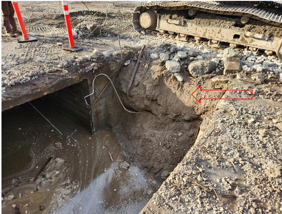
Photo 3: Powerhouse vault, west of the Powerhouse, after initial discovery. Initial waste characterization soil sample collected from the brown soil marked with a red arrow. View to the southwest.
