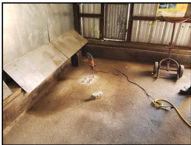
Photo 2: CAA Containment, SE Quadrant, 29 May 2020
