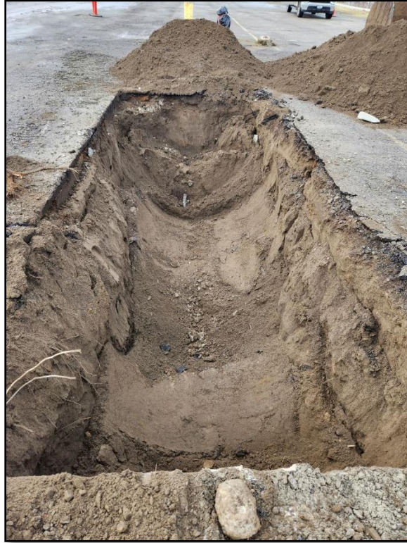
Photo 01, Facing West, Admin Building Heating Oil Tank Excavation, 1/29/2024
