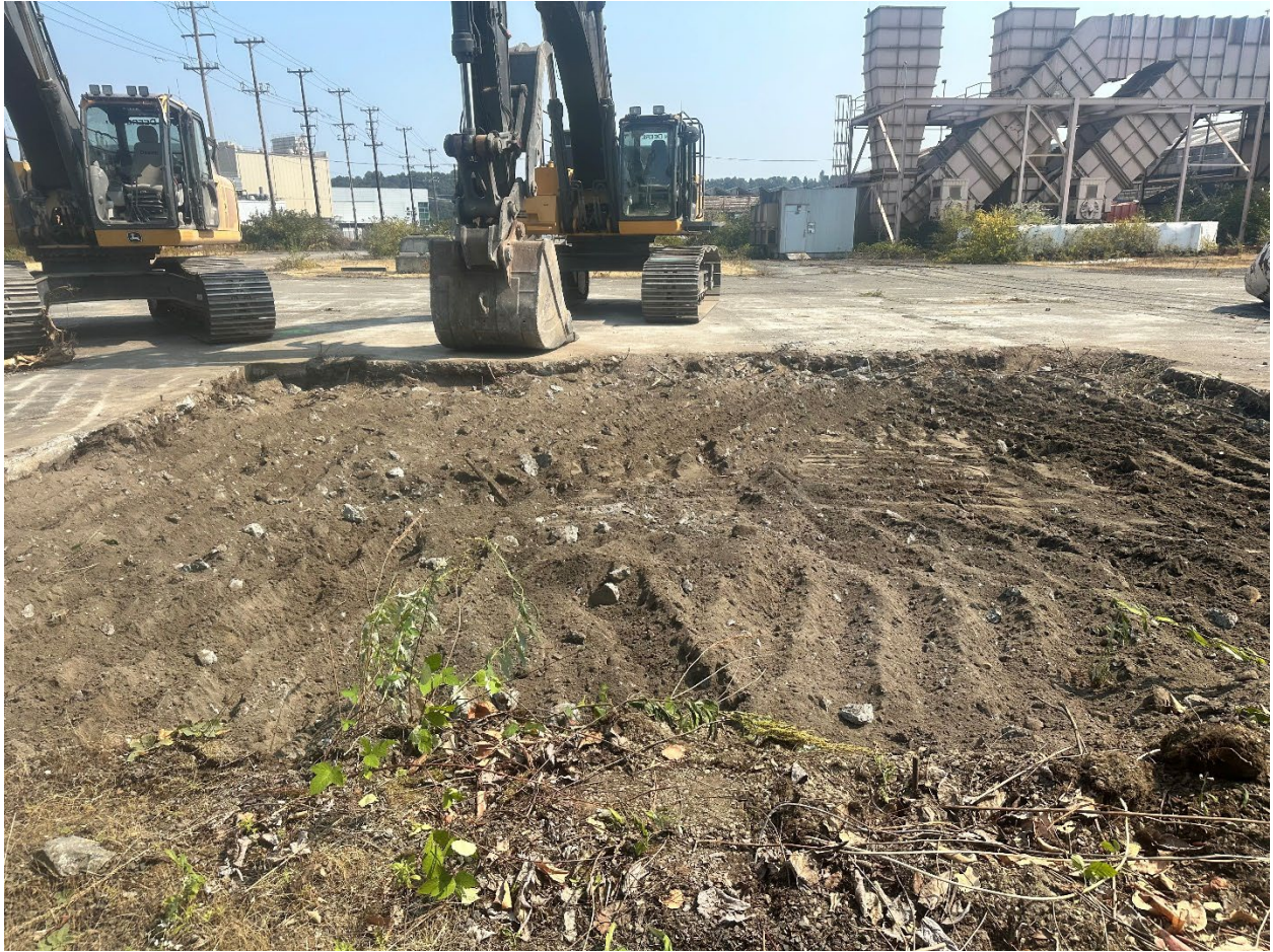
Figure 6. Overview end of day, view east.
