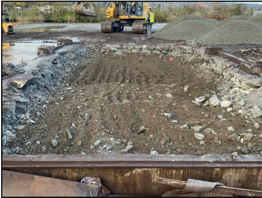
Photo BH-08: Facing North, Footprint of Baghouse North After Slab Removal Photo Taken: 11/22/2023
