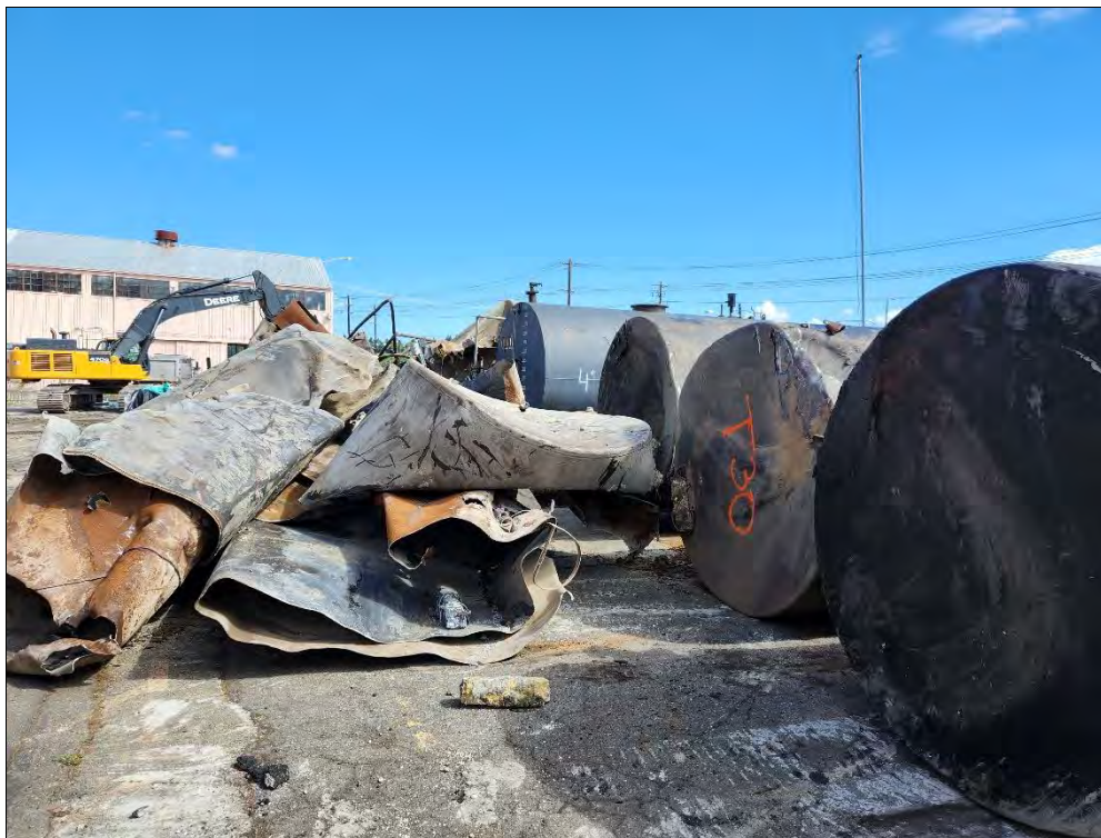
Photo 4: North Tank Vault, tanks staged for transport. The tank fragments on the left side were tanks previously filled with sand, which were cut open to empty. View to the north.
