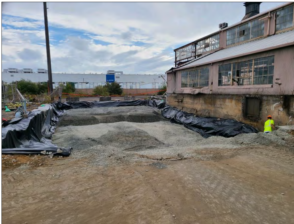
Photo 18: South Tank Vault, backfilling the excavation. View to the south southwest.
