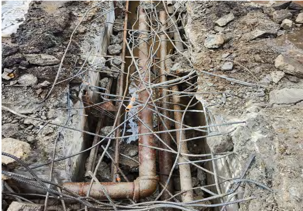
Photo 23: South Tank Vault, product piping in the utilidor following removal of the concrete top. Note there are more pipes visible in the utilidor than were visible running towards the former tanks. Several of the pipes had been cut and/or capped at some point in the past. View to the south southwest.
