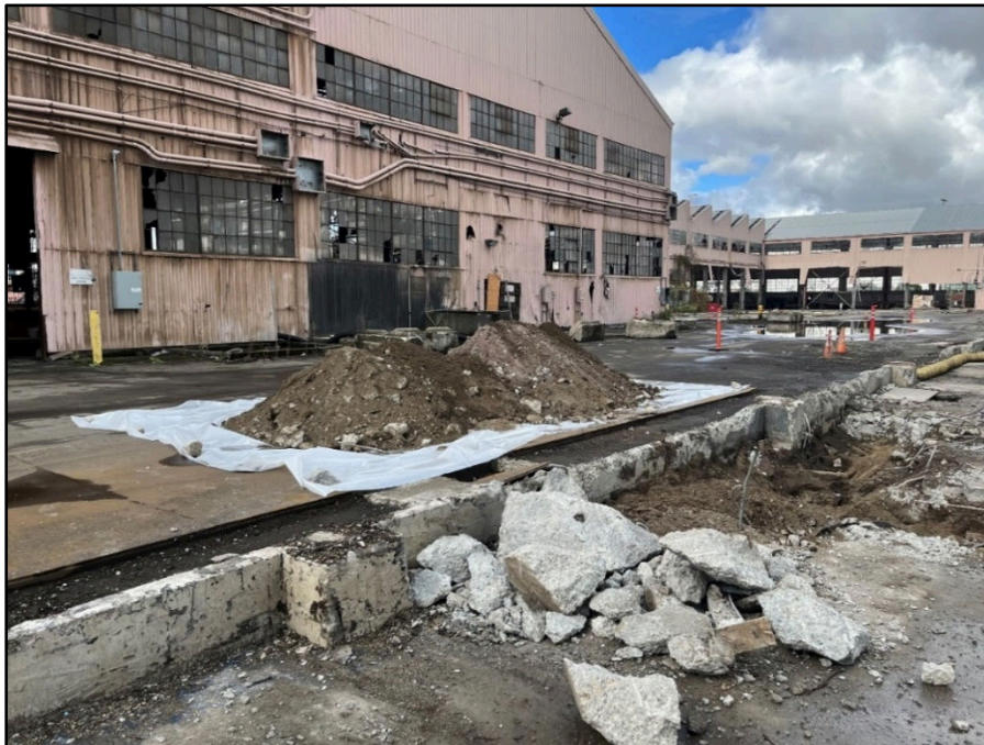
Figure 5-1. Western wall of Aluminum building foundation with soil pile, facing northwest
