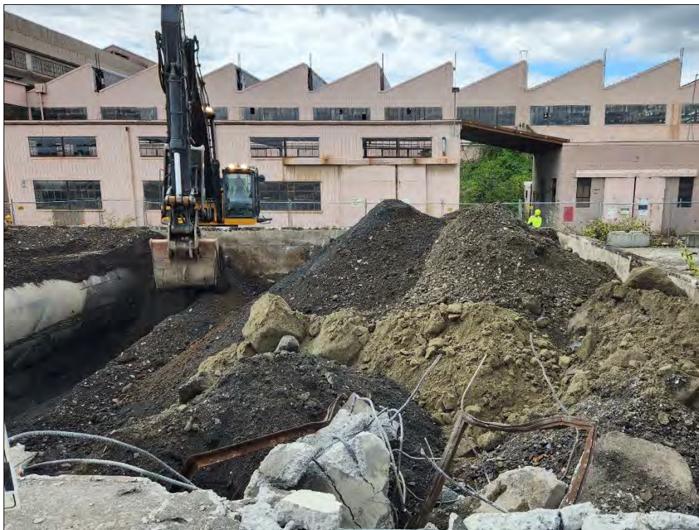
Photo 2: North Tank Vault, exposing UST-28 in preparation for removal. View to the west.
