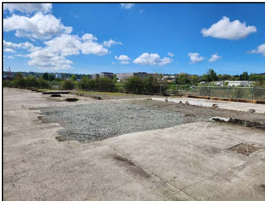
Photo CAA-04: Facing Southwest, Photo of the CAA, backfilled and closure completed Date Taken: 4/23/2024
