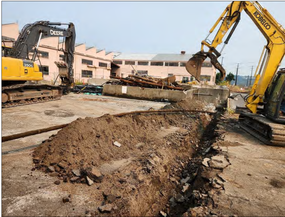
Photo 7: North Tank Vault, product piping removal. View to the north northwest.
