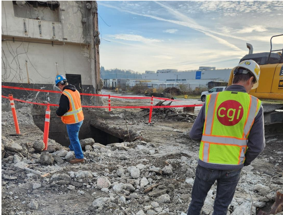
Photo 1: Location of the vault, west of the Powerhouse, after initial discovery. The vault was hidden beneath a concrete structure, and beneath a steel plate supported by an I-beam. The main Powerhouse structure is visible in the background, view to the east southeast.
