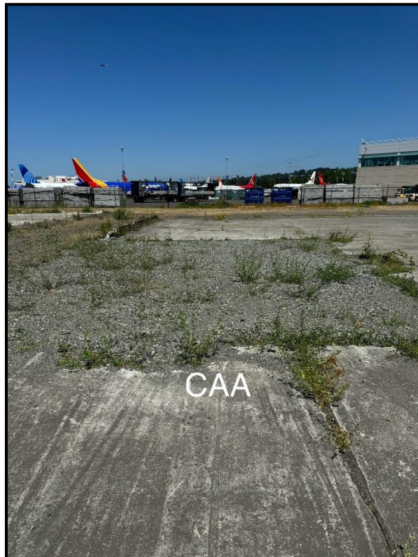
Photo 11, Facing North, Former Central Accumulation Area DWMU Area, 7/15/2024
