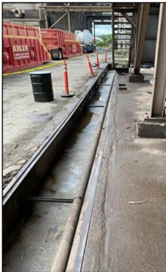
Photo 10: Baghouse Utility Trench, Facing South, 16 June 2020
