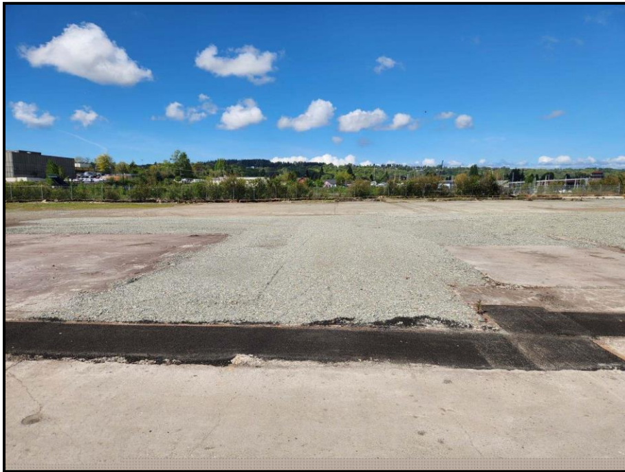
Photo BH-09: Facing West, Backfilled Footprint of Baghouse North Post Demolition Photo Taken: 4/22/2024
