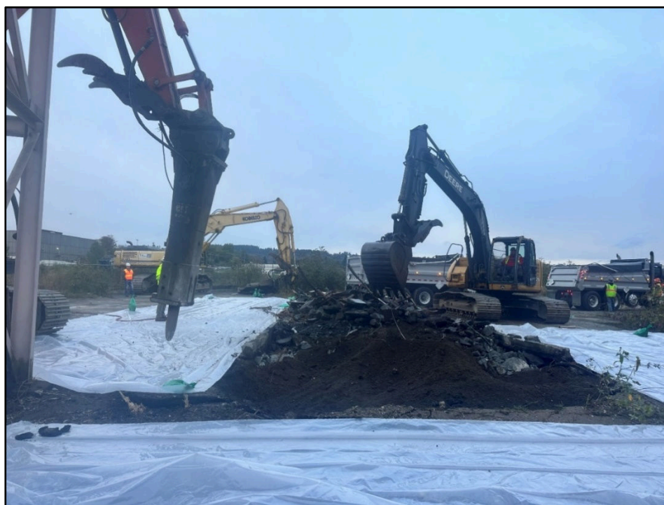
Figure 5-8. Overview Tote Storage Area, facing west
