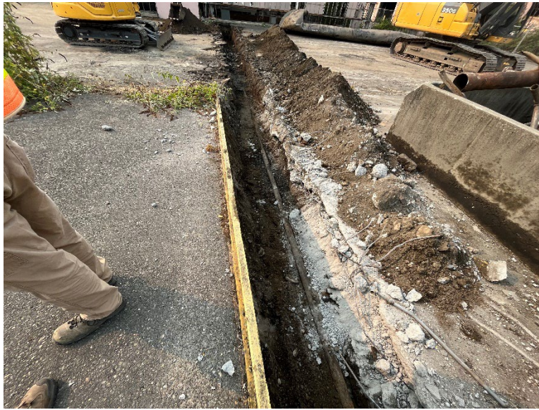
Figure 3. Unidentified piping running out of North Vault; prompted exploratory excavation.
