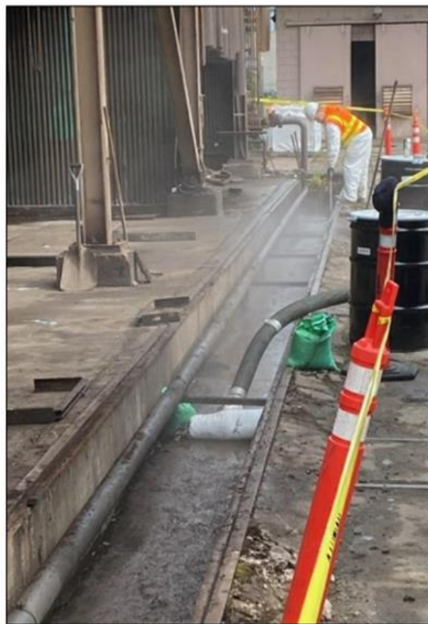
Photo 9: Baghouse Utility Trench, Facing North, 16 June 2020
