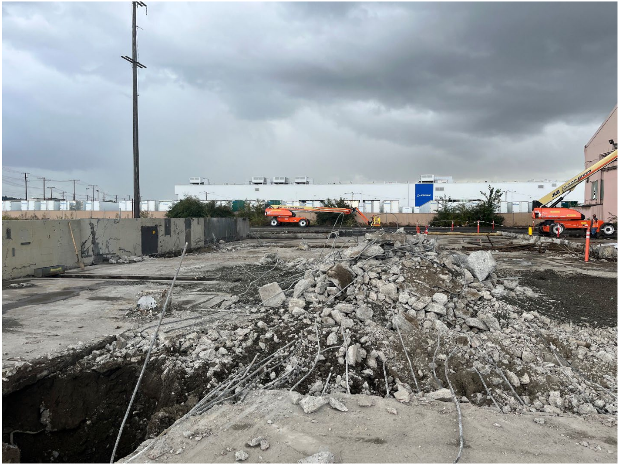
Figure 9. End of day overview.
