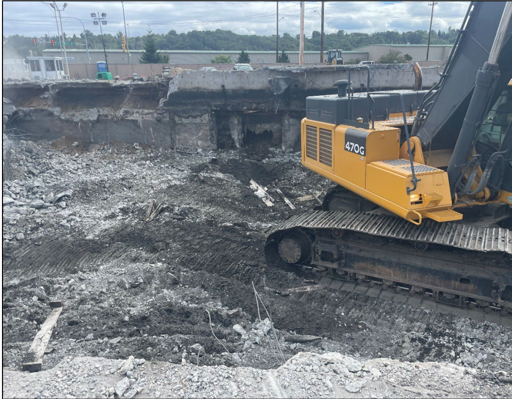
Figure 14: UST-32 Overview, facing NE
