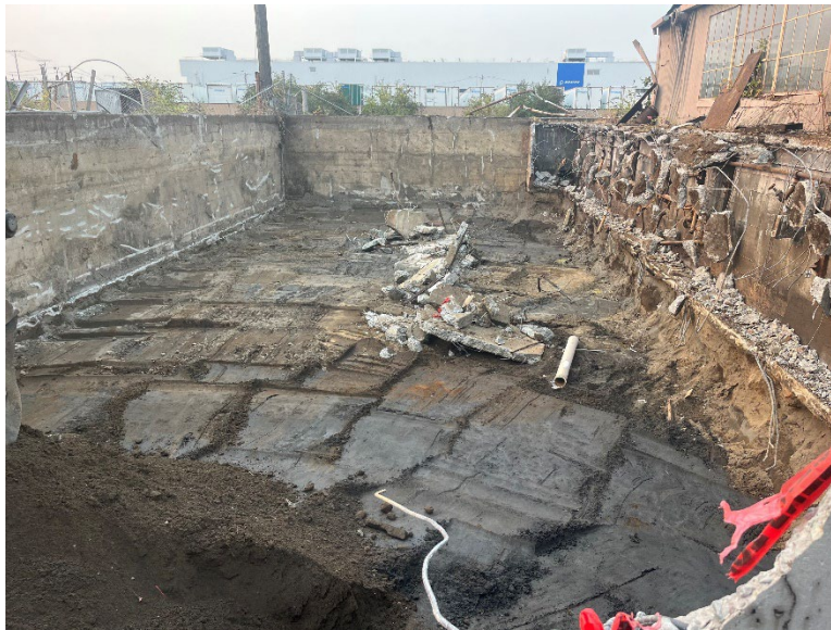
Figure 2. Overview start of day, view South Vault.
