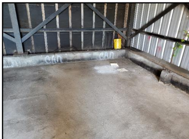
Photo 3: CAA Containment, NW Quadrant, 29 May 2020
