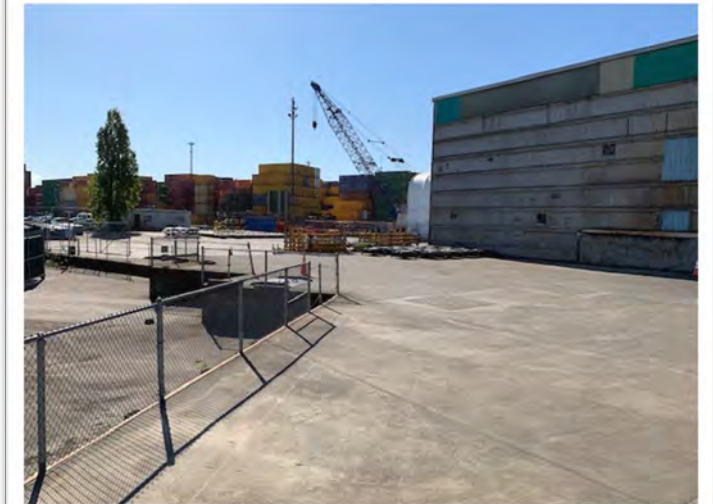
Photo 8: Former Unimacts Global, LLC Area Looking Southeast.
