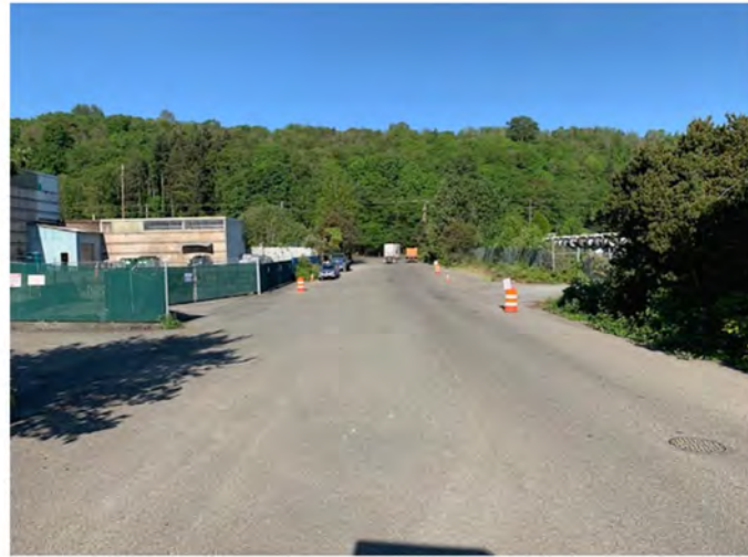
Photo 2: Terminal 115 Driveway Looking West.
