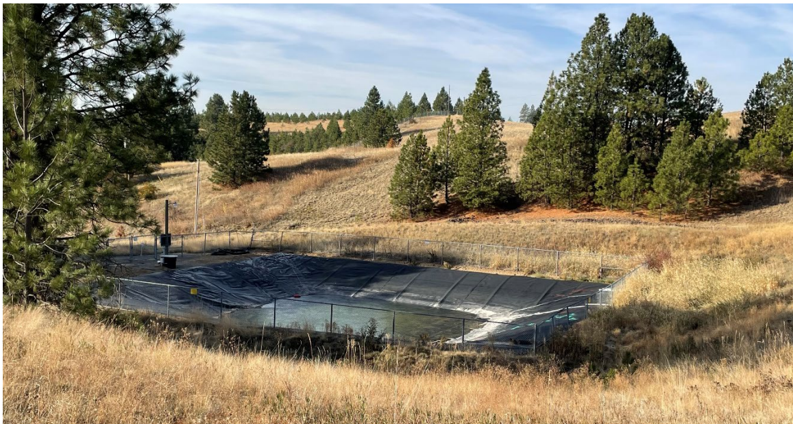
Photo 2: View of southeast leachate pond facing west
