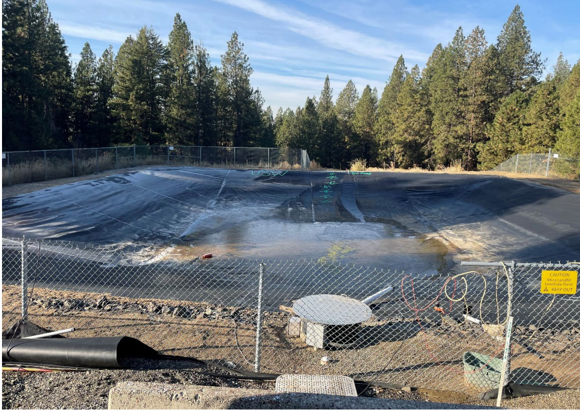
Photo 1: View of southwest leachate pond facing south
