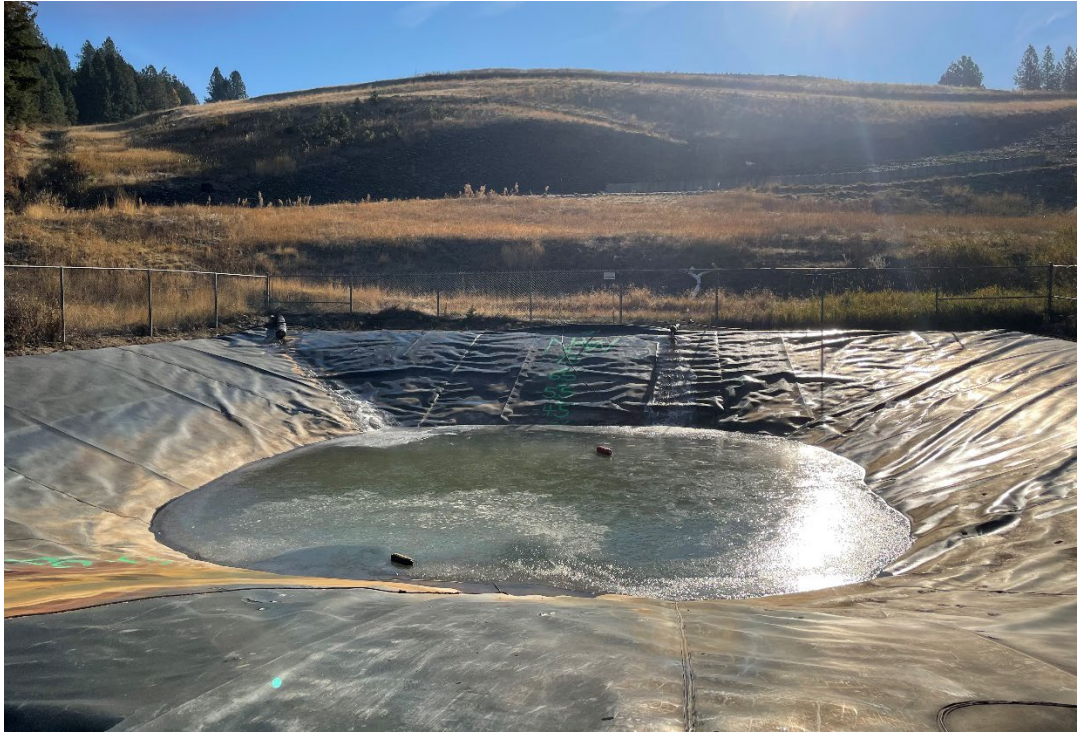
Photo 3: View of northwest leachate pond facing south
