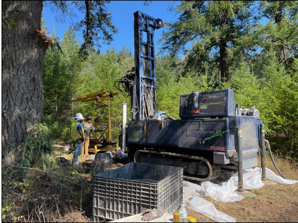
Photograph B-1. Sonic drilling and soil sampling activities at Building 1864 Former Fire Station location CBV-1864-07
