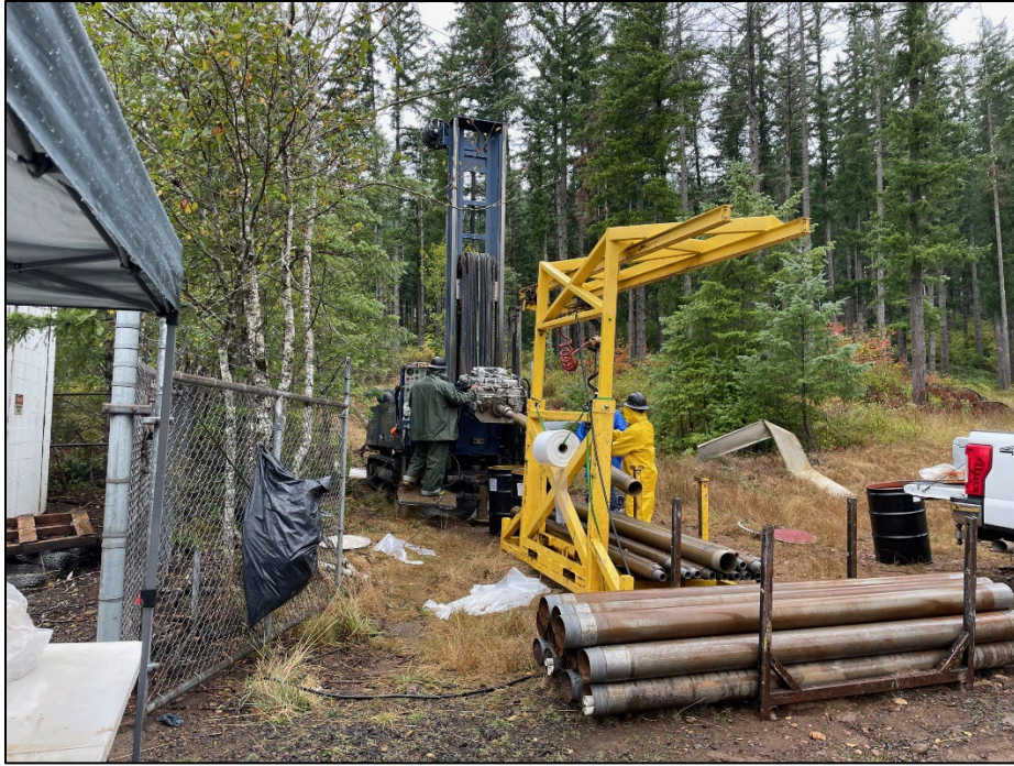
Photograph B-3. Sonic drilling and soil sampling activities at Wash Racks 1 and 2 location CBV-WR12-06
