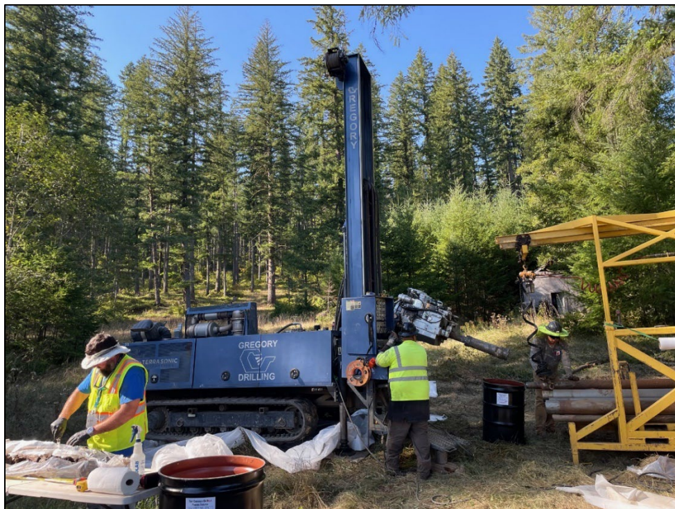
Photograph B-2. Sonic drilling and soil sampling activities at Building 1864 Former Fire Station location CBV-1864-06
