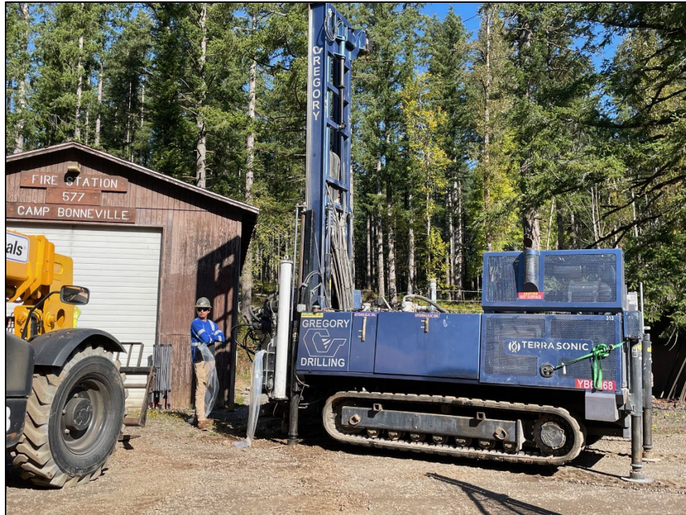
Photograph B-5. Sonic drilling and soil sampling activities at Building 4483 Former Fire Station location CBV-4483-05
