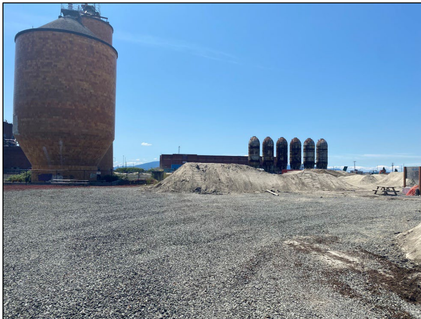
Photograph 4. Area northeast of the tile silos where the pump track was removed.
