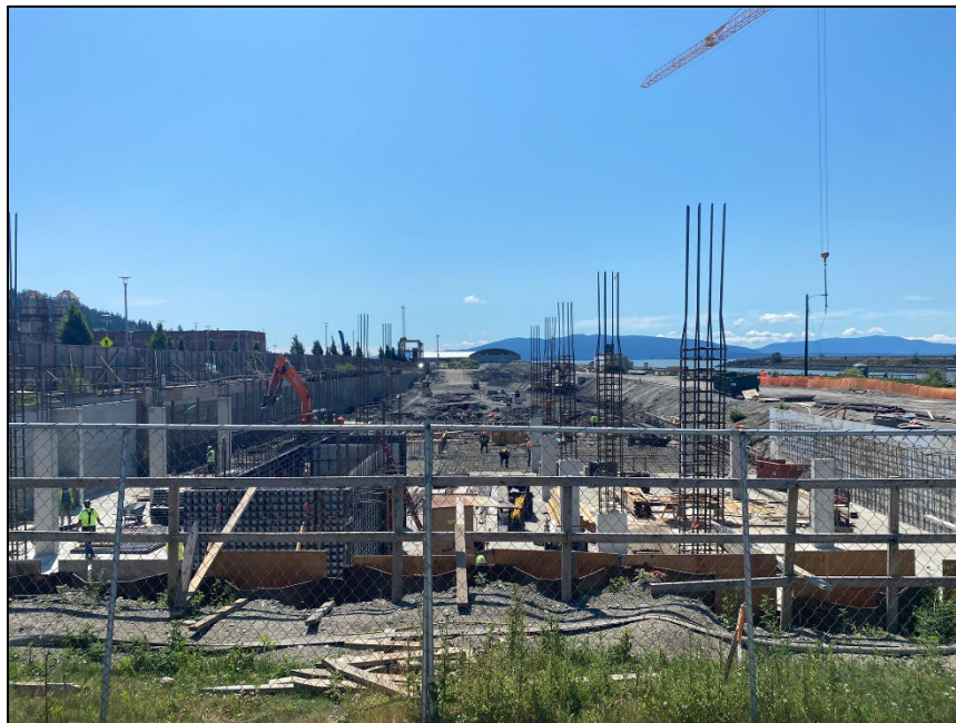
Photograph 6. Harcourt construction in process north of Granary Ave with temporary fencing on the left. Photo looking west.
