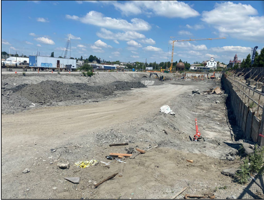
Photograph 7. Harcourt construction in process north of Granary Ave with temporary fencing on the right. Photo looking east.
