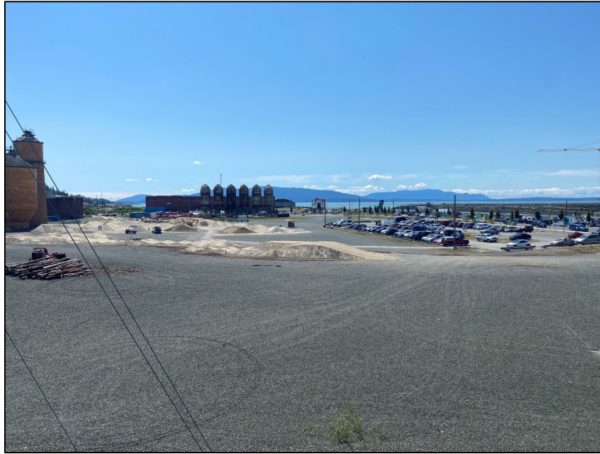
Photograph 5. View showing majority of cap area looking west.
