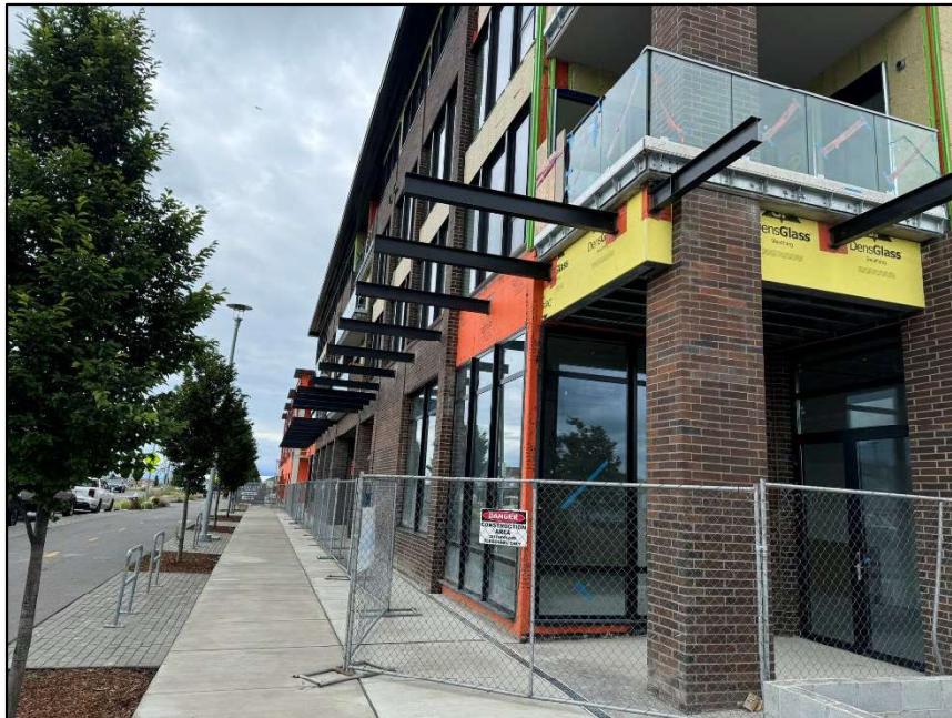
Photograph 8. Harcourt construction in process north of Granary Ave with temporary fencing. Photograph looking mill-west.
