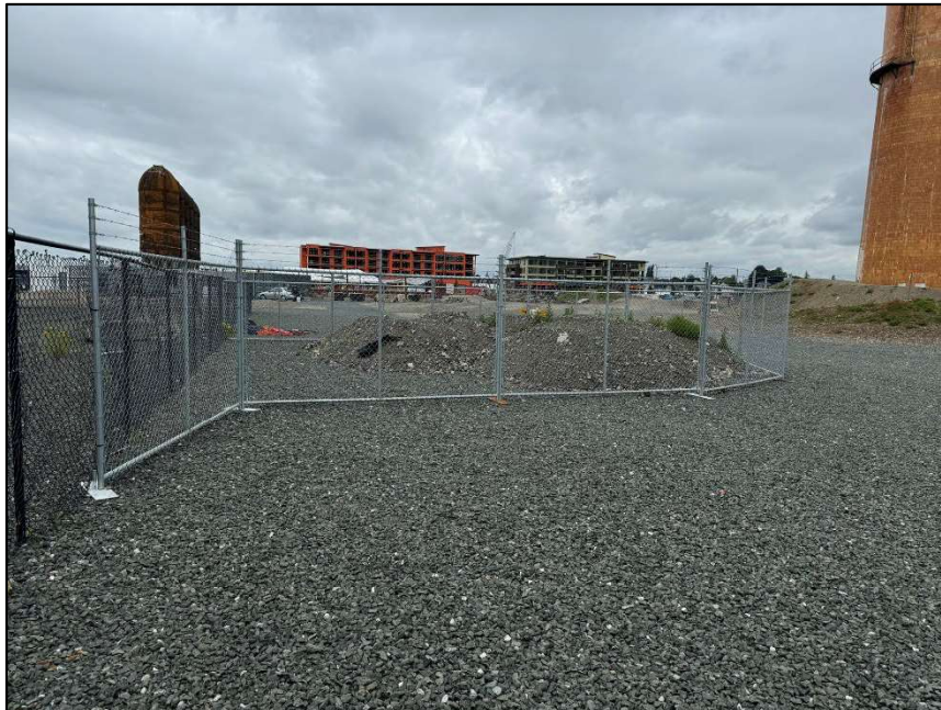
Photograph 4. Soil stockpile between the alcohol plant and the tile silos, protected by fencing. Photograph looking mill-north.
