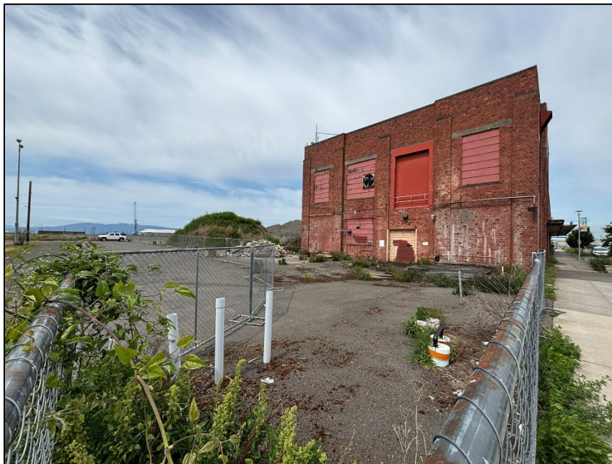
Photograph 4. Working area behind the Board Mill. Area is protected from public access by fencing. Photograph looking mill-northwest.
