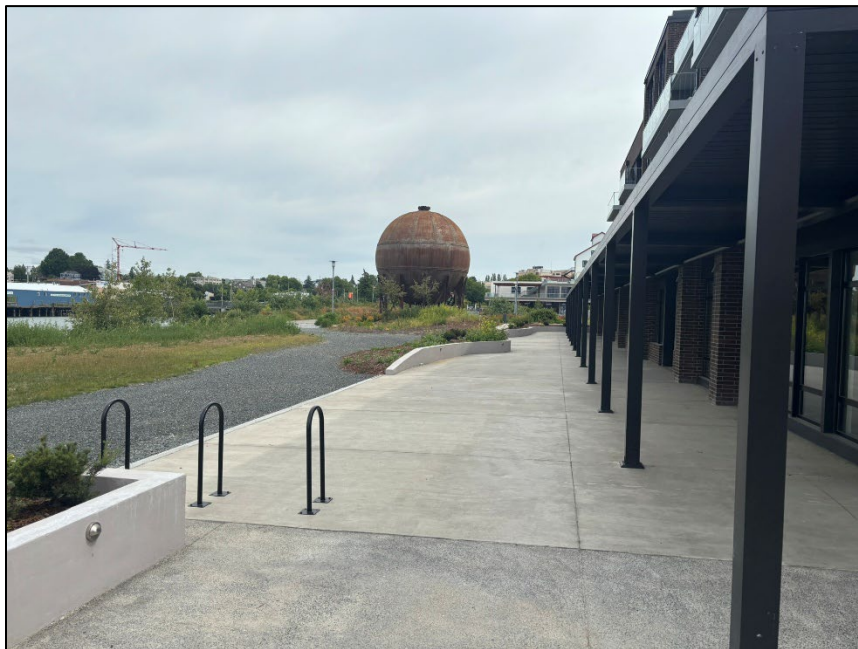
Photograph 8. Completed condo area with finished grading open to the public. Photo looking mill-east.
