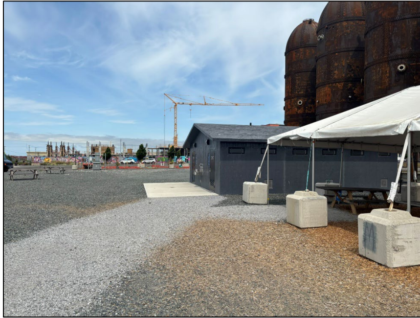
Photograph 9. New bathroom structure to the mill-west of the digester towers. Photo looking mill-north.
