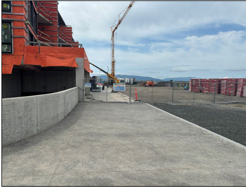
Photograph 7. Harcourt construction in process north of Granary Ave with temporary fencing on north side. Photograph looking mill-west.
