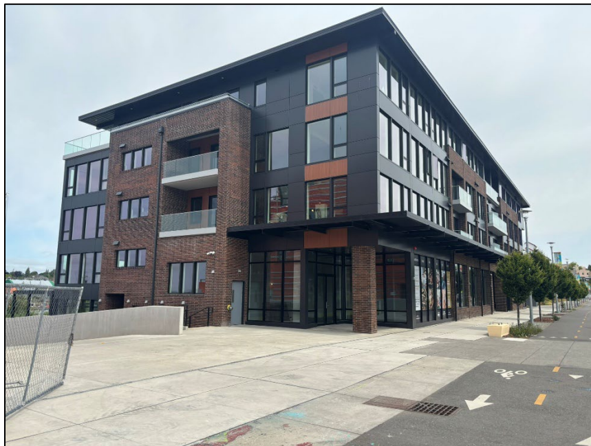
Photograph 6. Completed condo with finished grading open to the public. Photo looking mill-northeast.
