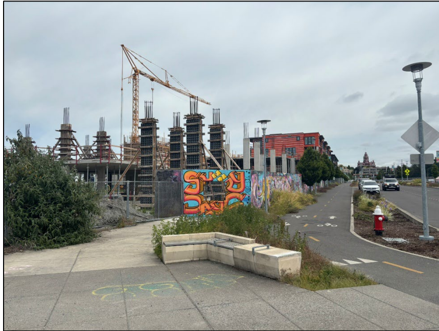
Photograph 5. Harcourt construction in process north of Granary Ave with temporary fencing. Photograph looking mill-east.
