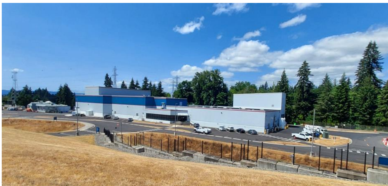
Photo of Hazardous Materials Building (HMB) – BPA Ross Complex, courtesy of Bonneville Power Administration.
