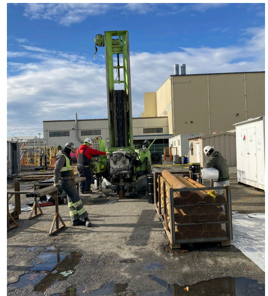
Figure 2: Soil boring and well installation, Building C-29, Nov 2022
