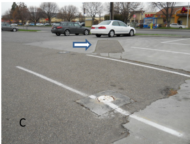
Figure 3. Site Photos (A) looking to SE, (B) looking to NE, (C) previous location of gas dispensers (see arrow)
