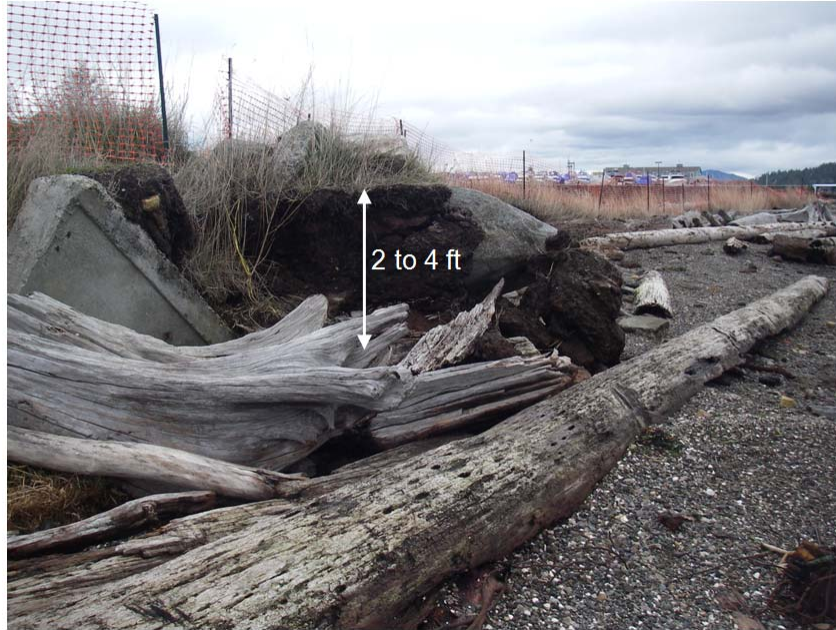
Figure 2. Erosion evident along shoreline at south end of project
