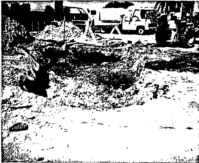
July 1996 - Excavation prior to plastic lining
