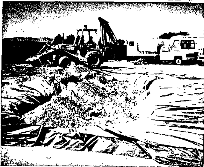
July 1996 - Excavation area with plastic lining and PCS contaminated soil
