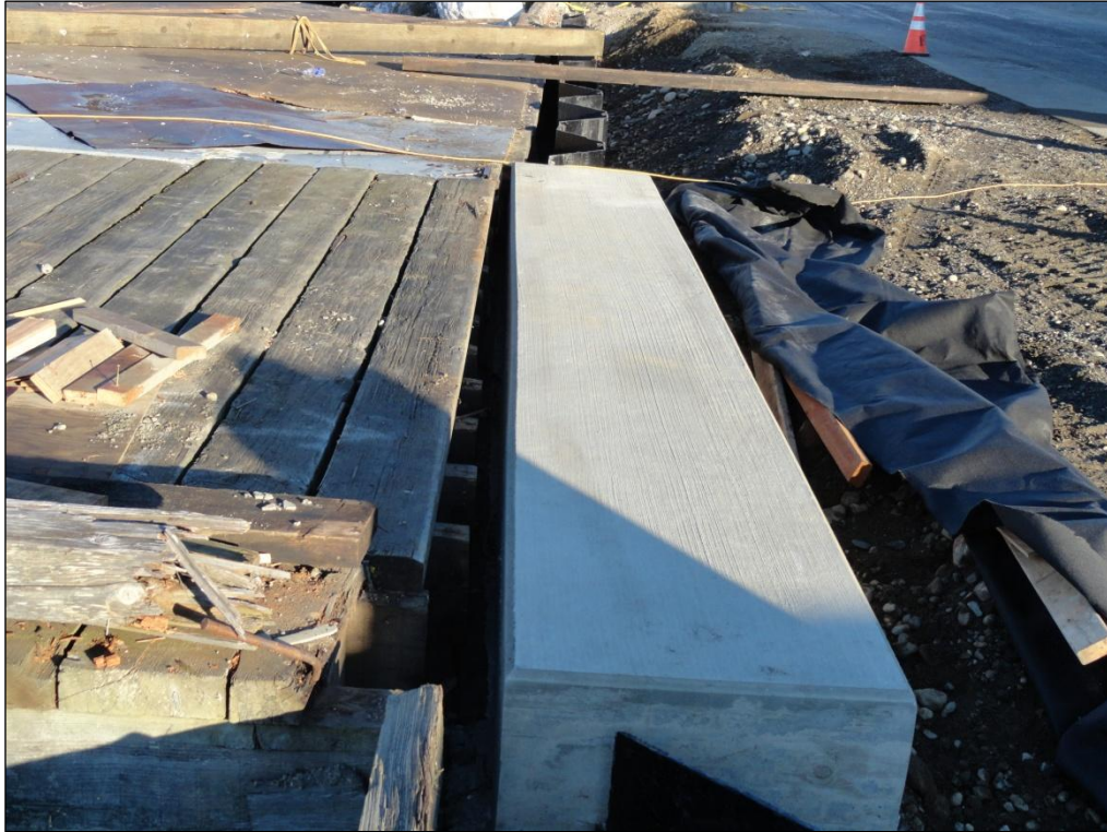
5. Completed pile cap.
