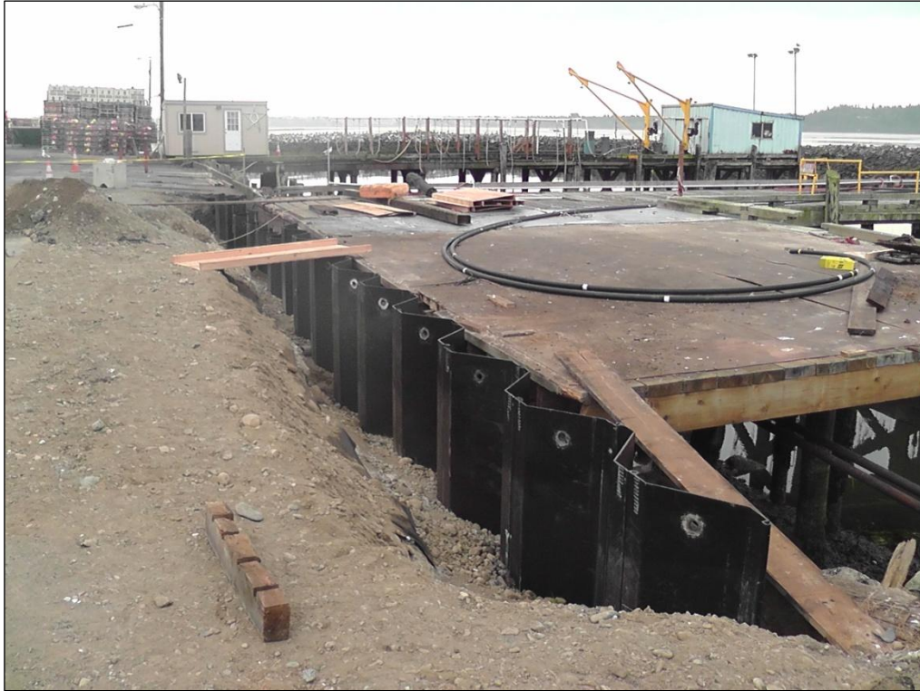
3. Installed bulkhead.
