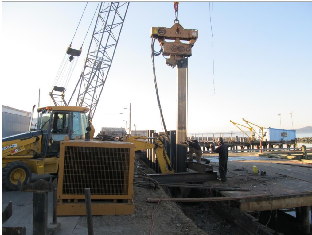
2. Installation of bulkhead sheetpiles.
