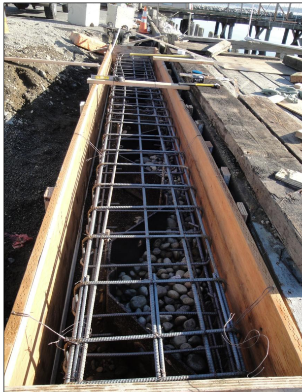
4. Pile cap form in front of fuel dock.
