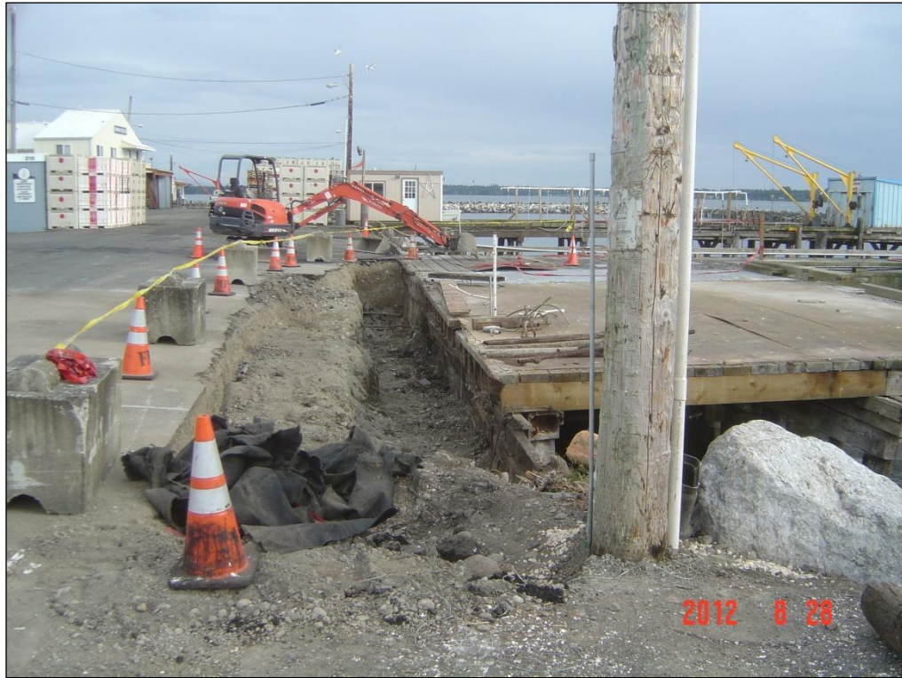
1. Construction trench for bulkhead installation.
