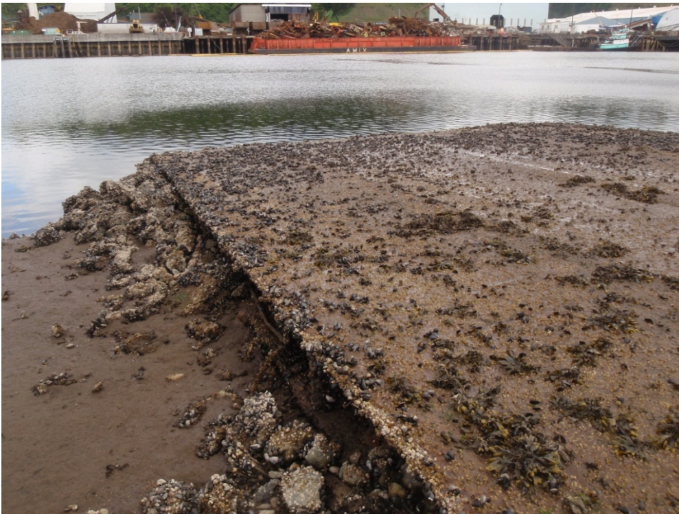
Photograph 2. The existing concrete ramp, facing north. Tidal elevation is approximately +3 ft MLLW.
