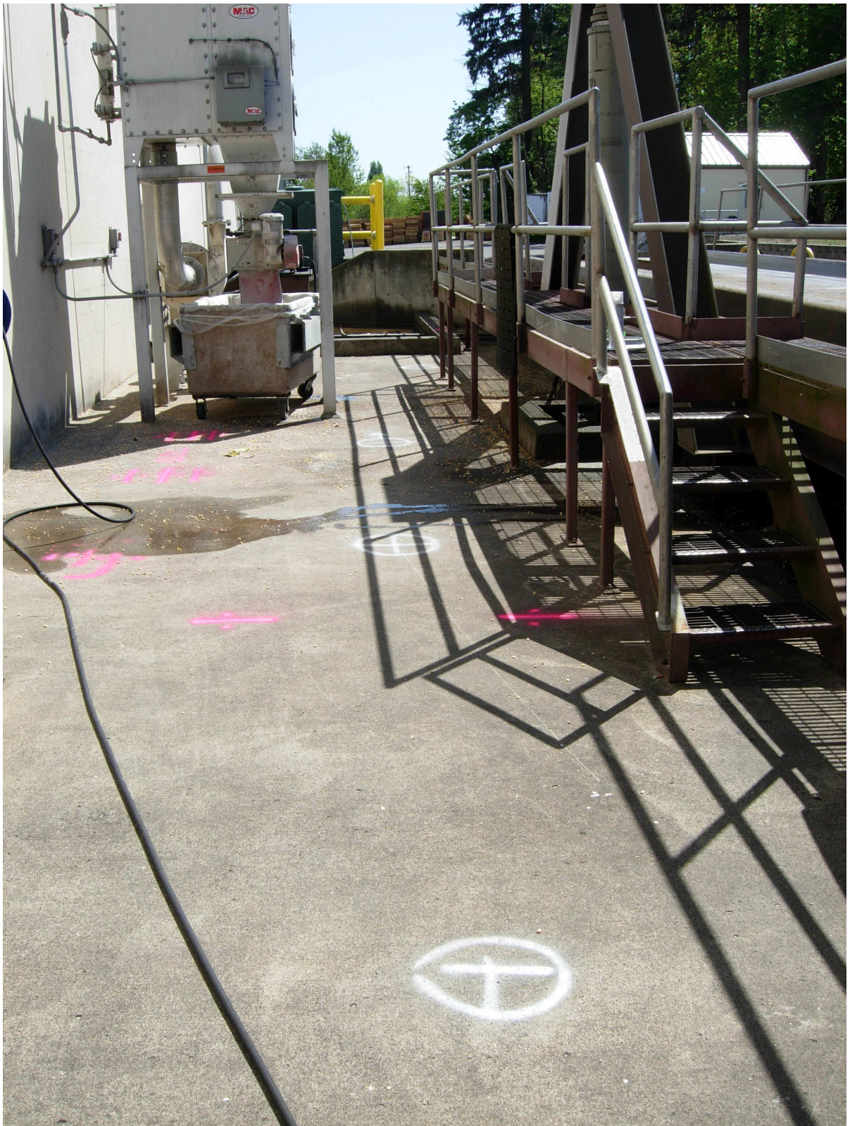
Photo 3: Sample locations East side of lift, looking south. FL-04 in foreground. Note U/G power to right, crossing to lift, rams beyond stairs to right.
