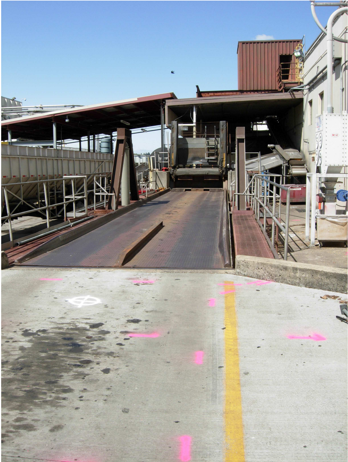
Photo 2: Ramp with hydraulic lift beyond, looking North. FL-08 in foreground on concrete ramp.
