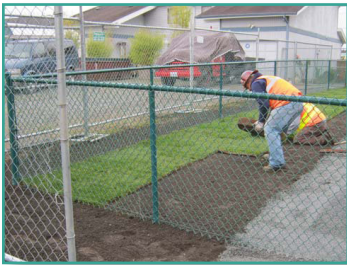
The property will be restored after soil has been excavated.
