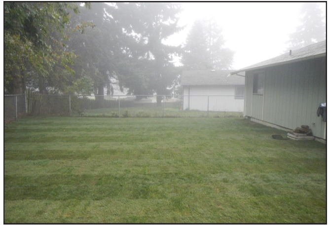
Sod is installed to replace the lawn area.
