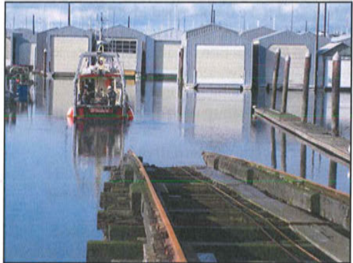
Sediment sampling is conducted just beyond the Marine Railway, which was used to move boats from the water to the Everett Shipyard, Inc. Site.
