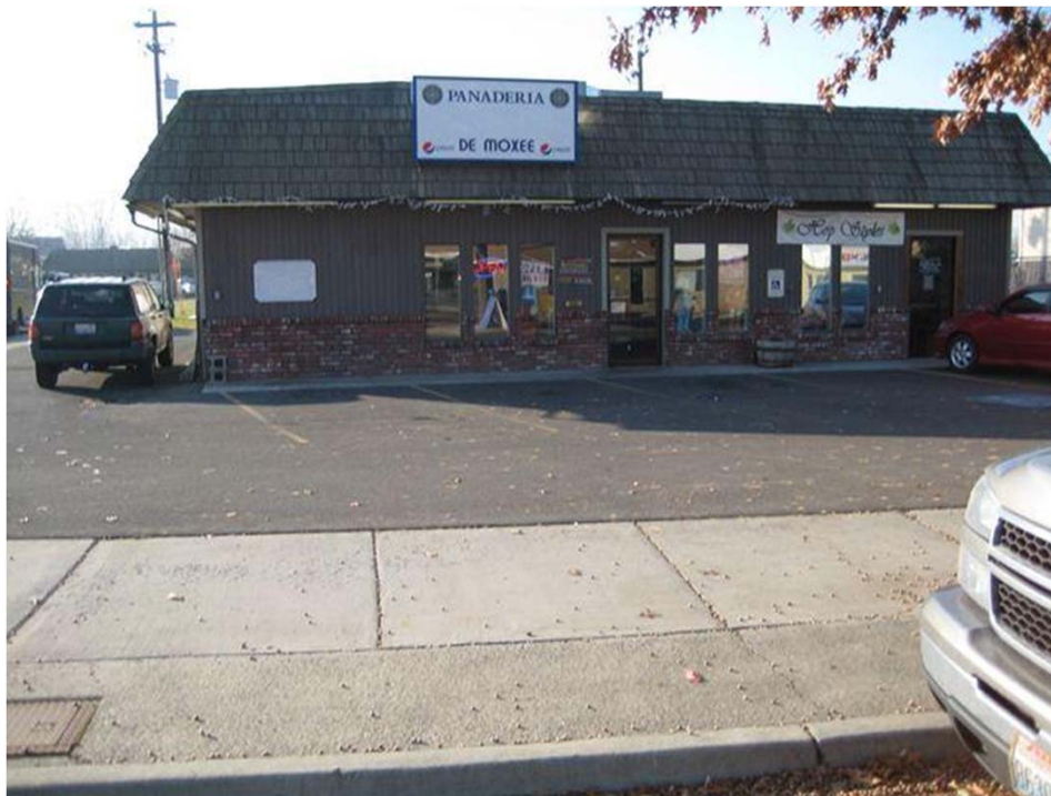
View of existing site building (view to southwest)
