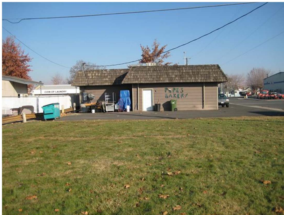
View of existing site building (view to northeast)
