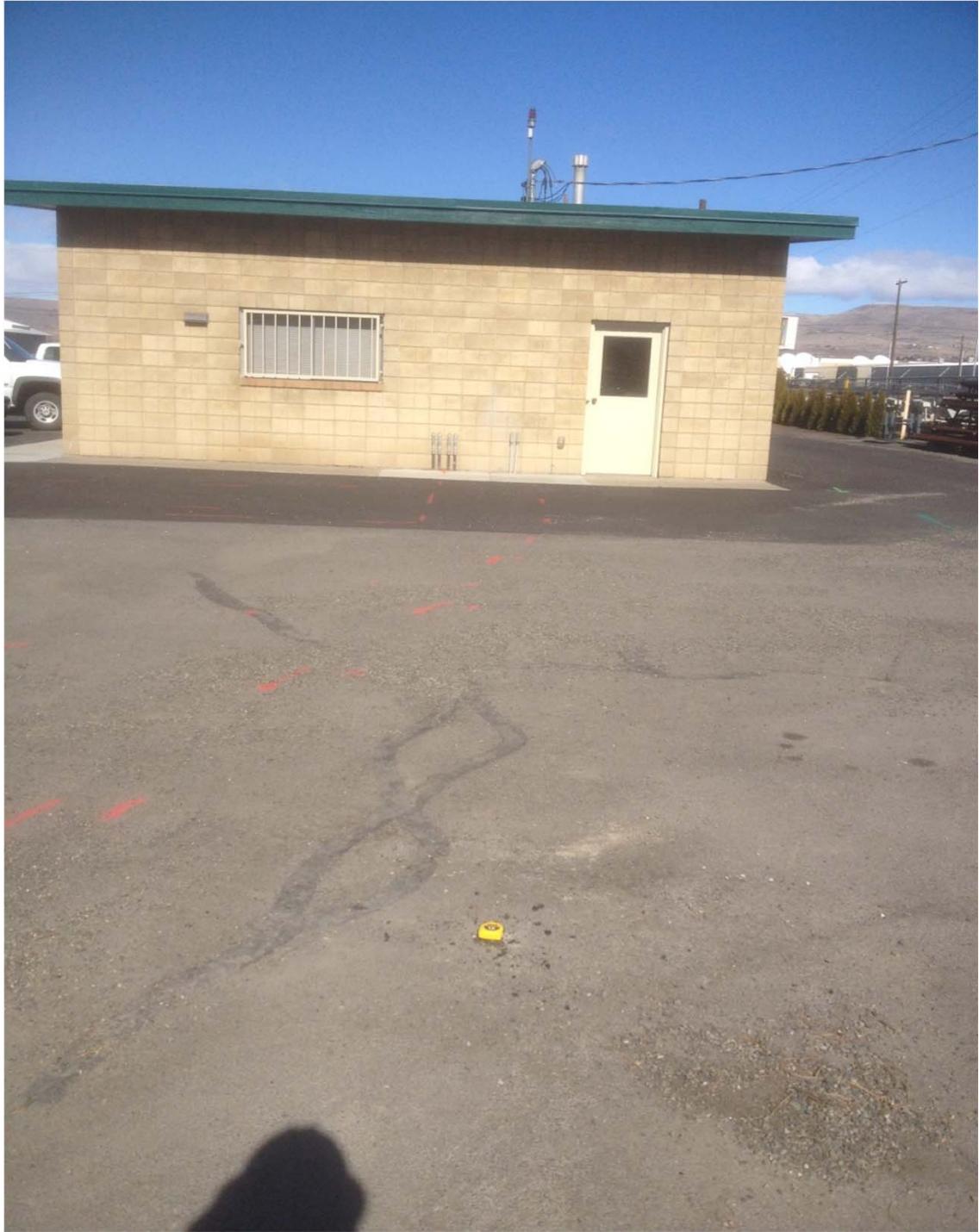
View of south shop building with boring DP-3 in foreground (view to northwest)
