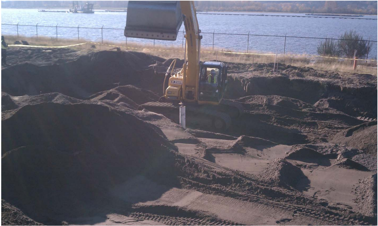
Photograph 1: Excavation of soil in CaSx application area.
