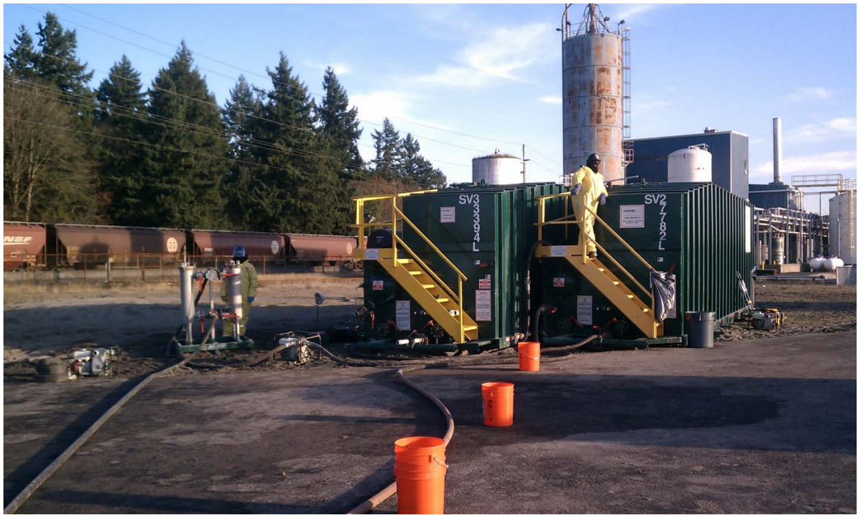
Photograph 15: Injection & re-circulation equipment.
