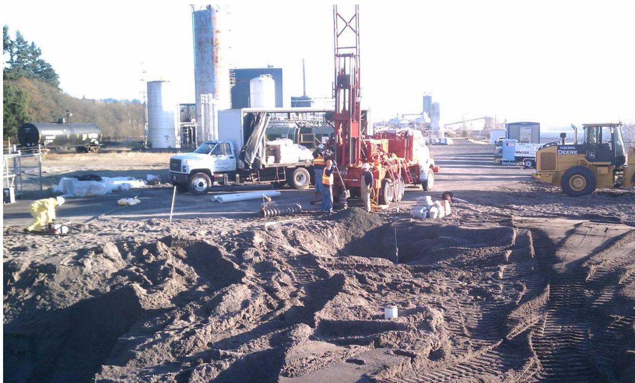
Photograph 12: Extraction well installation.
