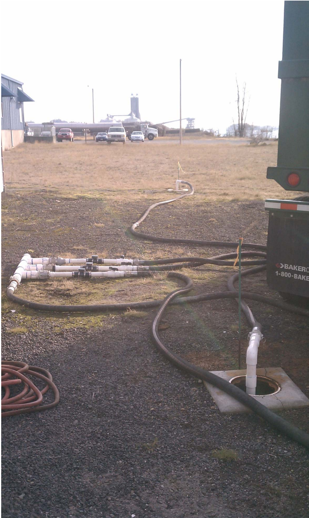
Photograph 19: Injection manifold.
