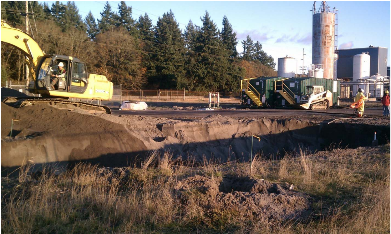
Photograph 6: Excavation and preparation for application of CaSx.
