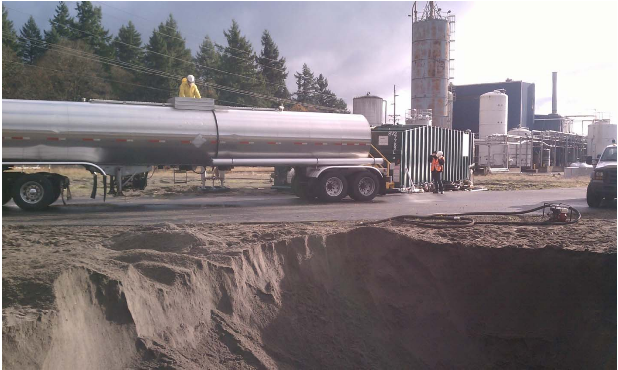
Photograph 5: CaSx delivery and transfer into frac tank.
