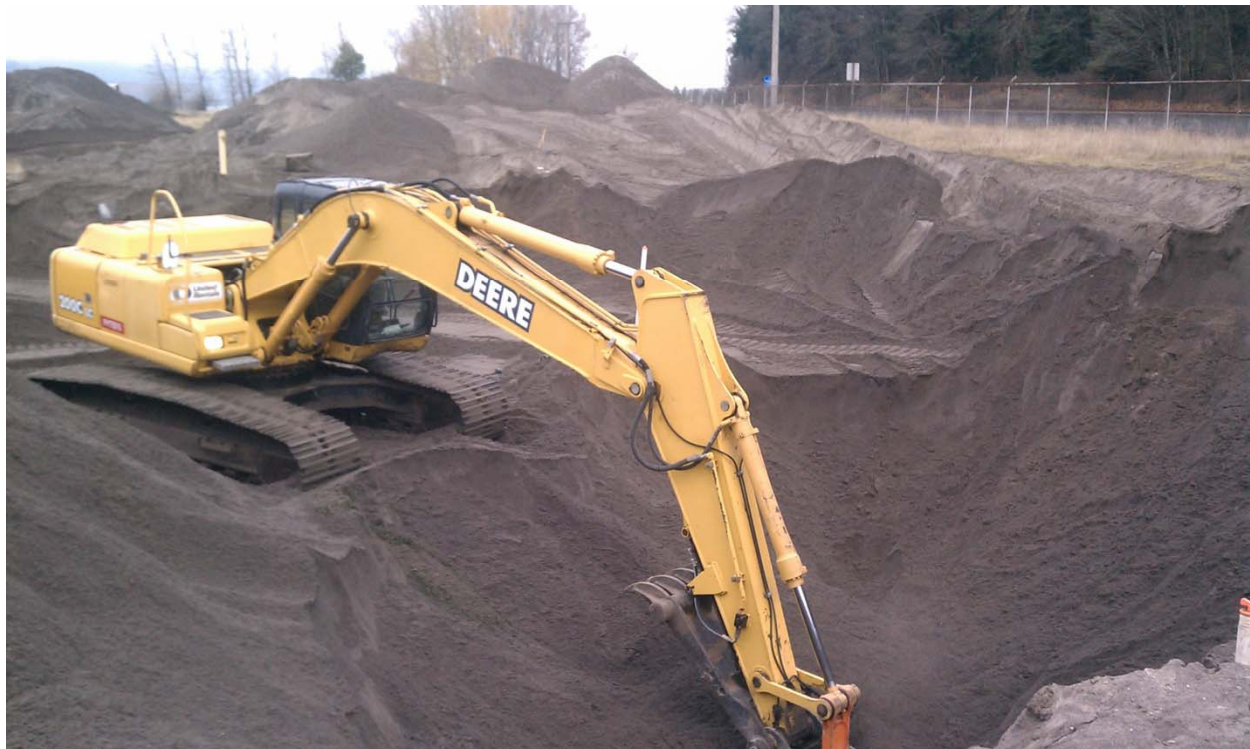
Photograph 4: Excavation of soil in CaSx application area.
