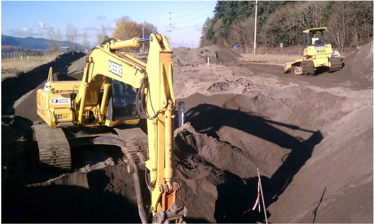
Photograph 3: Excavation of soil in CaSx application area.
