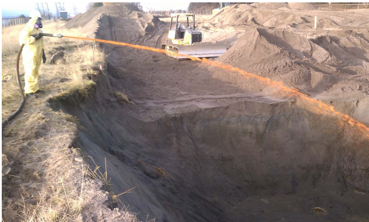
Photograph 8: Application of CaSx to base of excavation.
