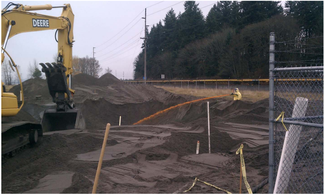
Photograph 9: Application of CaSx to base of excavation.
