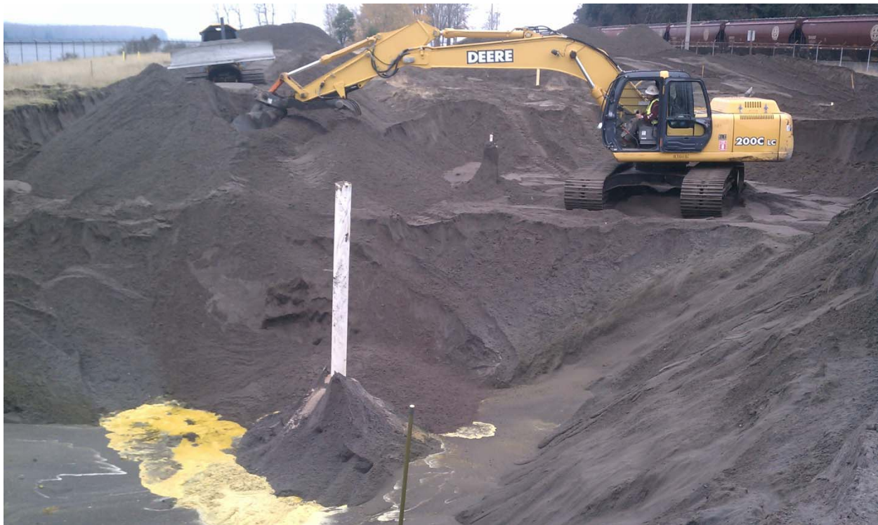
Photograph 10: Backfilling after application of CaSx to base of excavation.
