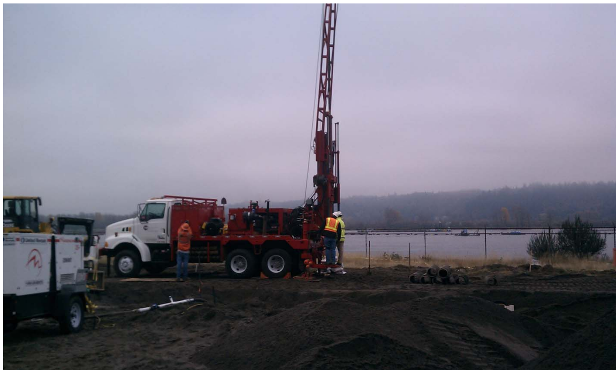
Photograph 11: Extraction well installation.
