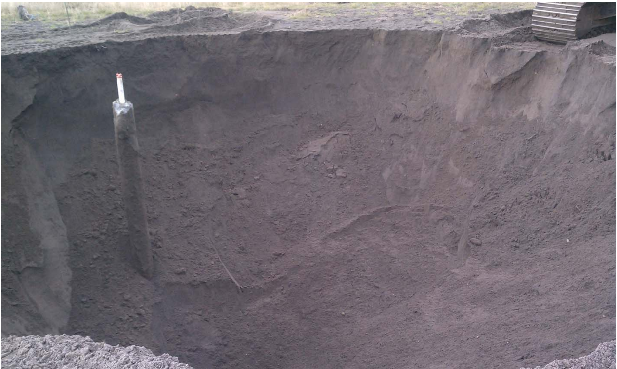
Photograph 2: Injection well exposed during soil excavation.
