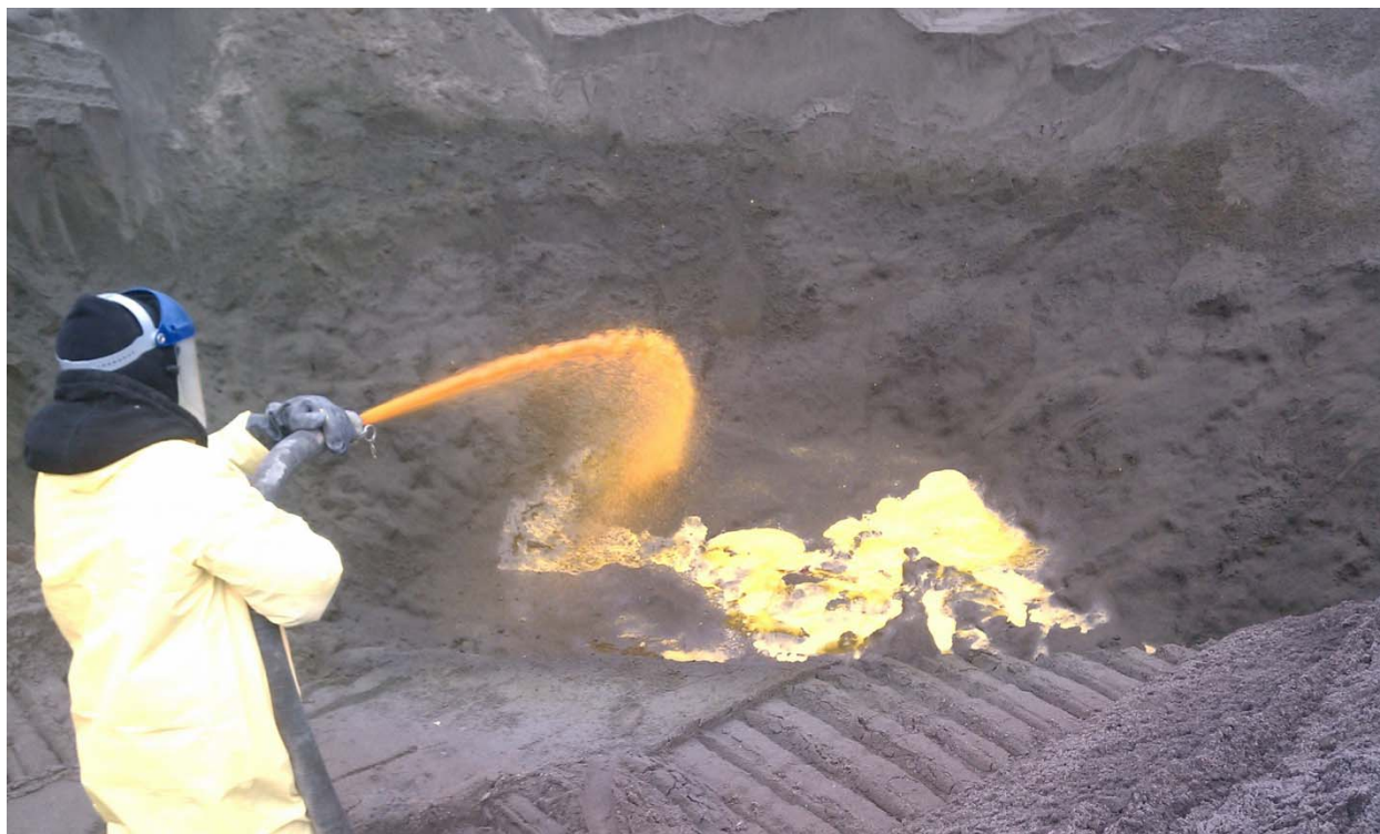
Photograph 7: Application of CaSx to base of excavation.
