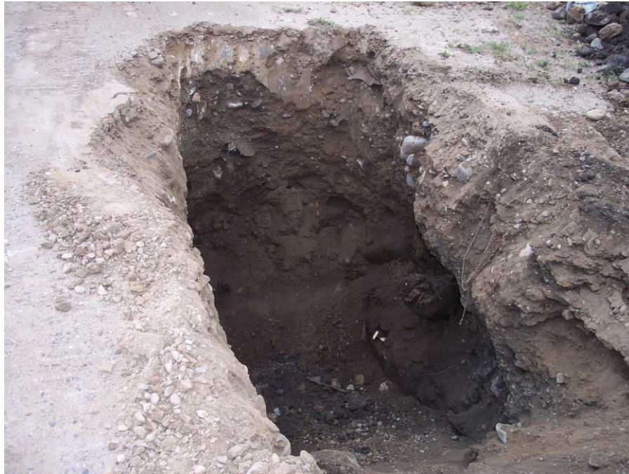
Figure 3. Test pit 35 nearing the water table at 7 ft. below surface.
