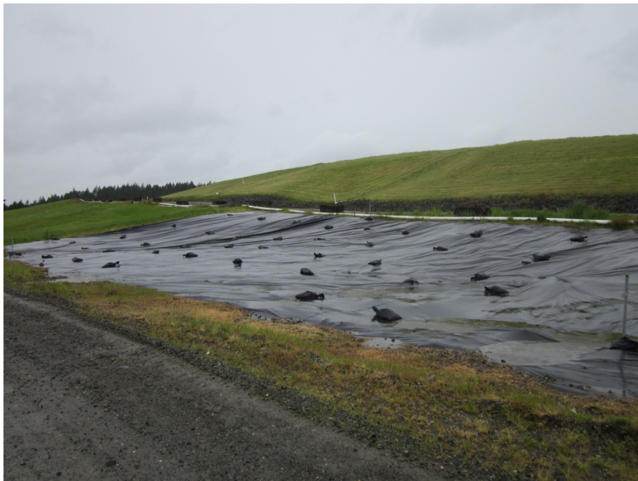
Photo 12. View of south slope of landfill, facing northwest. Photograph taken on 5/23/12.
