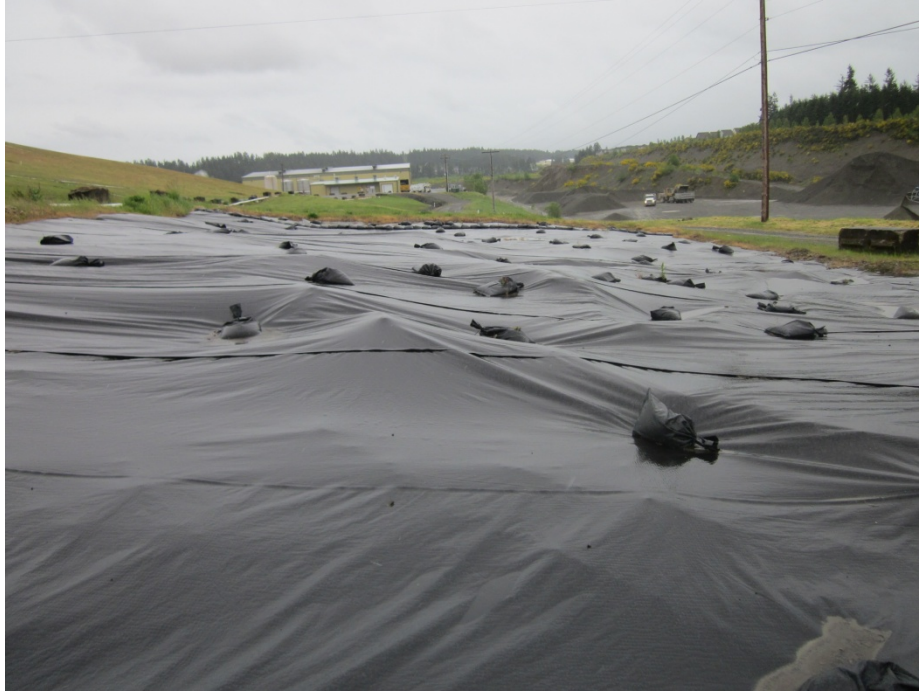
Photo 11. View of south slope of landfill, facing the leachate treatment plant and transfer station. Photograph taken on 5/23/12.
