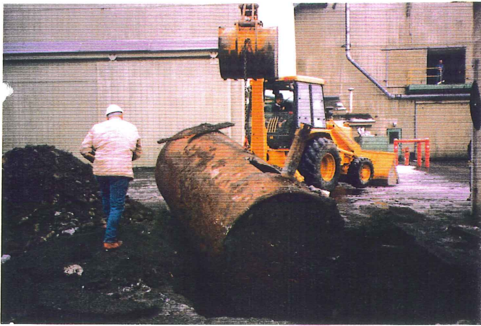
Photo 4. Tank being lifted from pit.
