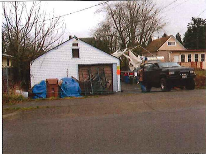
Street view of the Phillips property showing the garage, concrete pad and driveway, and the dilapidated carport.
