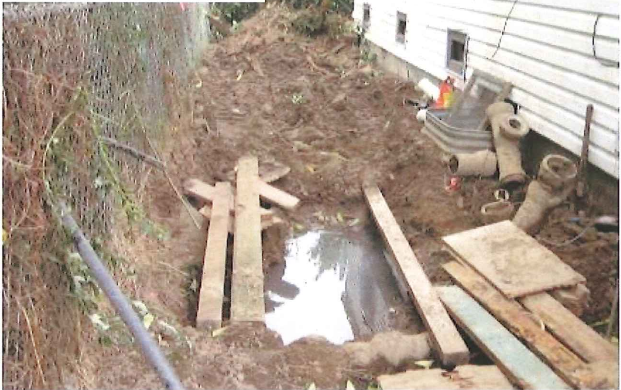
Along North side of house where work to fix side-sewer was occurring. Puddle of sewage and plumbing debris.
