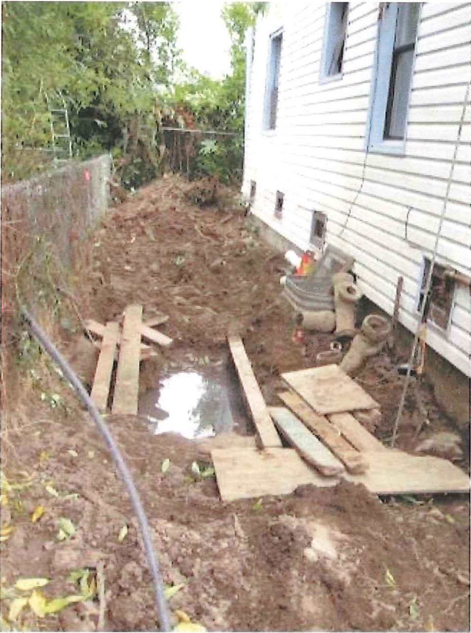
Side sewer work area – north west corner of house
