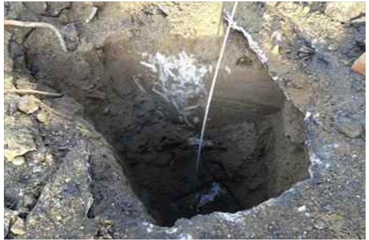
Photograph 4: View of concrete footing of former building, encountered on the north wall of the excavation.
