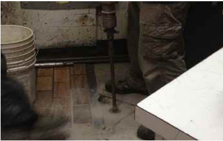
Photograph 1: Advancing boring B6 (attempt 1 of 3), adjacent to the freezers.
