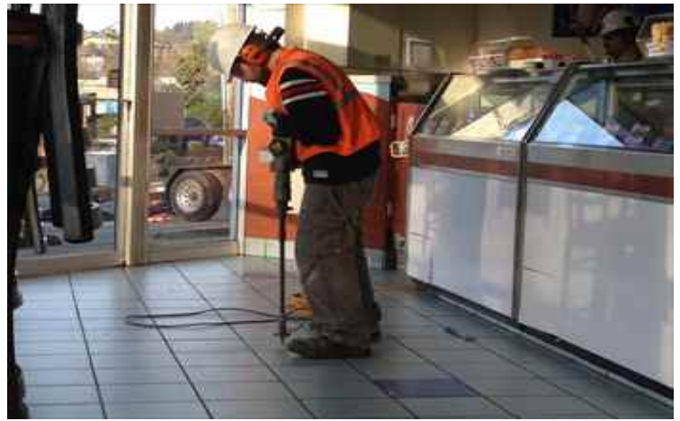
Photograph 2: Advancing boring B7, refusal encountered less than 1 foot bgs.
