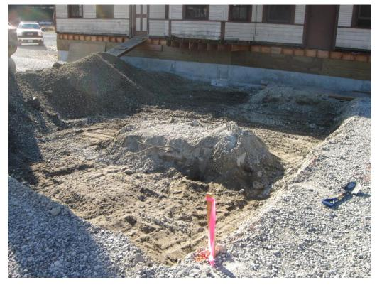
**Photograph 4**: Area B: View from FC-005 looking southeast at building footings encountered during excavation.
