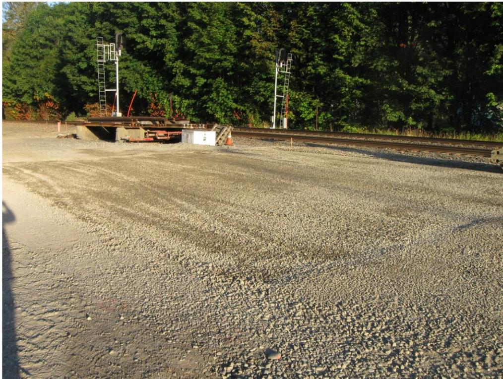
**Photograph 3:** Area A: View from FC-004 looking northwest following compaction of backfill aggregate.
