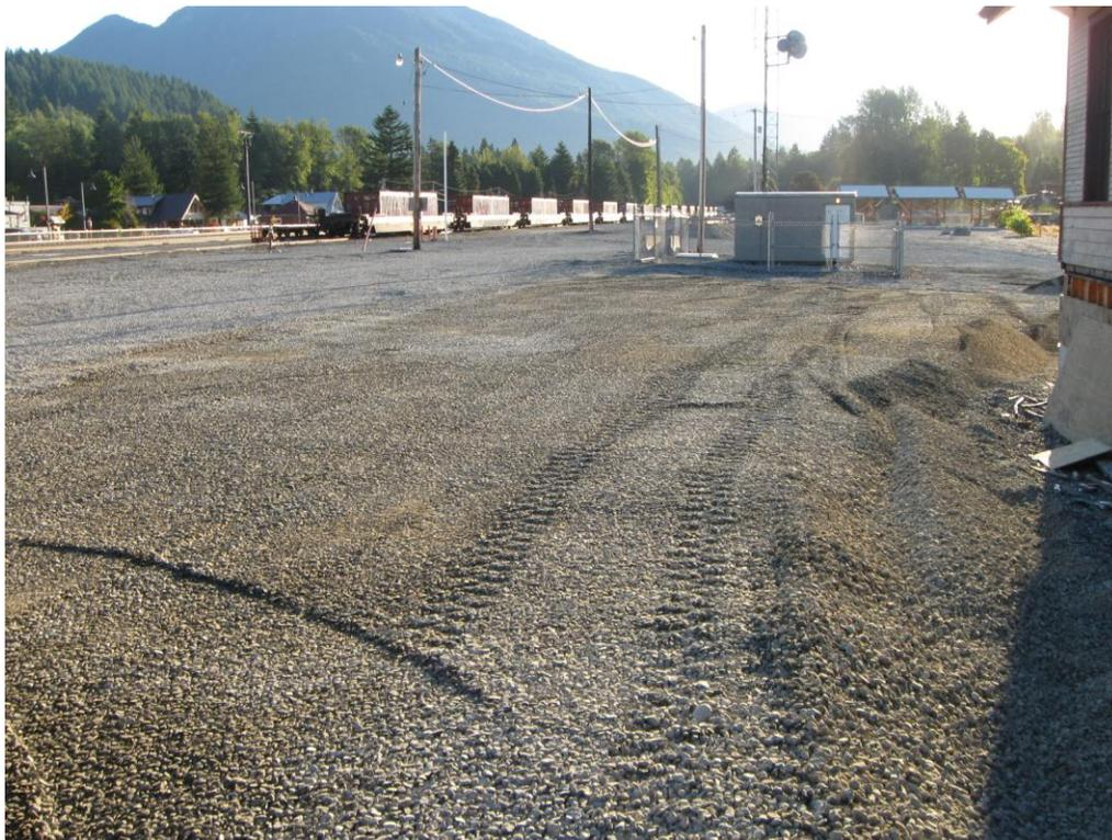
**Photograph 7:** Area B: View from FC-007 looking east following compaction of backfill aggregate.
