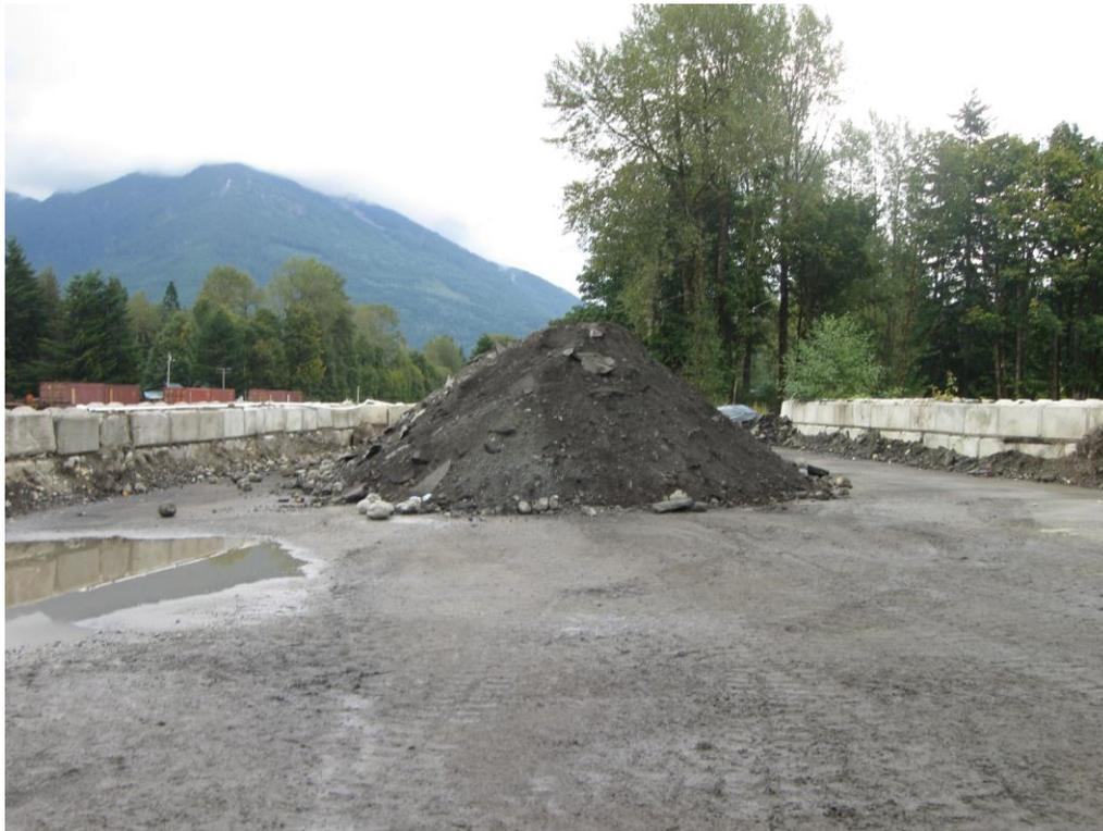
**Photograph 9:** Area C: View from FC-012 looking east at metals-impacted soil stockpiled in soil-handling facility.
