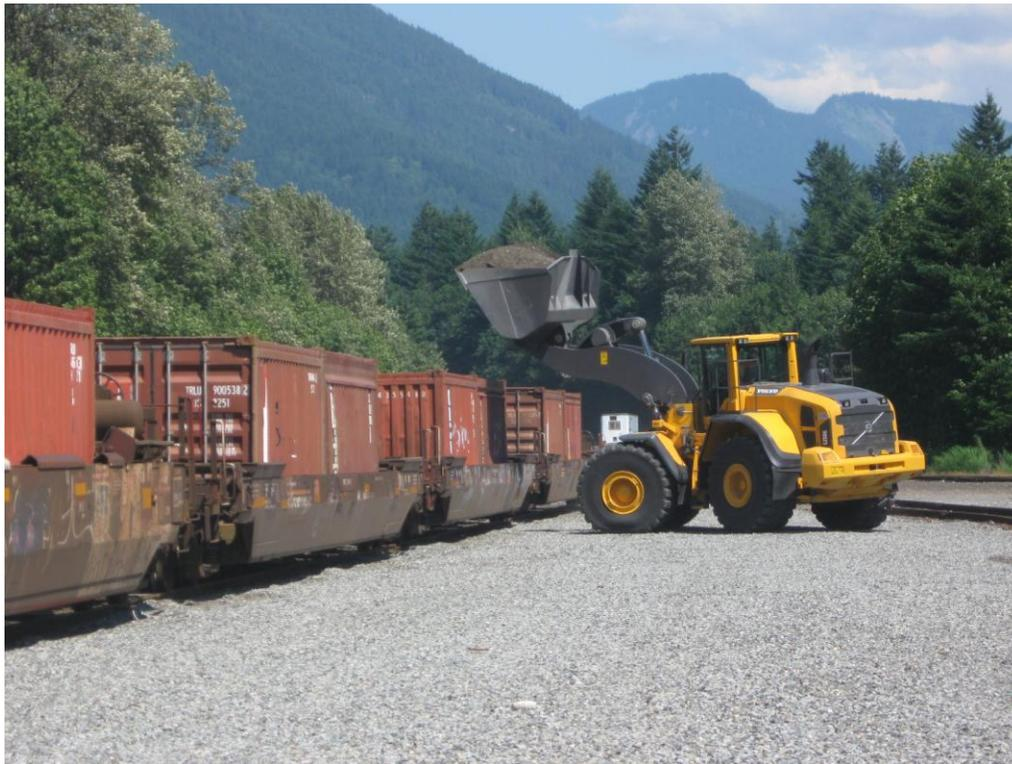
**Photograph 11:** Loadout: View from soil-handling facility looking east at railcars being loaded with impacted soil.
