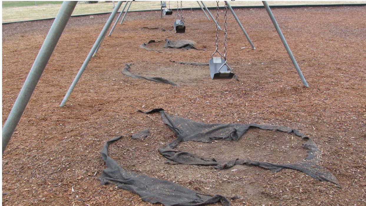
Photo 2: Torn Geotextile and Exposed Soil Beneath Swings - from the east
