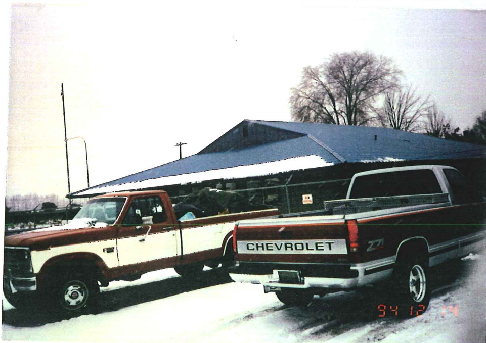
Photograph 3: Looking South- A office building.
