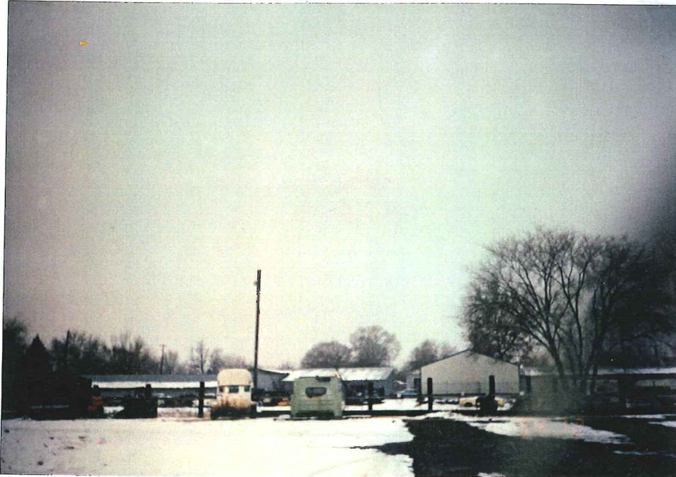
Photograph 2: Looking West- Industrial metal buildings.
