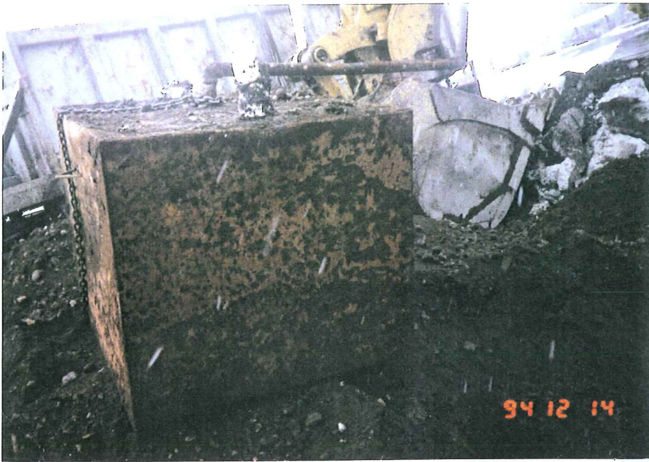
Photograph 4: Condition of tank from excavation #1.
