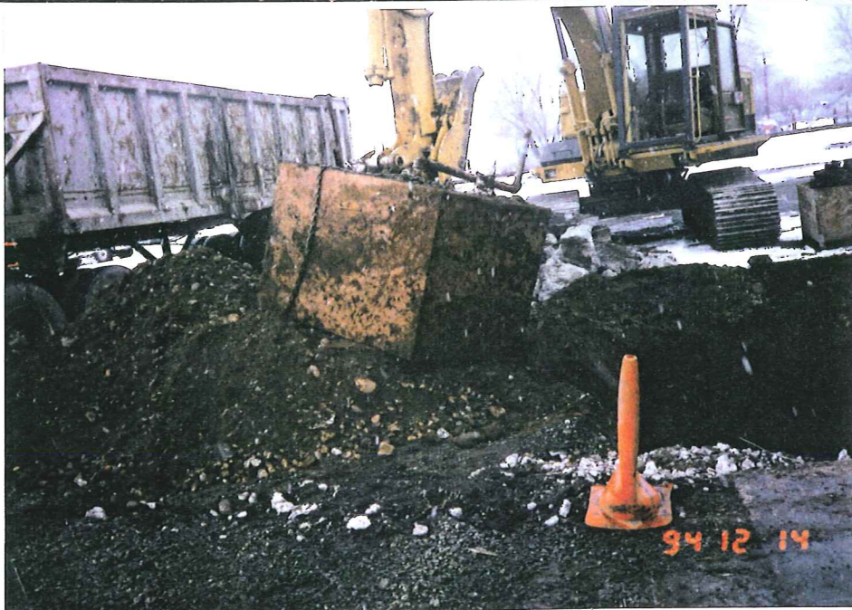
Photograph 5: Condition of tank from excavation #2.
