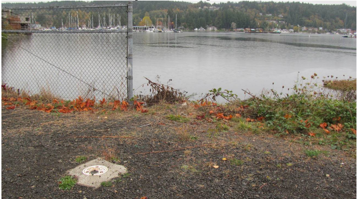
Photo 4: Conditional Point of Compliance Wells along Waterfront – from the west
