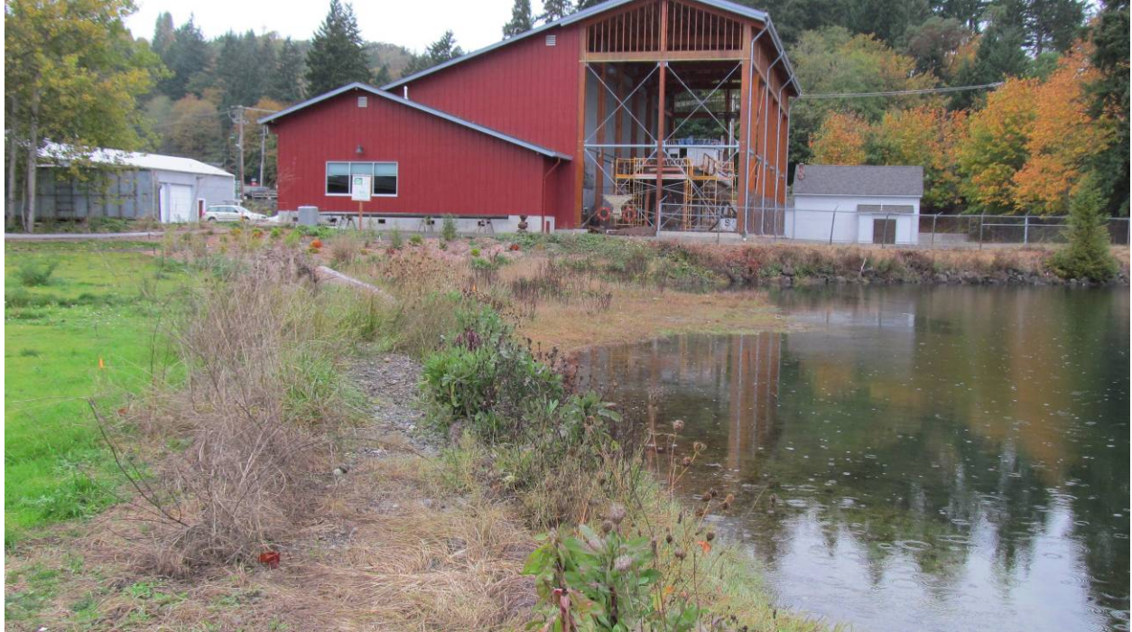
Photo 3: Gig Harbor Waterfront Southeast of Site – from the South
