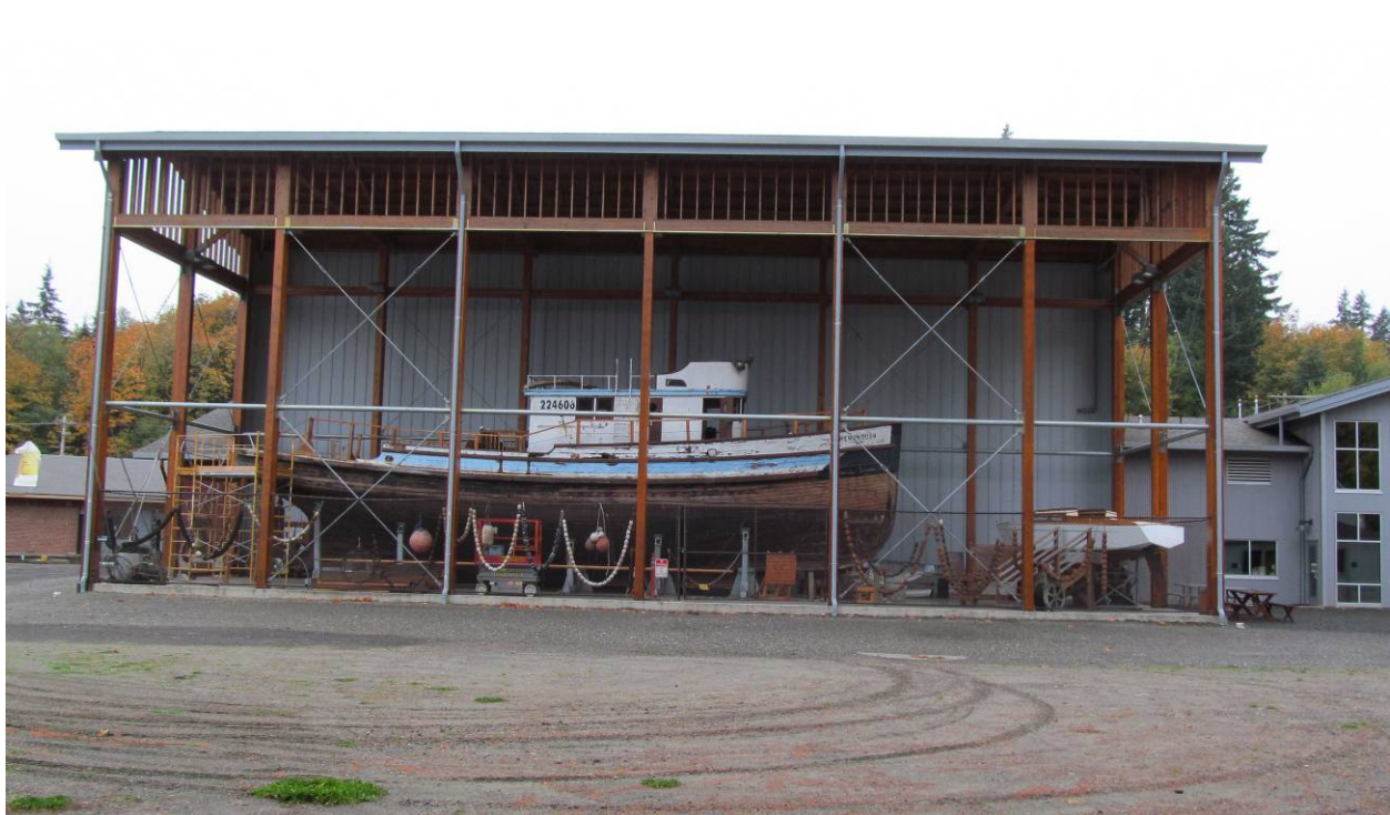
Photo 2: North Gravel Parking Lot and Boat Storage Area – from the north
