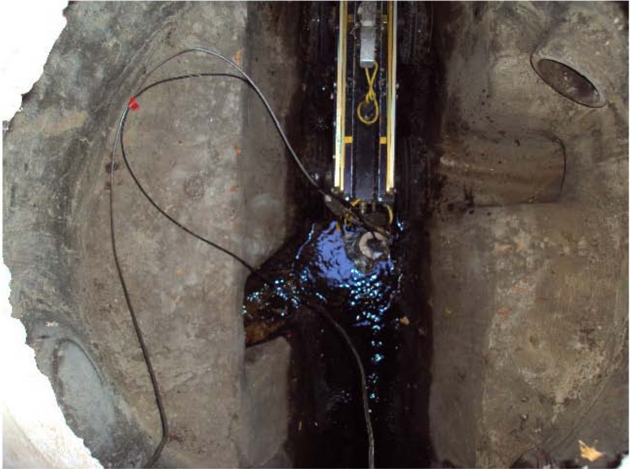
Figure 29 Concrete Construction Inside Manhole MH-136
