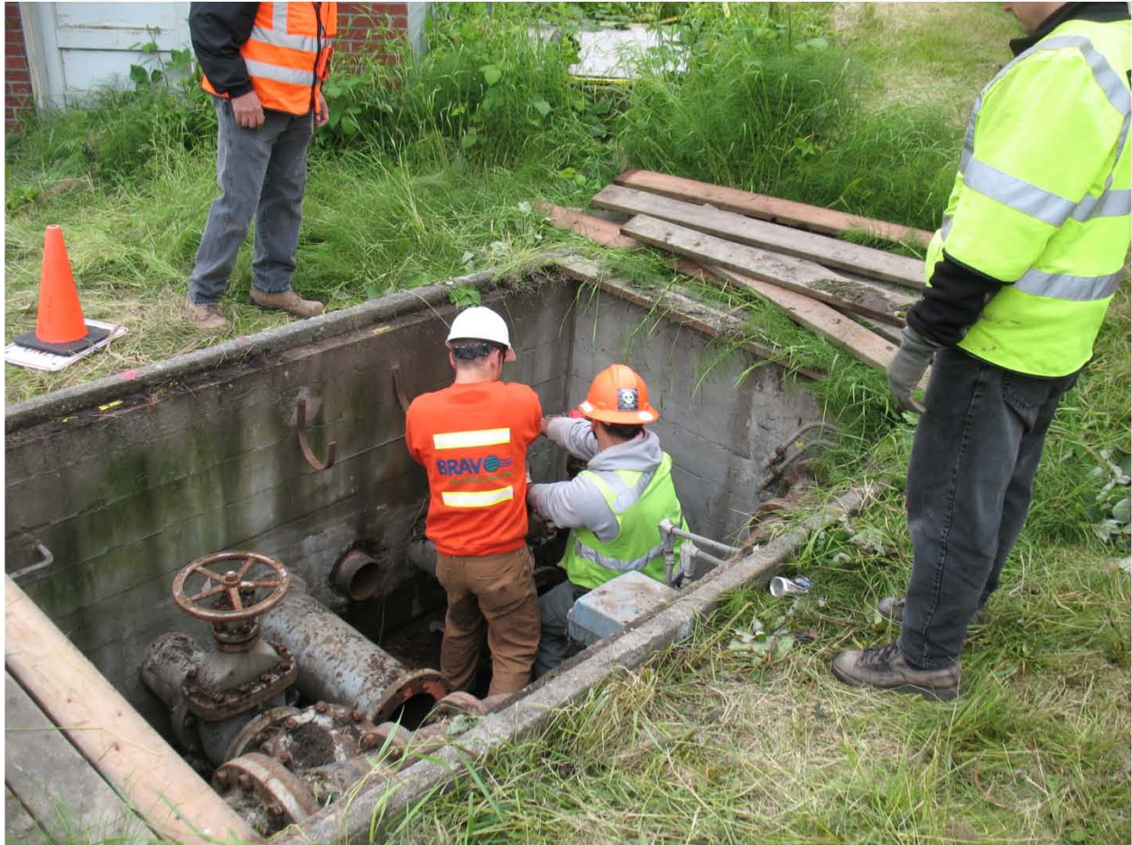
Figure 6 Pump House 98 Valve Pit
