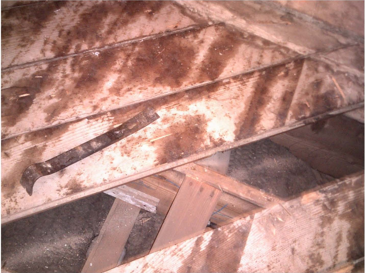
Figure 14 Radium Room Floor – Joist Space
