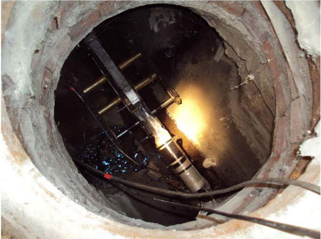
Figure 28 Concrete and Brick Construction Inside Manhole MH-135
