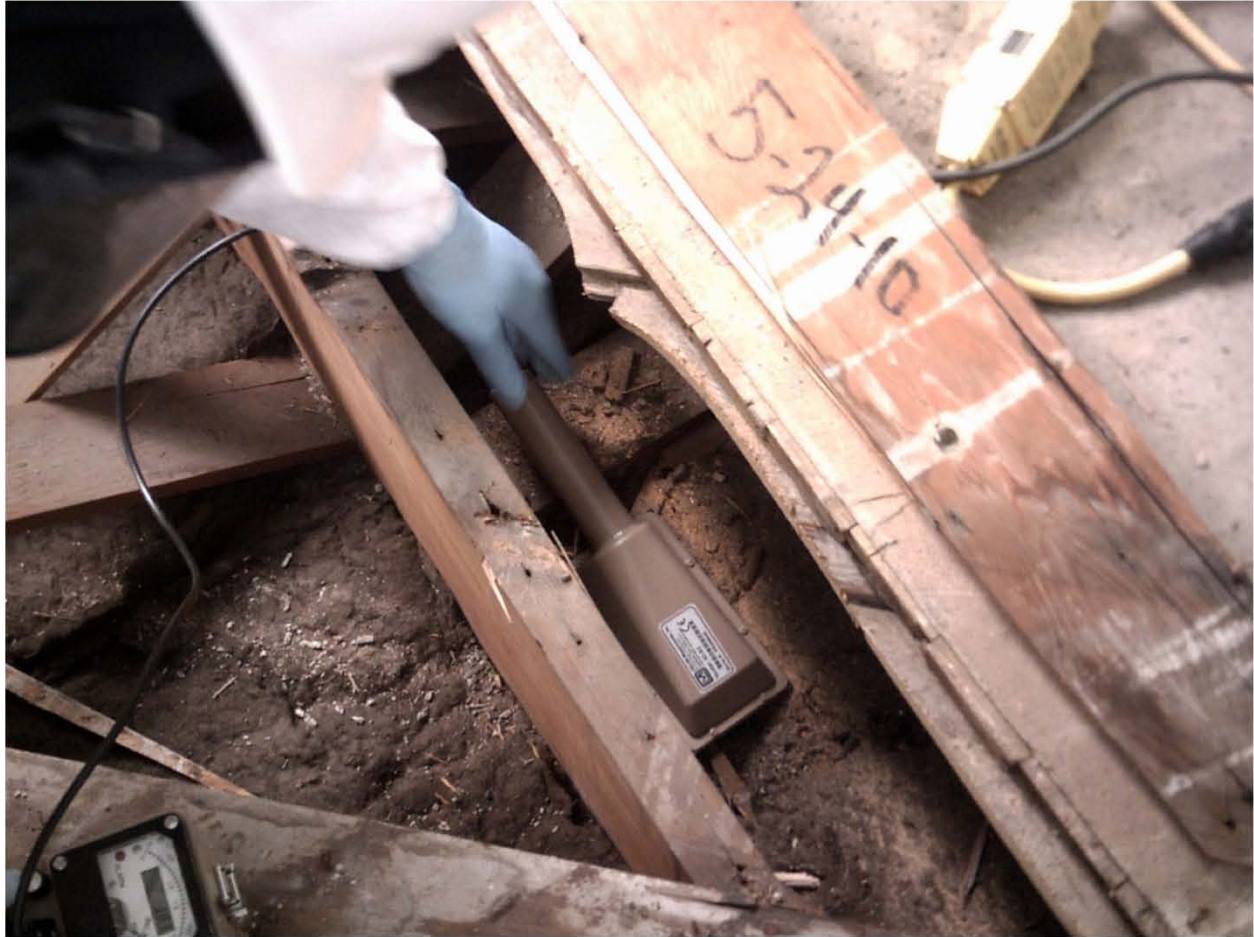
Figure 15 Survey of Floor Joist Space (Insulation) – Safety Chief Office
