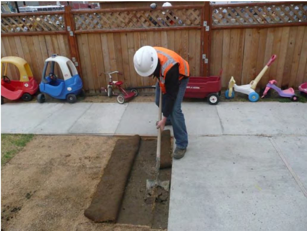
Photo 50 - Collecting additional confirmation samples for characterization of backfill material. 6/05/12
