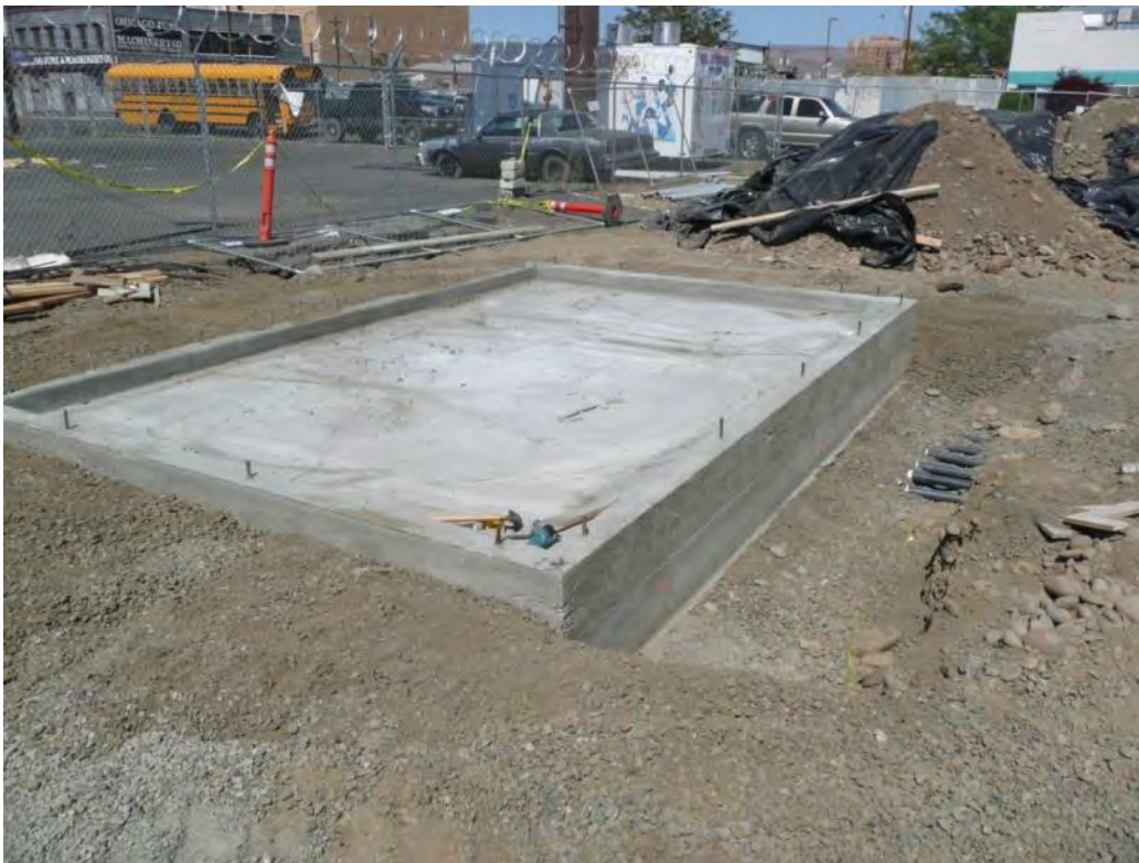
Photo 34 - Removing forms and compaction around SVE utility building foundation. 5/14/12
