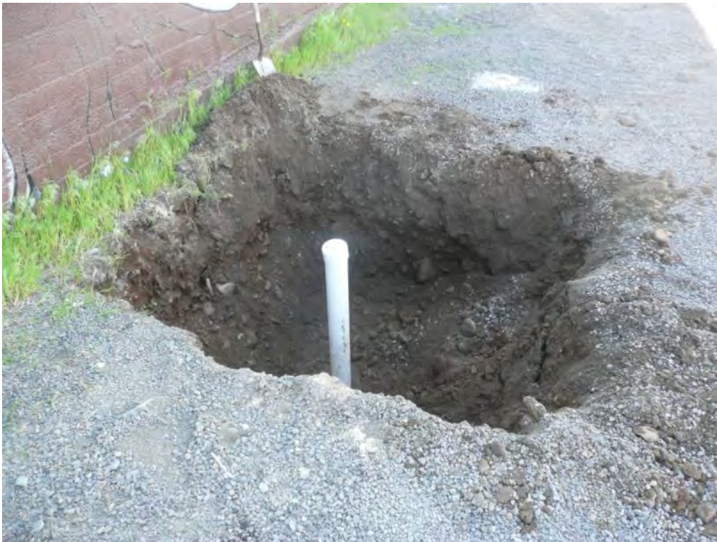
Photo 2 - Excavating around SVE wells. 4/23/12
