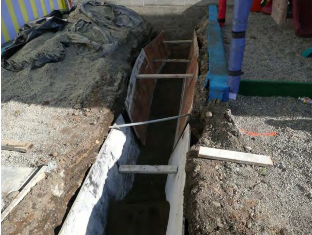
Photo 9 - Trench approximately 2 feet in depth with temporary shoring. 4/26/12
