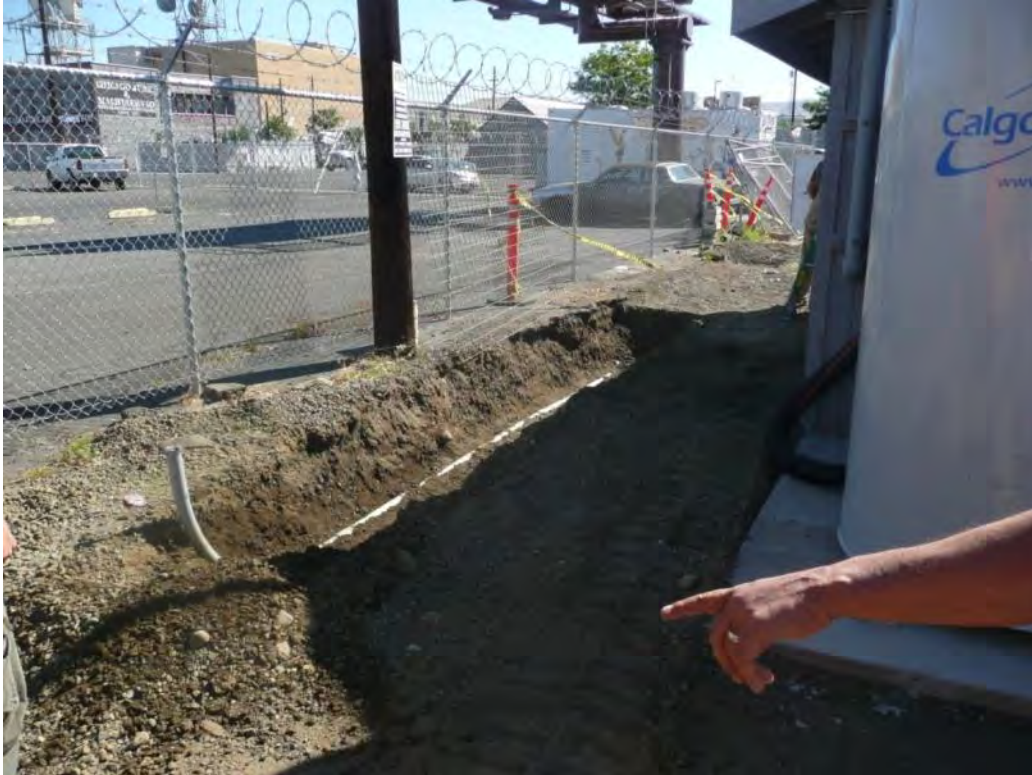
Photo 57 – Spare conduit stubbed up to connect electrical to service disconnect panel. 6/15/12
