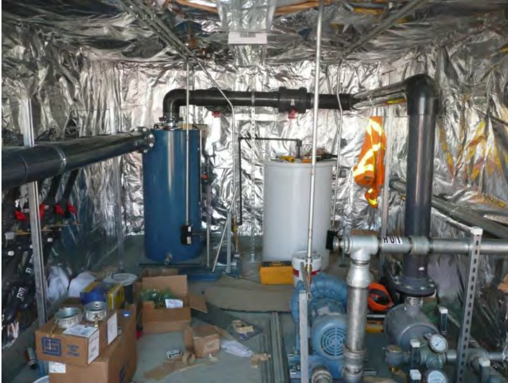
Photo 67 - Insulation and foilback inside SVE utility building. 6/27/12
