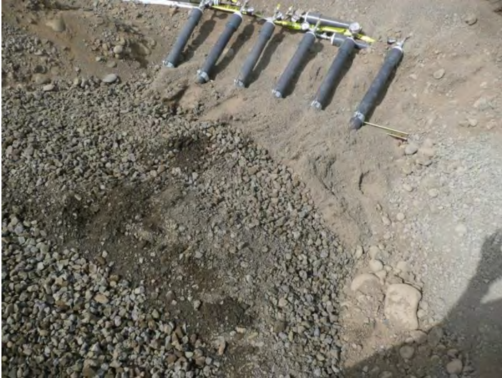
Photo 23 - Pressure testing of all upper and lower zone SVE well piping. 5/02/12
