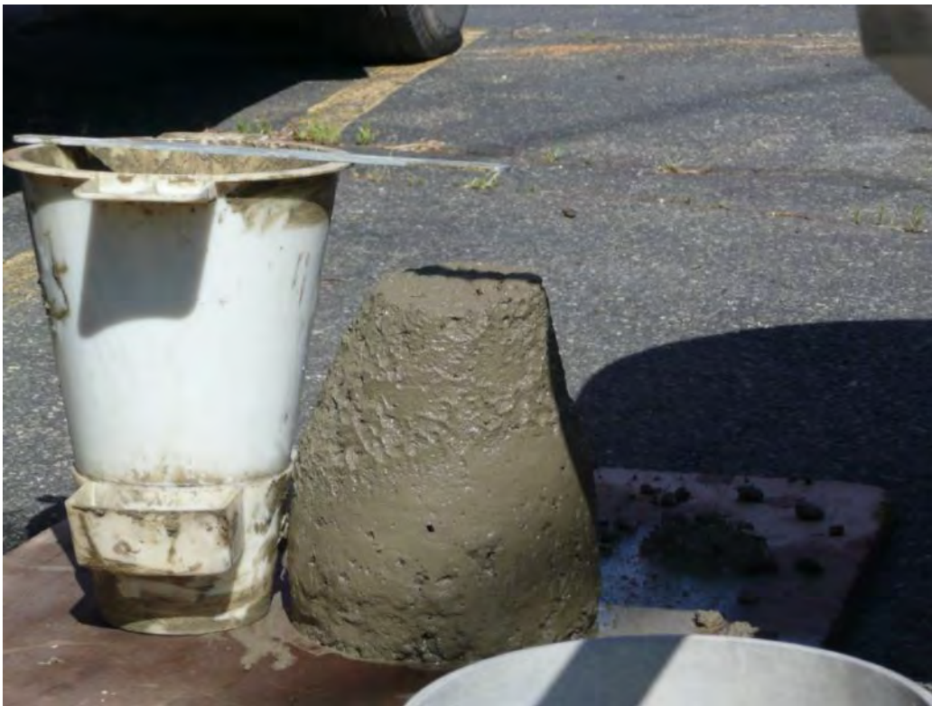
Photo 32 - Slump test, entrained air, and concrete test cylinders. 5/08/12
