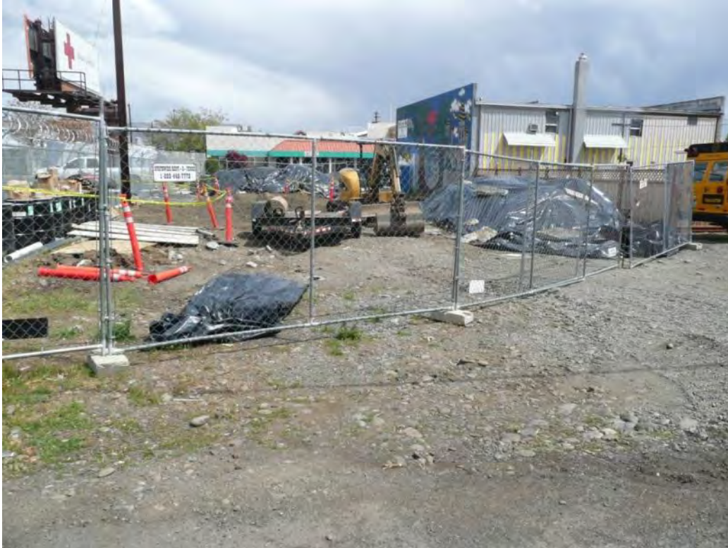
Photo 27 - Secured construction site. 5/04/12
