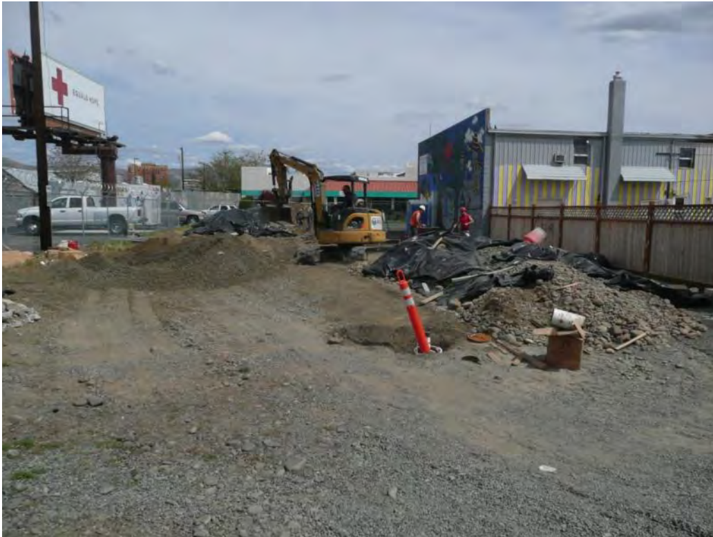
Photo 22 - SVE-1 trench backfilled and compacted. 5/02/12
