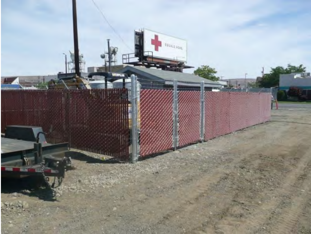
Photo 61 - Fence installed around SVE utility building. 6/21/12
