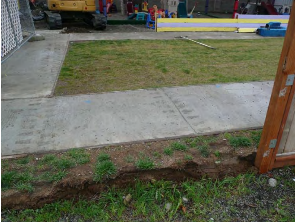
Photo 7 – Childcare center courtyard fenced-off prior to excavation. 4/26/12
