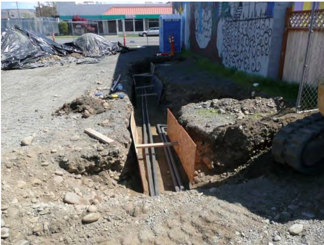
Photo 12 - Trenching to SVE-4 and SVE-5 looking east. 4/28/12
