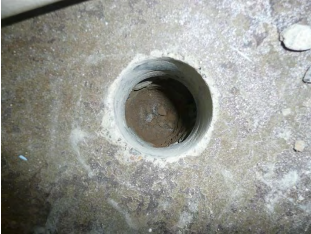
Photo 65 - View down SS monitoring point to soil under childcare center foundation. 6/22/12
