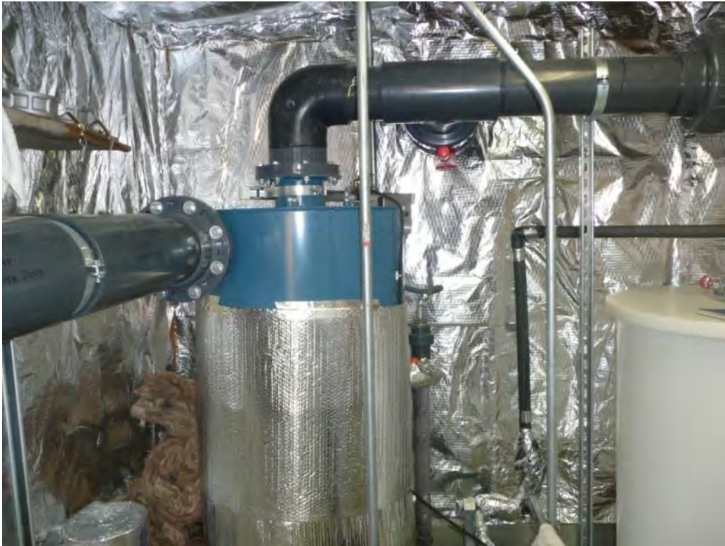
Photo 70 - VLS and double bubble foil insulation. 7/12/12
