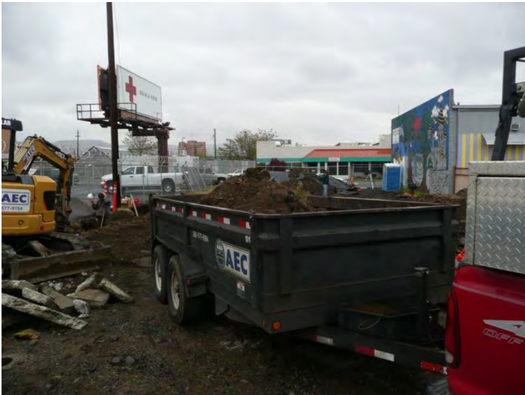
Photo 24 - Excavating for utilities: Electrical and communications. 5/03/12
