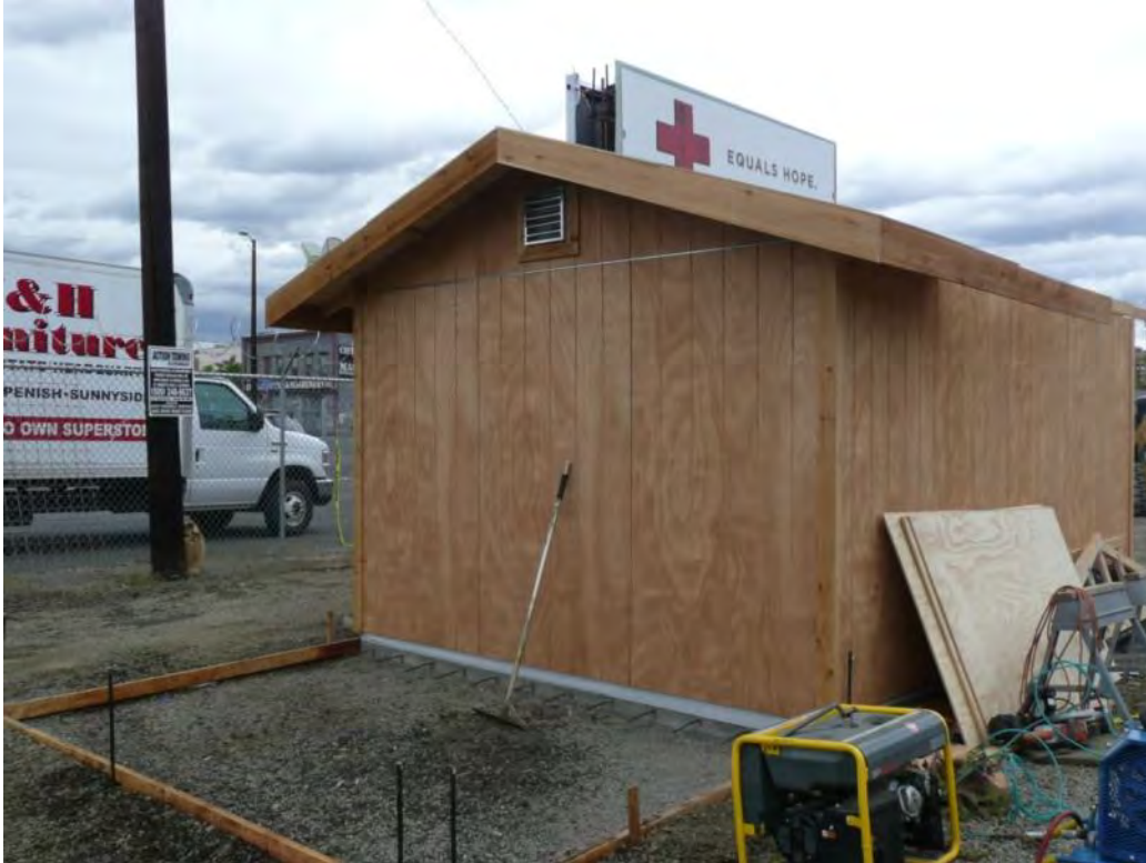
Photo 45 - Z-flashing on utility building and caulking. 5/31/12
