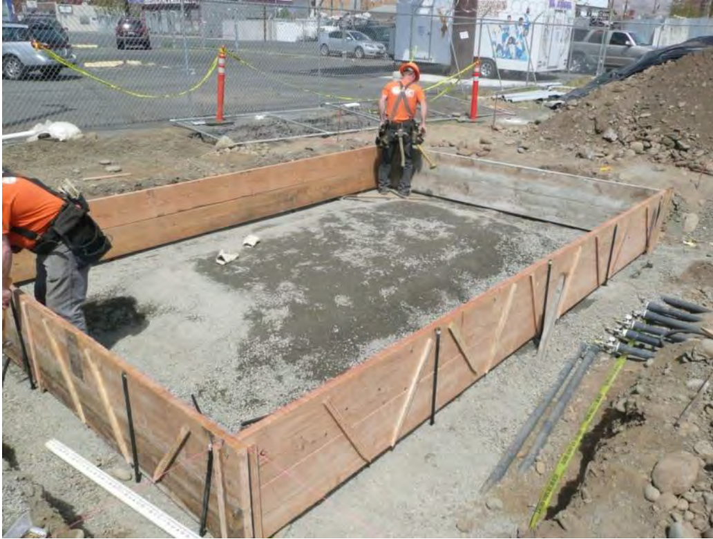
Photo 29 - Foundation with 12-inch crushed base course and formwork for concrete pour. 5/08/12
