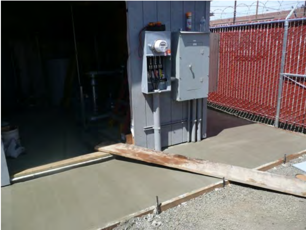
Photo 62 - Concrete entrance pad poured. 6/21/12
