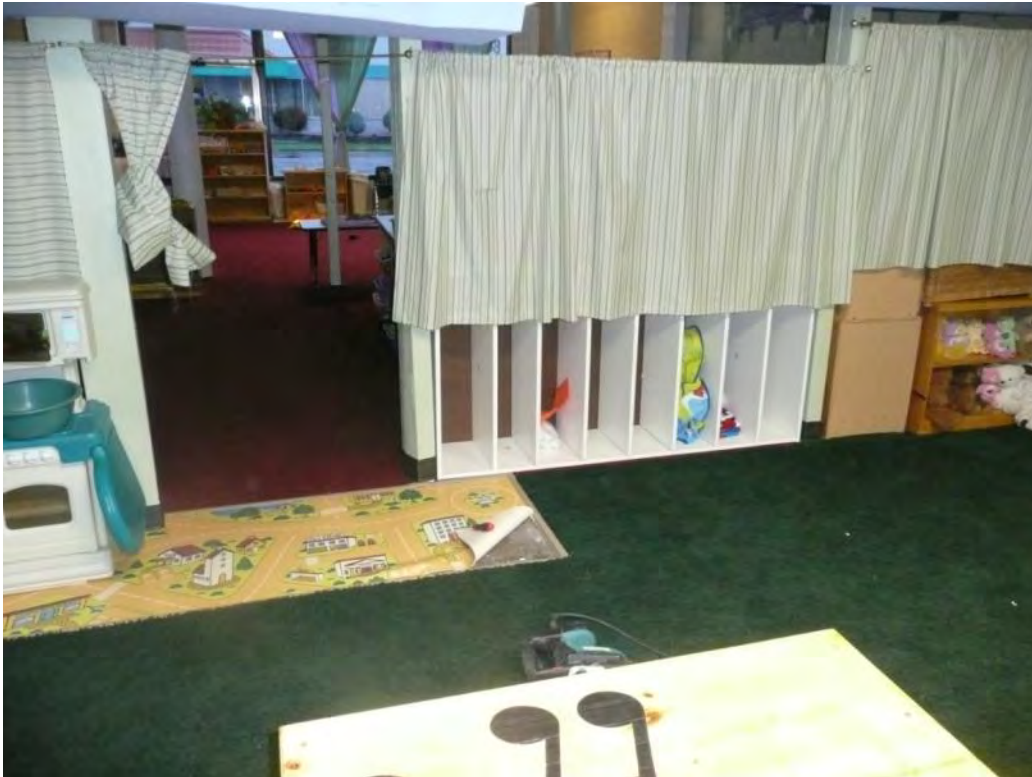
Photo 64 - Installing subslab monitoring point SS-5 inside the childcare center. 6/22/12
