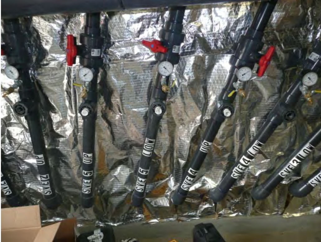
Photo 69 - Completed labeling and testing of extraction manifold. 7/12/12
