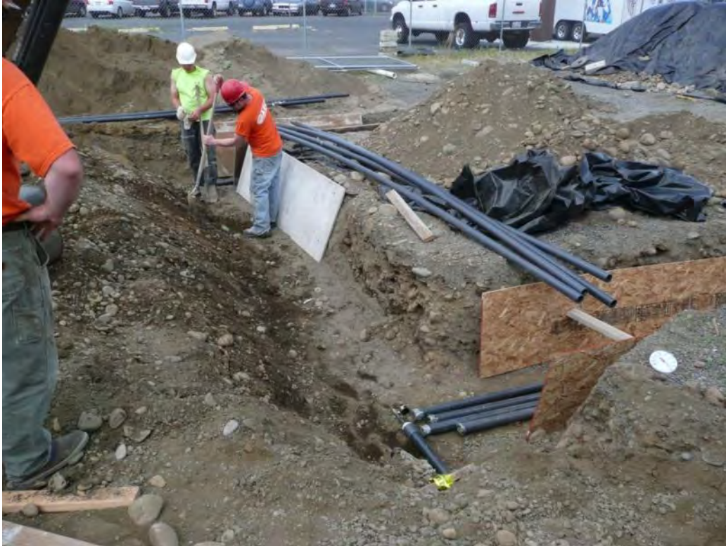
Photo 17 - Schedule 80 PVC 2-inch piping to SVE wells. Pipes on pressure test. 4/30/12
