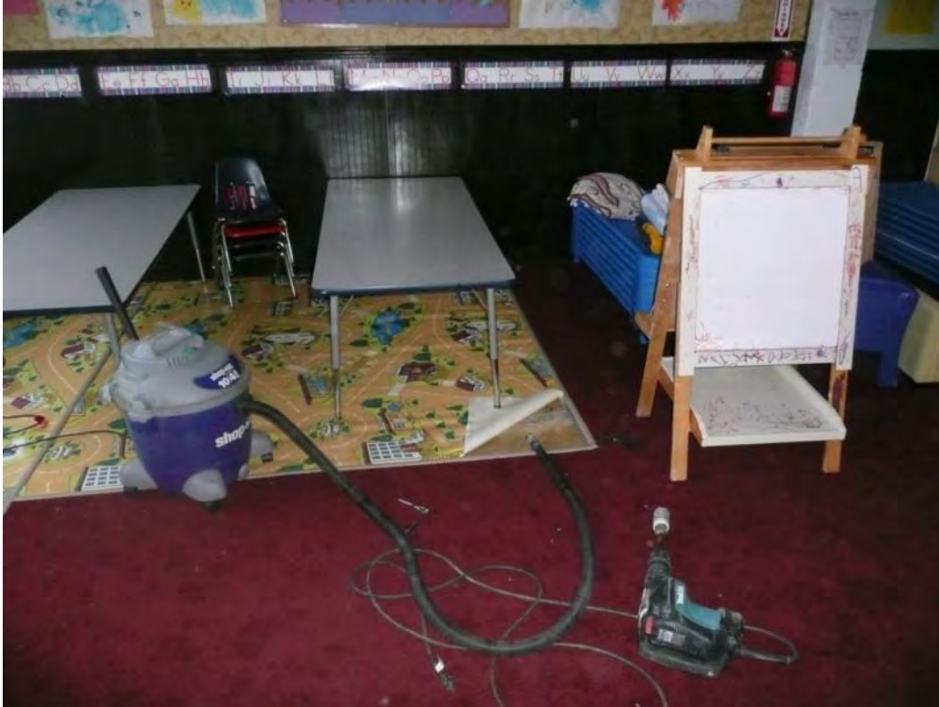
Photo 63 – Installing subslab monitoring point SS-4 inside the childcare center. 6/22/12
