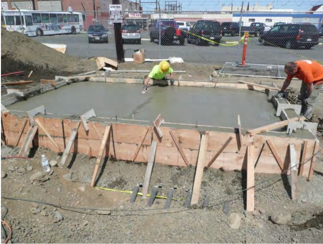
Photo 33 – Finishing for SVE utility building foundation. 5/08/12
