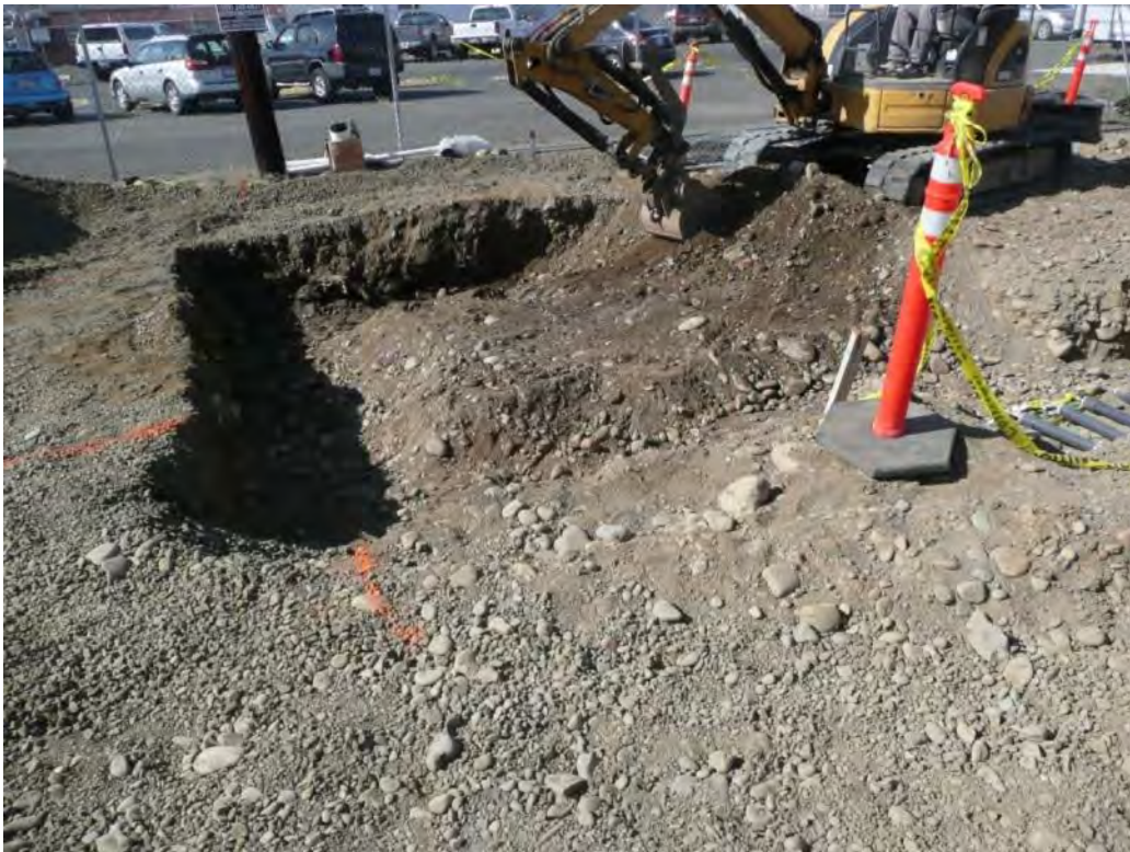
Photo 28 - Excavating for SVE utility building foundation. 5/07/12
