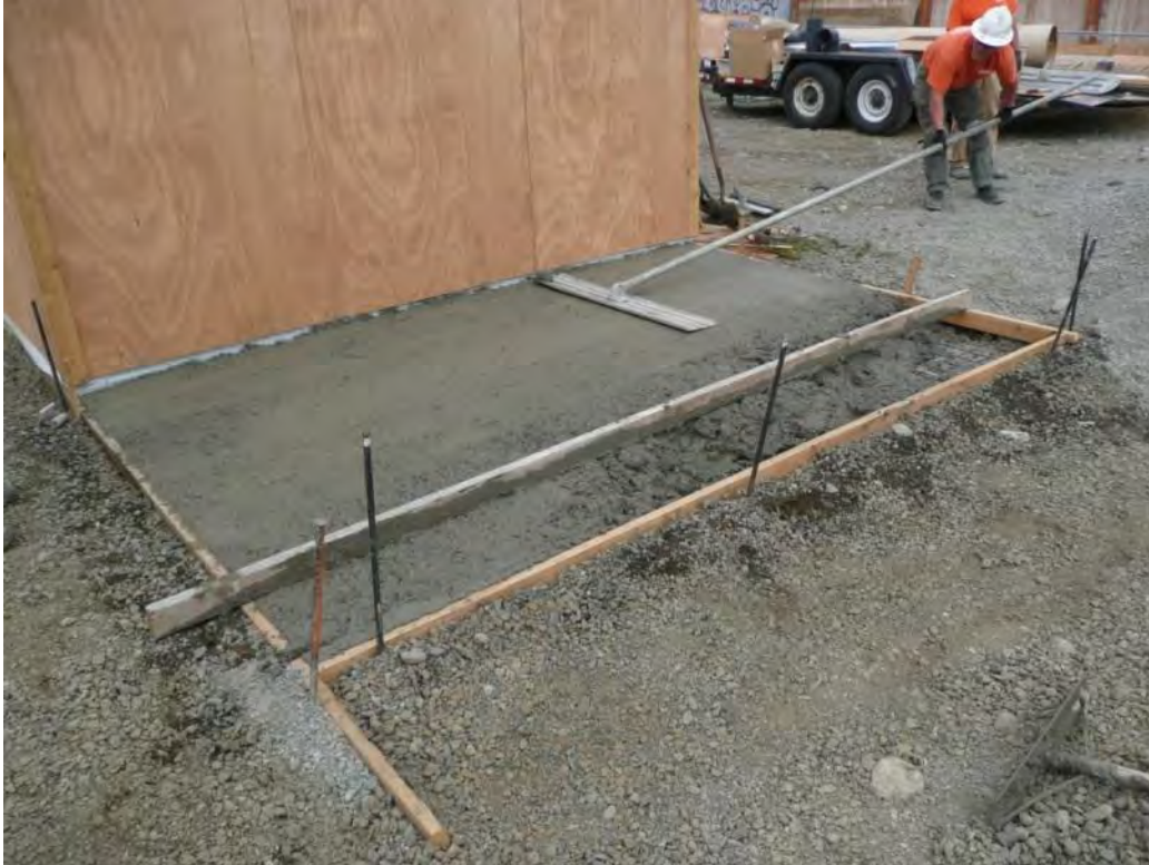
Photo 47 – GAC unit equipment pad poured. 5/31/12
