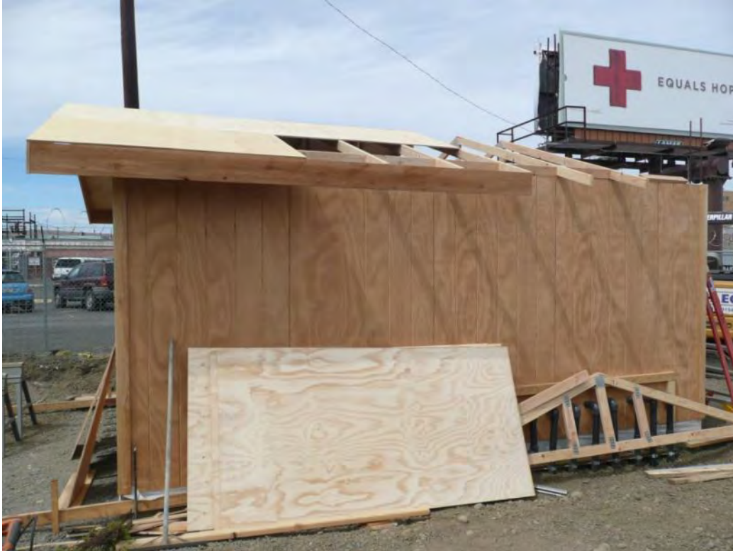
Photo 43 - Constructing SVE utility building roof. 5/30/12
