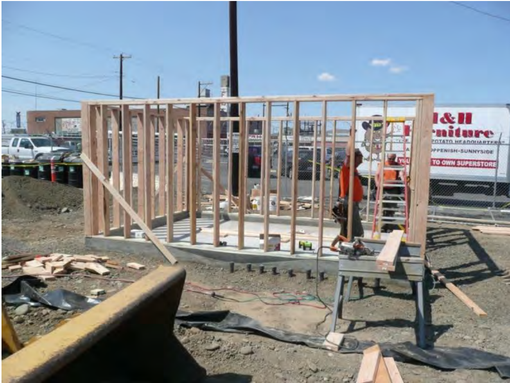
Photo 38 - SVE utility building walls. 5/17/12
