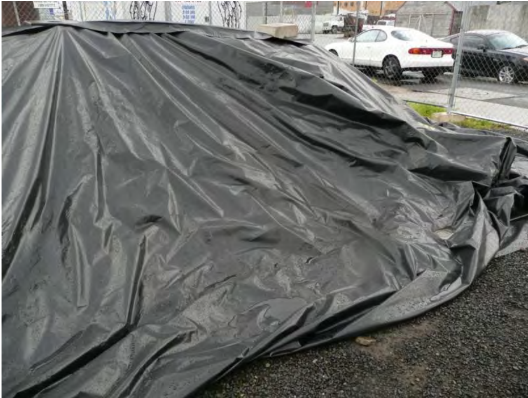
Photo 6 - Stockpiled spoils covered and weighed down. 4/25/12
