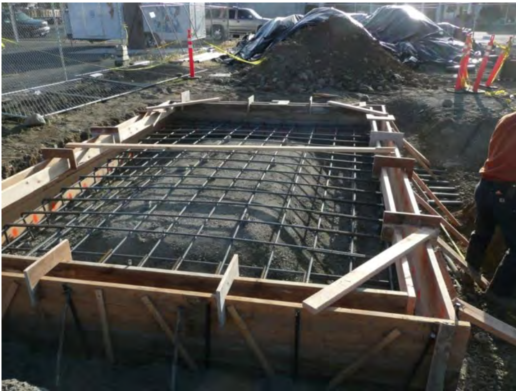
Photo 30 - Reinforced steel, #6 bar on 1 foot centers for SVE utility building foundation. 5/08/12
