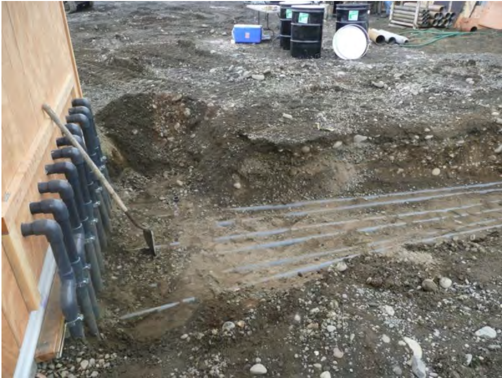
Photo 48 - Backfill material removed due to results of chemical analysis. 5/22/12
