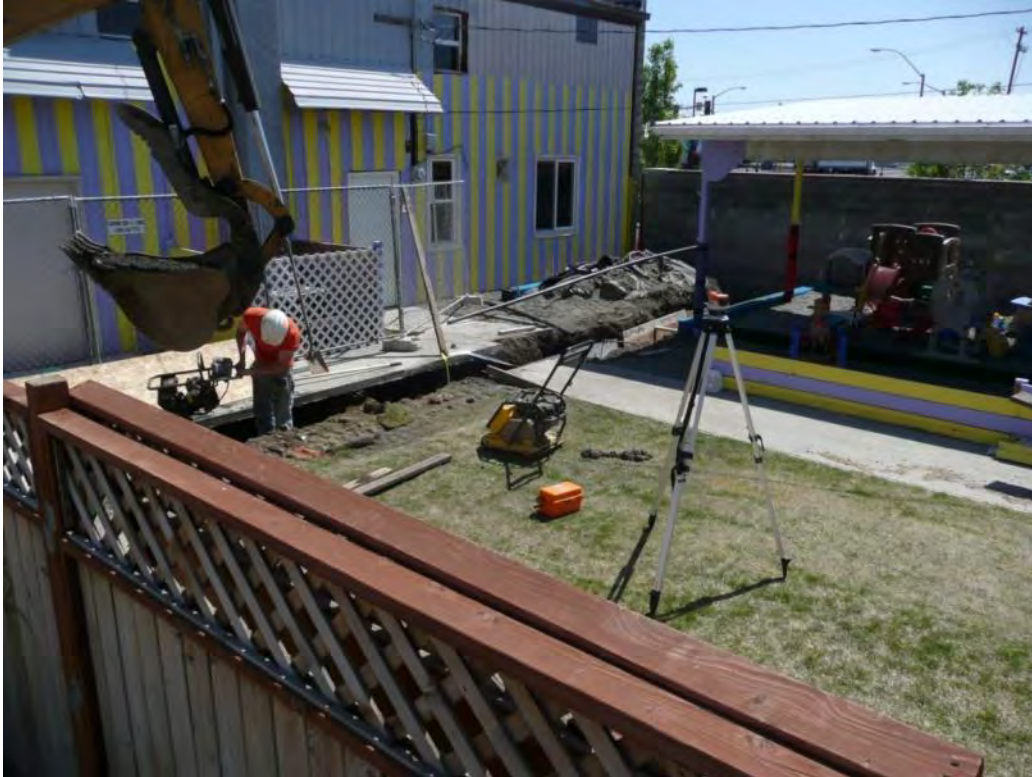
Photo 13 - Backfilling and compacting trench in childcare center courtyard. 4/28/12
