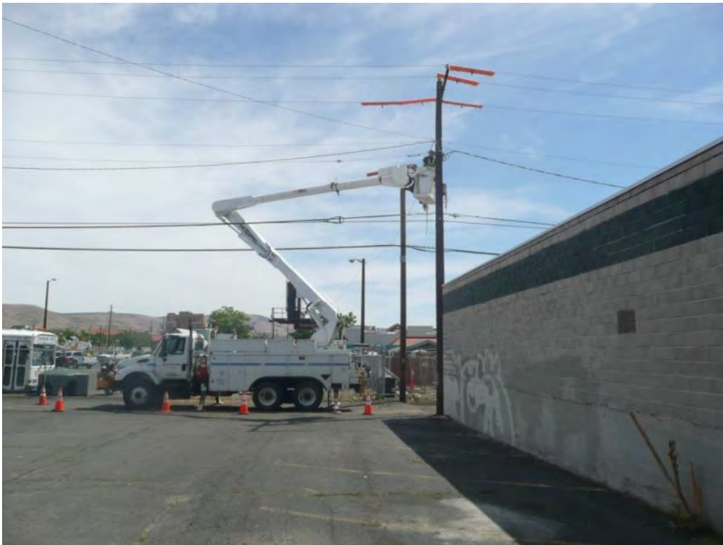
Photo 60 – Power company installing new transformers for service to SVE system. 6/21/12
