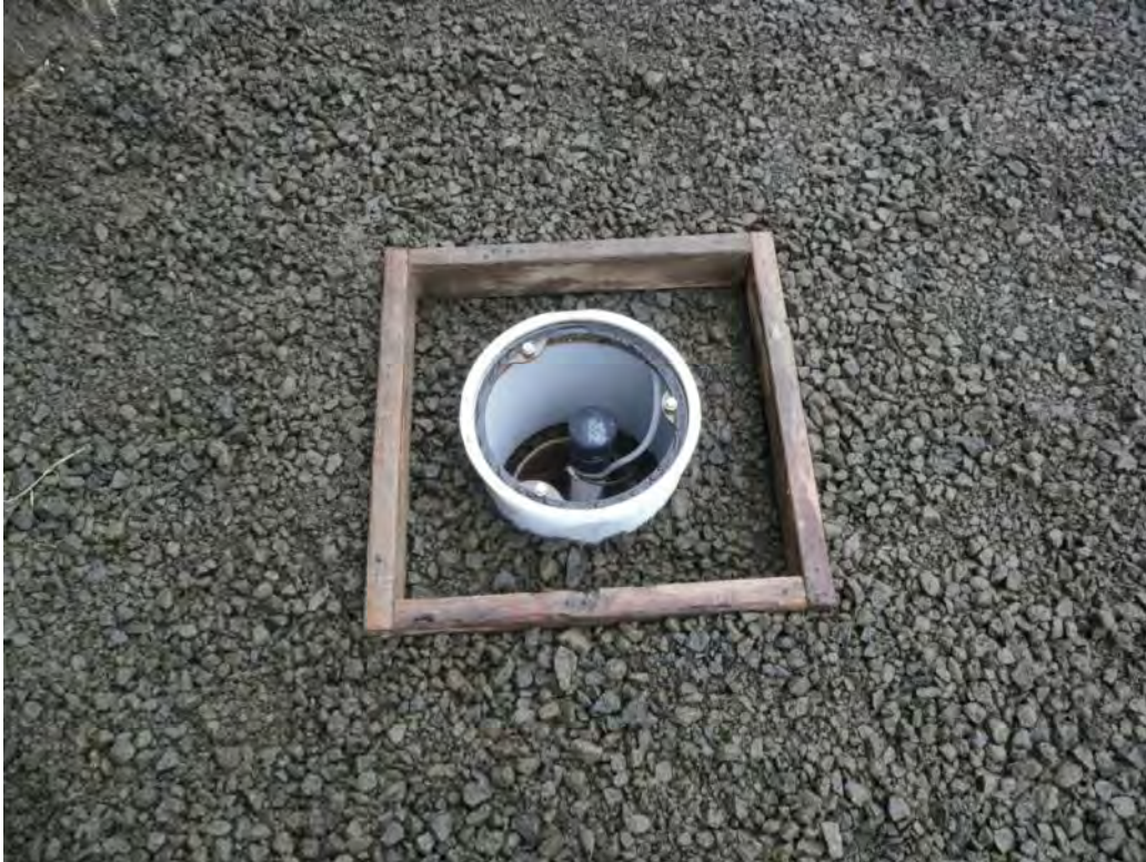
Photo 25 - Preparing well for completion with concrete monument. 5/03/12
