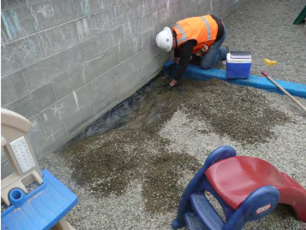
Photo 51 - Collecting additional confirmation samples for characterization of backfill material. 6/05/12
