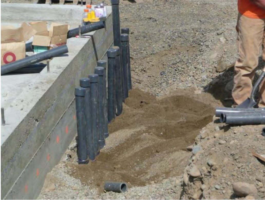
Photo 35 - Preparing piping for manifold/SVE utility building entrance. 5/15/12
