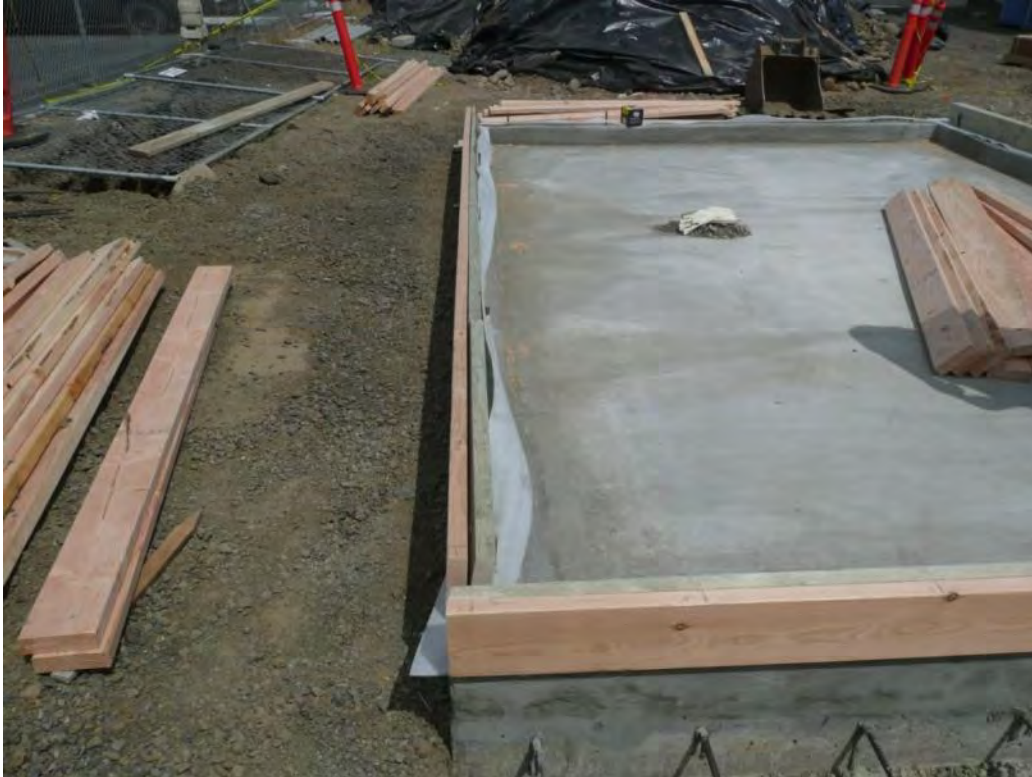
Photo 37 - Preparing for SVE utility building walls. 5/16/12
