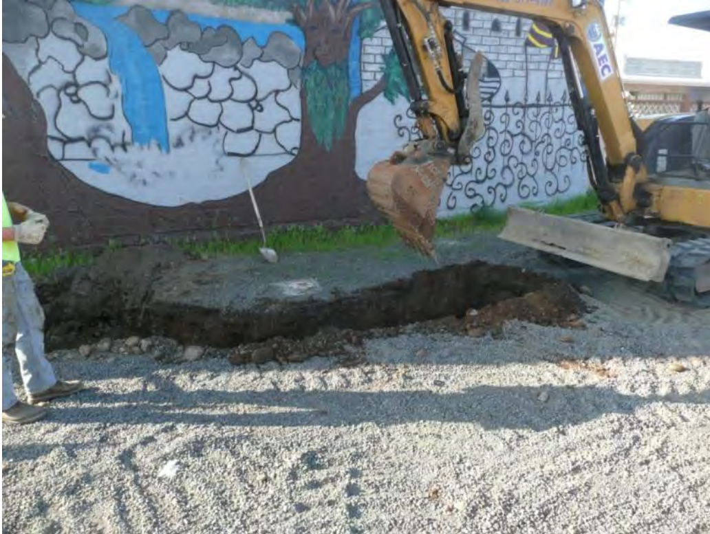
Photo 3 - Excavating SVE well trench from SVE-5. 4/24/12
