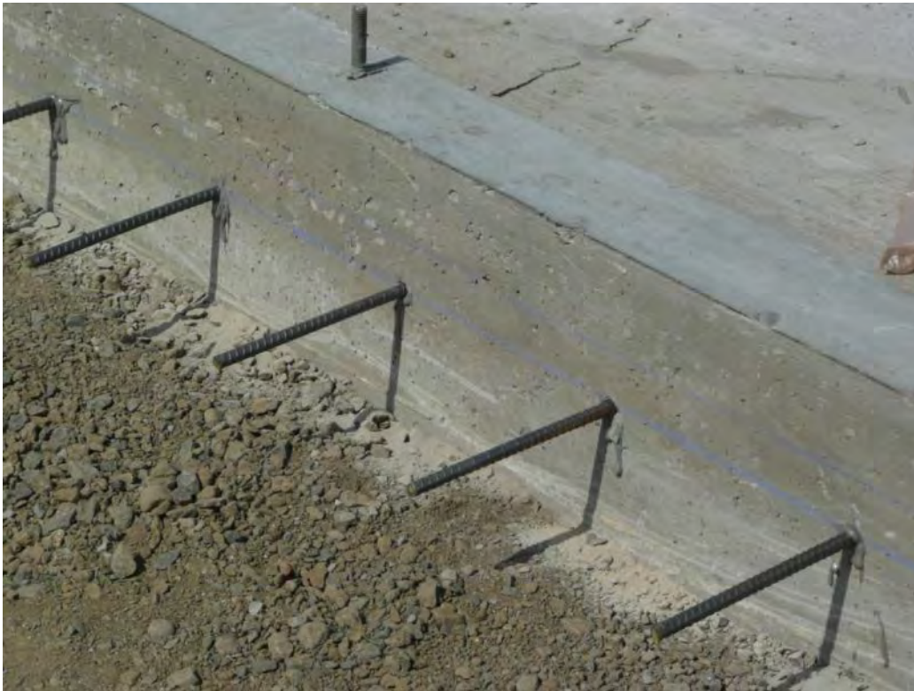
Photo 36 - Dowelled and epoxied #4 bar for GAC unit equipment slab. 5/15/12
