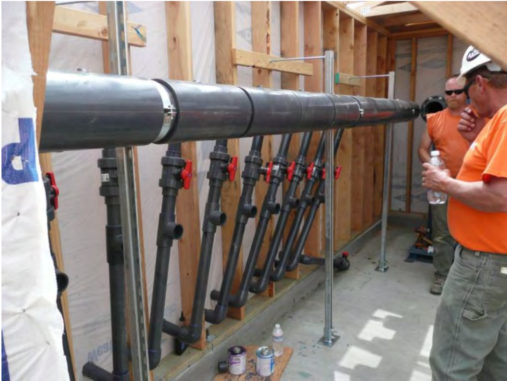
Photo 44 - Constructing utility building SVE manifold. 5/30/12
