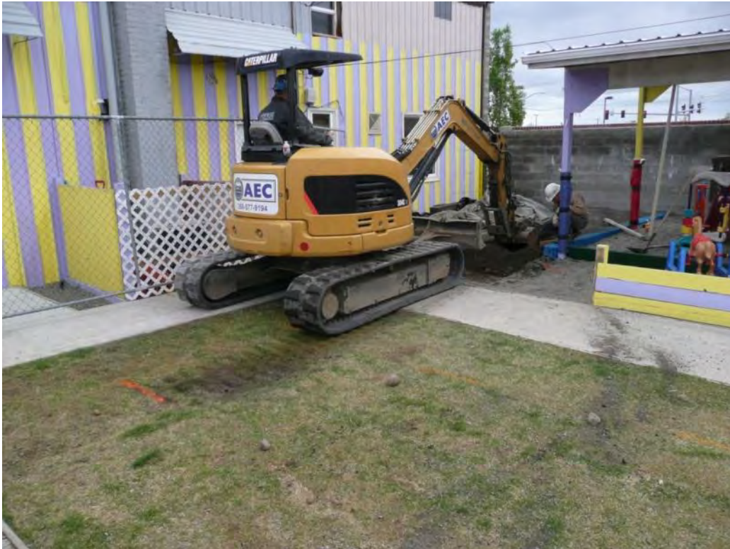
Photo 8 - Excavating in childcare center courtyard for SVE-3. 4/26/12
