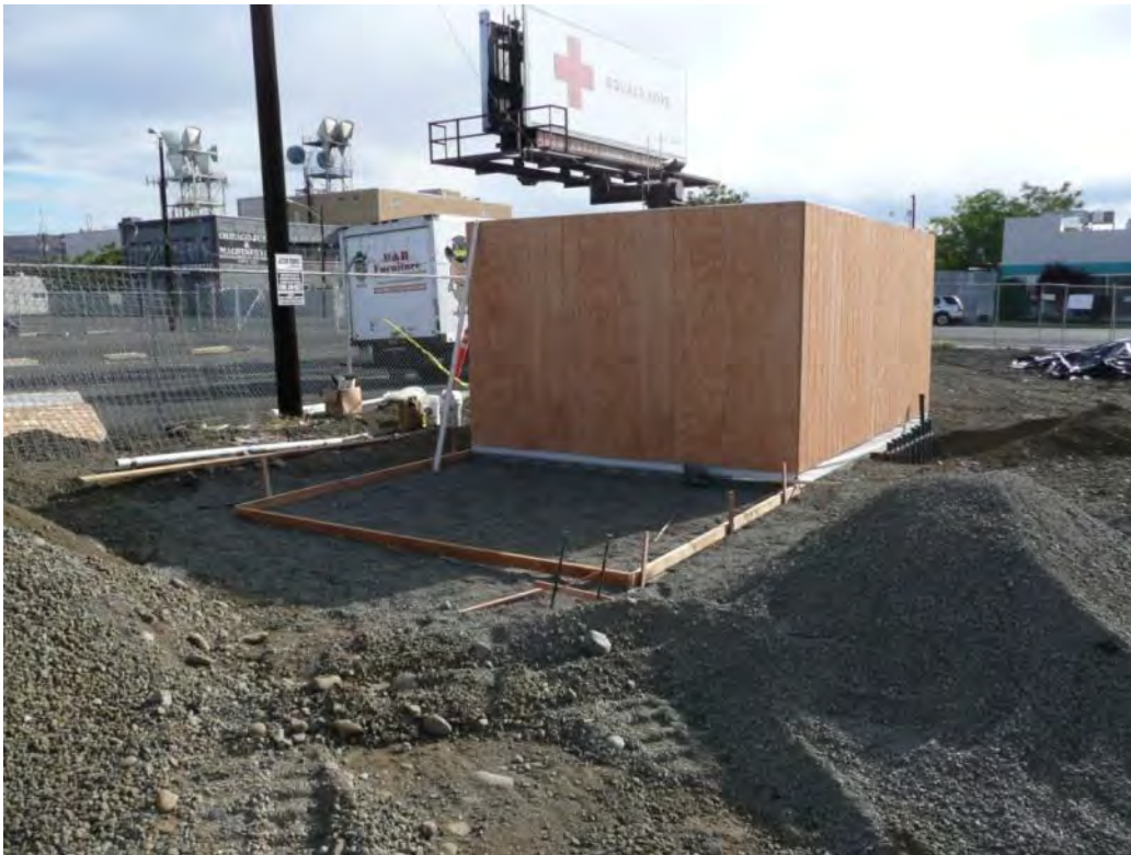
Photo 42 - Forming for GAC unit equipment slab. 5/23/12
