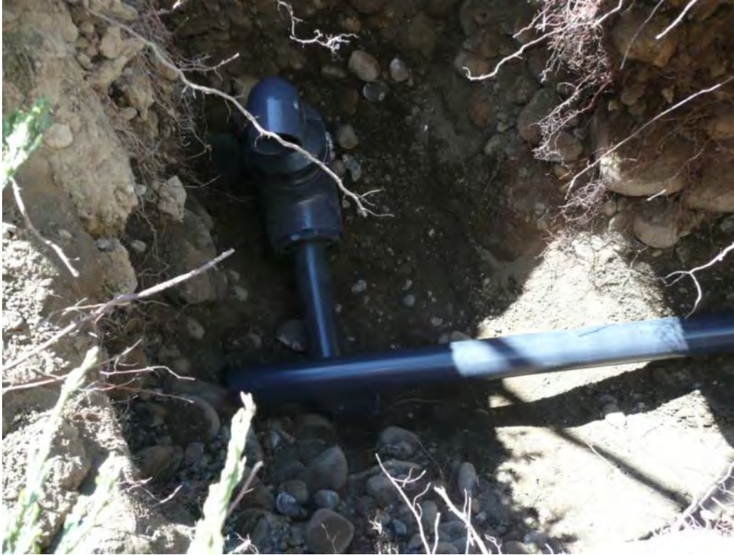
Photo 11 - Preparing pipe connections for SVE-3 well configuration. 4/27/12
