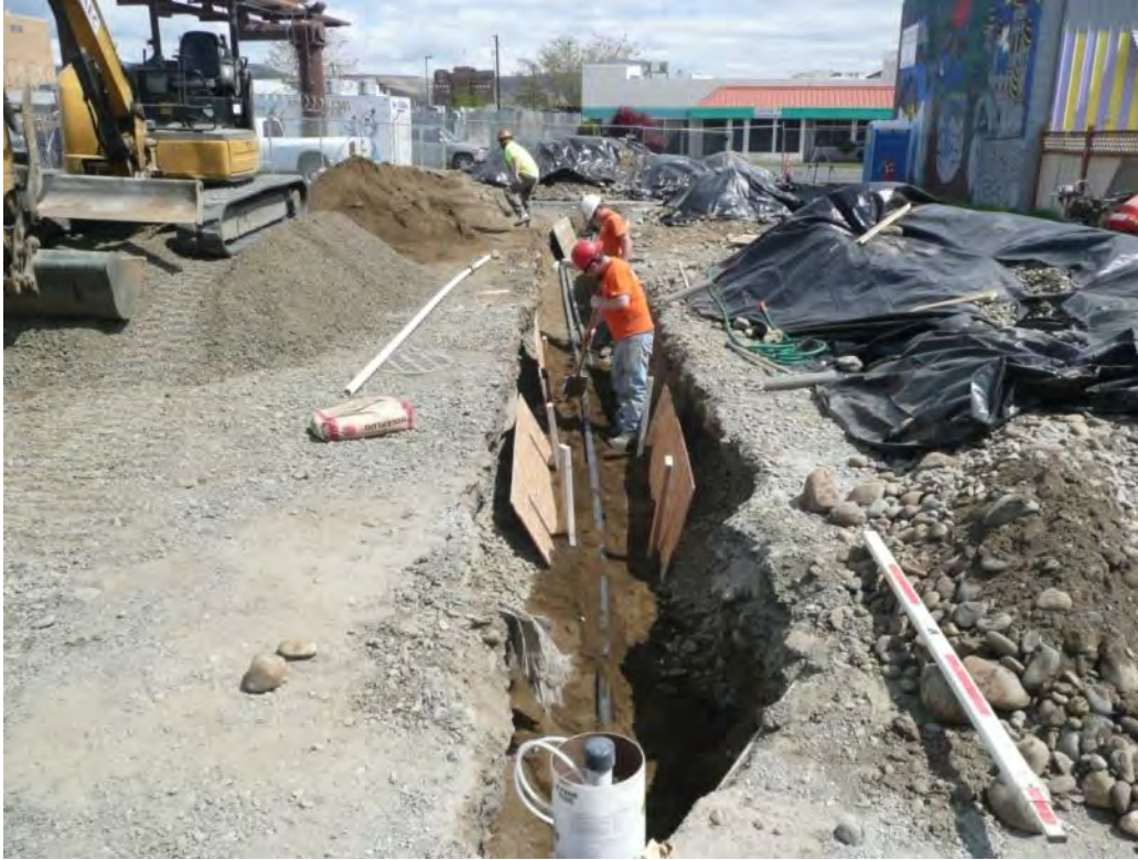
Photo 21 - Bedding piping within the trench. 5/01/12
