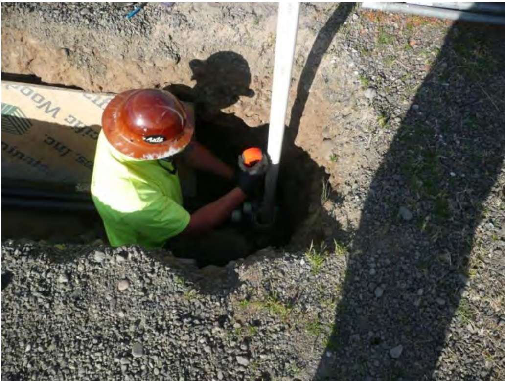
Photo 18 - Measuring placement of 2-inch drop pipe for lower zone SVE operation. 5/01/12
