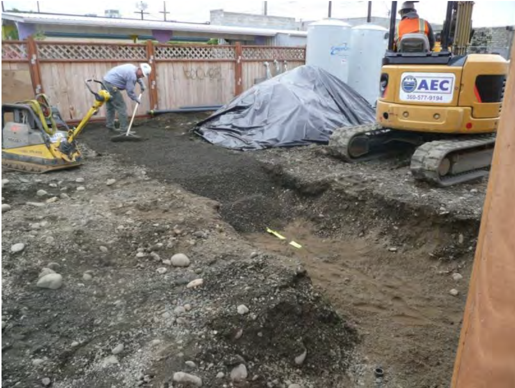
Photo 49 - Replacing removed contaminated 1-1/4-inch base course with clean 5/8-inch structural fill. 6/05/12
