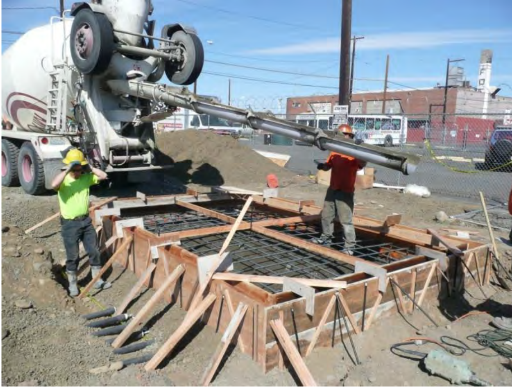
Photo 31 - Pouring concrete slab for SVE utility building foundation. 5/08/12
