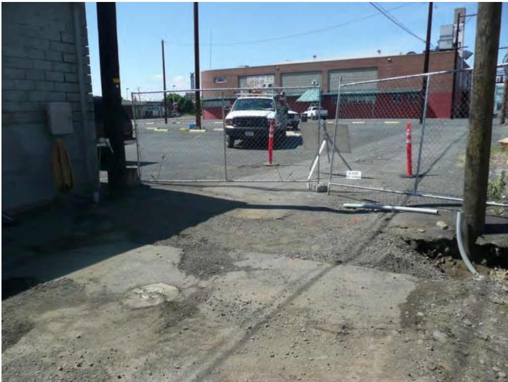
Photo 52 - Preparing to cross alleyway with utility trench. 6/06/12
