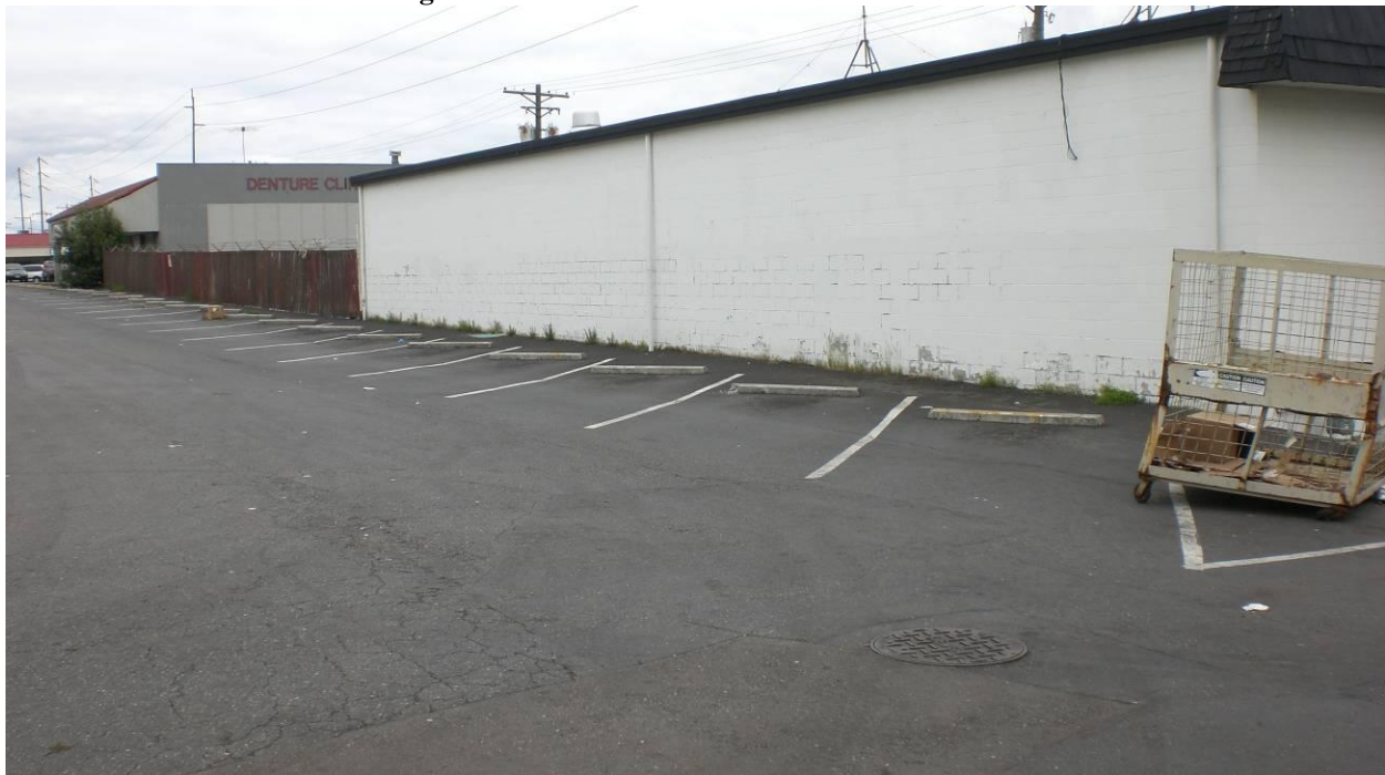
Photo 4: West Side of the Building – from the southwest
