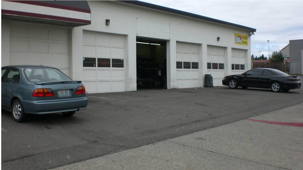
Photo 3: Service Bay Exterior – from the southeast
