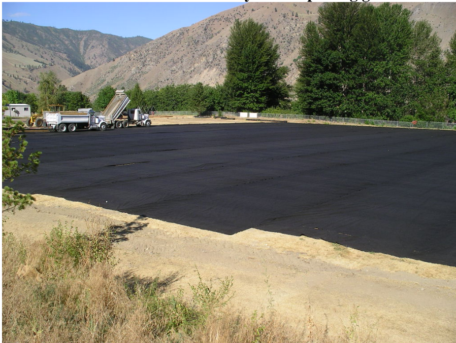
Photo D-2: Orondo Elementary School placing geotextile
