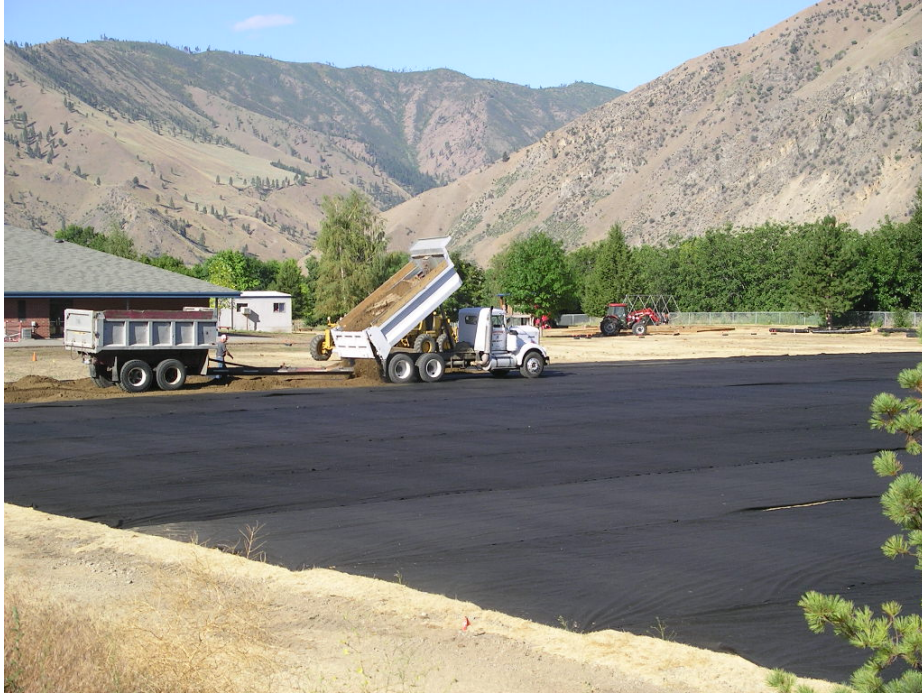
Photo D-3: Orondo Elementary School placing topsoil
