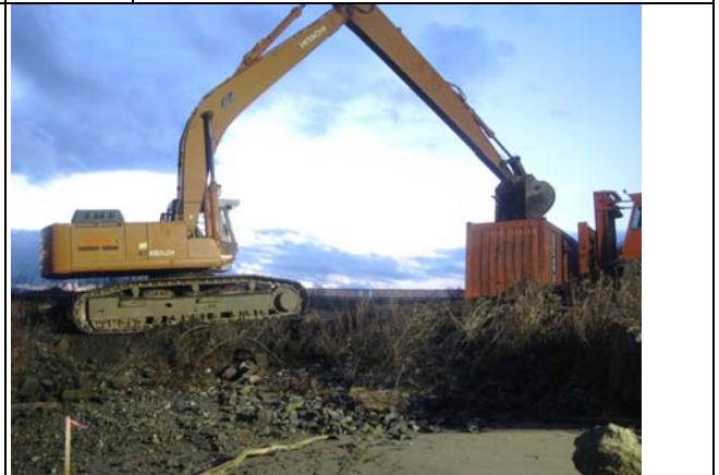
Comment: Excavating soil and placing directly into storage container.
