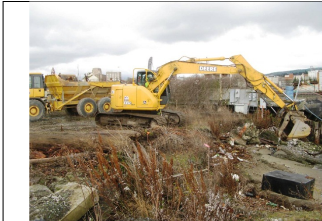
Comment: Removing wood debris from the site prior to excavation.
