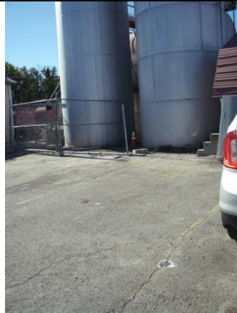
Photo #4: Location of borehole B-11 (white circle) in relation to diesel aboveground storage tanks T-1 and T-2. Photo looking southwest.
