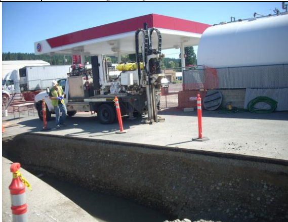
Photo #5: Borehole B-4 advanced immediately northeast of the aboveground gasoline storage tank. Gasoline dispenser canopy behind. Photo looking northeast
