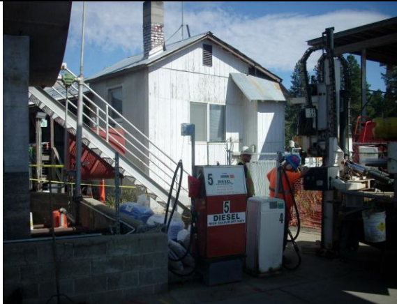
Photo #9: Borehole B-8 advanced in the immediate area of the diesel fuel dispenser pump. Photo looking southeast.
