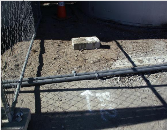
Photo #5: Location of borehole B-12 (white arrow) immediately east of the diesel fuel aboveground storage tank T-1 shown in the right above corner
