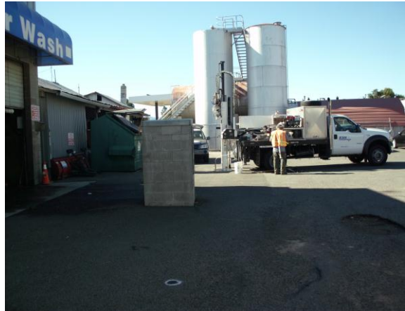
Photo #2: Location of borehole B-10 shown in white paint between the Site's Mini-mart and the carwash. Photo looking west
