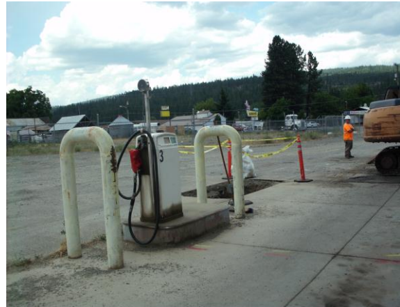
Photo #20: View looking north-northwest towards test pit west behind dispenser pump.
