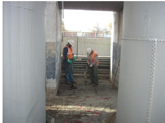
Photo #4: Borehole B-19 was hand-bored using a Rotor Hammer due to the inaccessible location of the boring beneath the split AST. Photo looking west.
