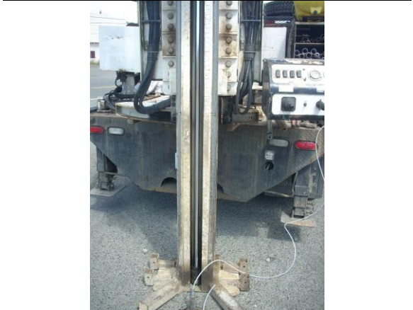
Photo #12: Stainless steel screen in the borehole and tubing inserted in the screen for groundwater sampling
