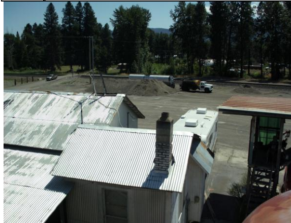
Photo #6: View looking south-southeast from location of spill.
