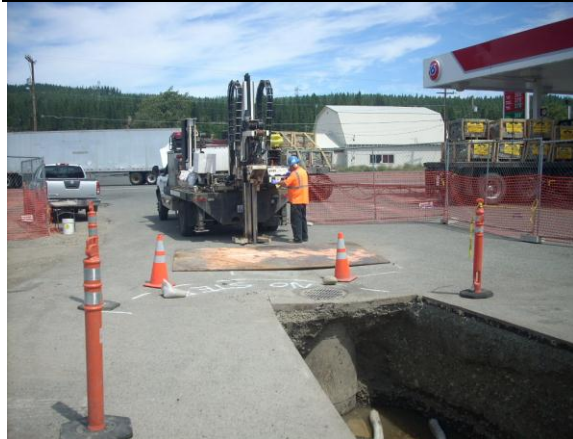
Photo #4: Borehole B-3 advanced immediately north of the "north catch basin" shown behind the Geoprobe rig. Photo looking north towards 1 st Street.
