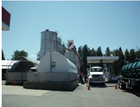
Photo #2: View looking south towards location of aboveground storage tanks (ASTs) fuel farm and location of spill at Site.
