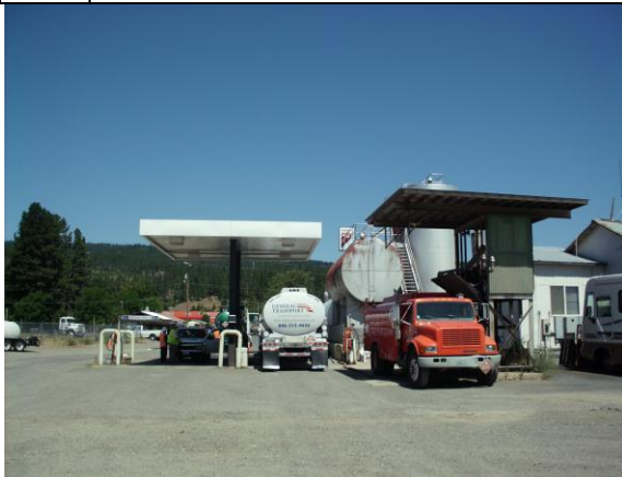
Photo #9: View looking north towards loading station, diesel fuel island w/canopy, and ASTs fuel farm where spill occurred.
