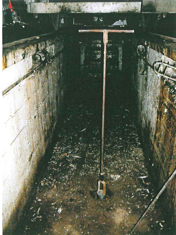
'Pit-1-S' sample location in west maintenance pit, Trolley Barn.
