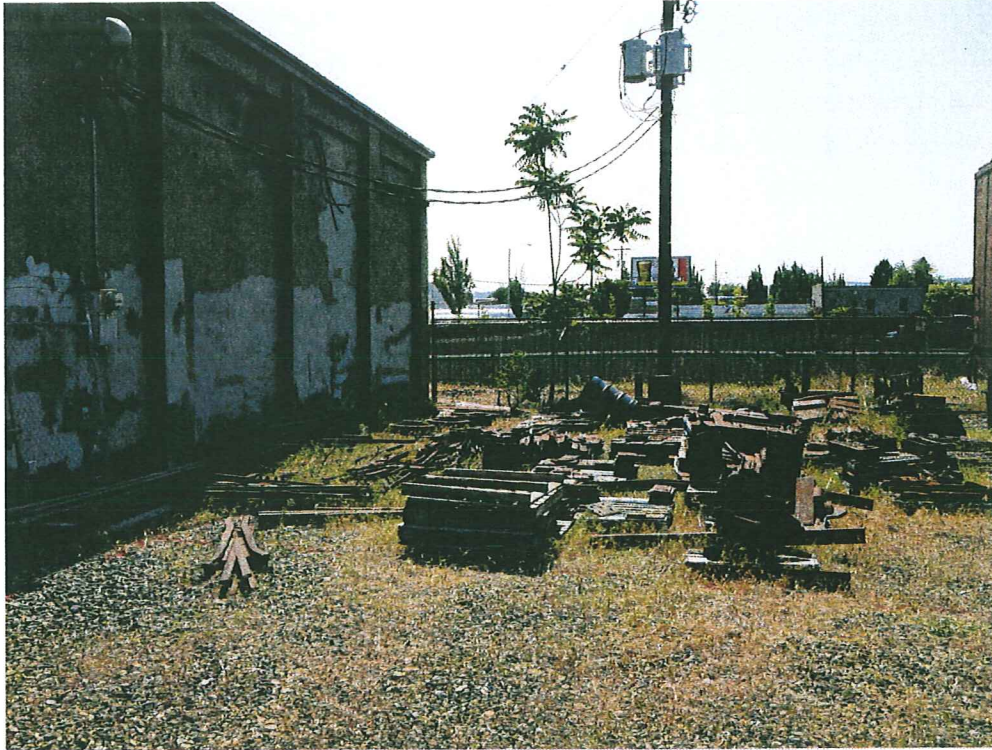
Rail yard and west side of Substation building. HWA-B1 location in foreground.
