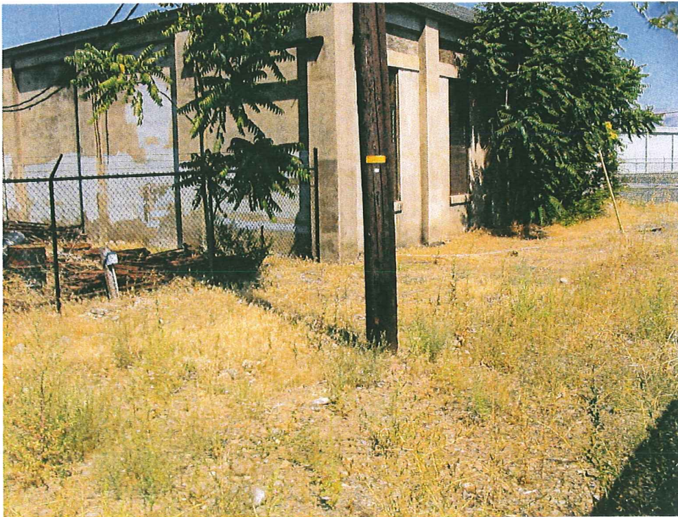
Southwest corner of Substation building. HWA-MW1 location near corner of building.
