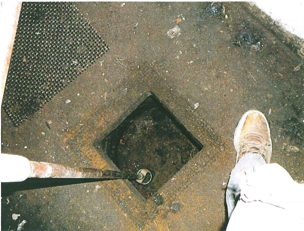
'Pit-2' sample location in east maintenance pit, Trolley Barn.
