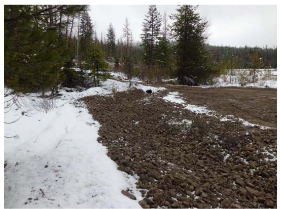
Photograph 8 – Area 2 channel condition downgradient of culvert at end of construction, 11/14/12.
