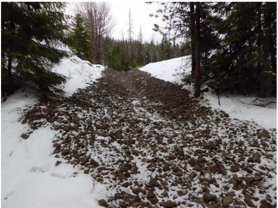
Photograph 11 – Condition of Area 2 intermediate channel at end of construction, 11/14/12.
