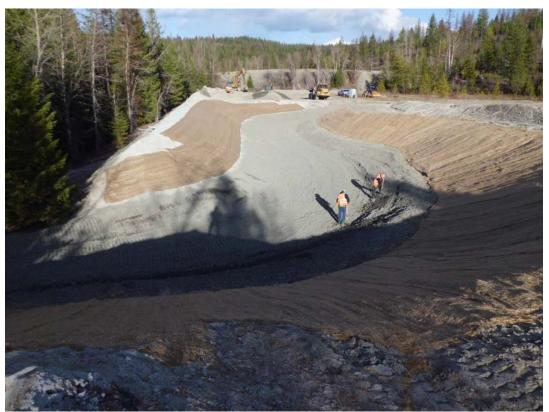
Photograph 6 – Erosion control matting placed above channel lining in Area 1, 11/07/12.
