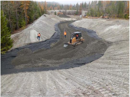
Photograph 5 – Grading the channel in Area 1, with extent of geotextile visible, 11/02/12.
