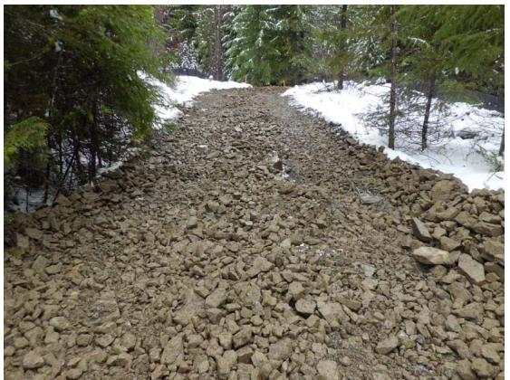
Photograph 10 – Area 1 channel condition downgradient of tailings pile toe at end of construction, 11/14/12.
