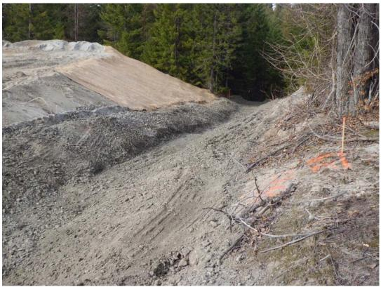
Photograph 7 – Erosion control matting placed above channel lining in Area 2, 11/08/12.
