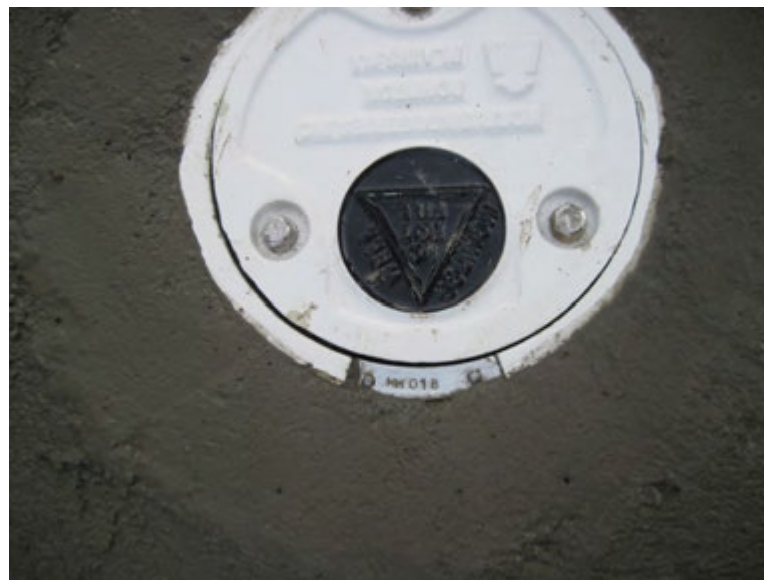
Monitoring wells were finished with flush mount monuments to prevent damage by site operations.
