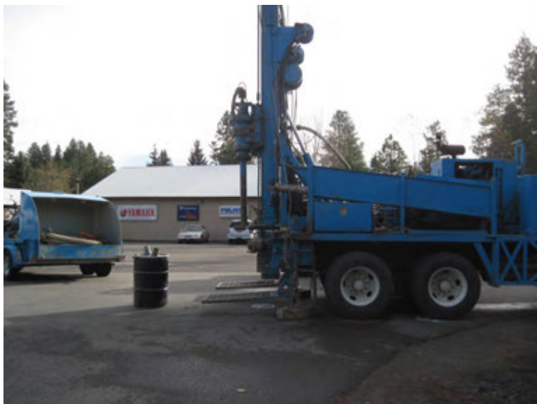
Monitoring well installation occurring with an air rotary drill rig.
