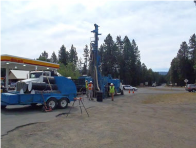
Boreholes were completed by an air rotary drilling rig.
