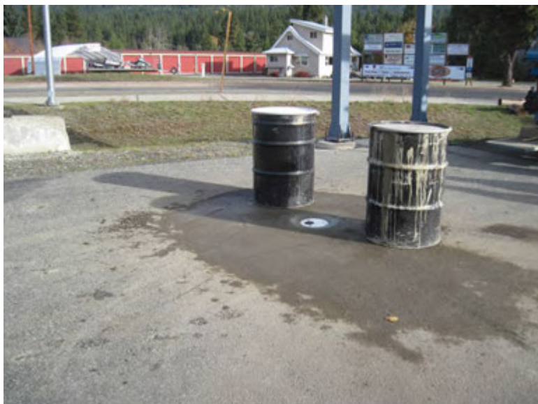
Finished monitoring wells were protected while cement hardened.
