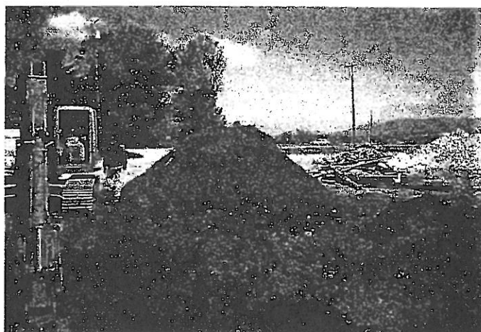
Looking northeast at gasoline-contaminated soils stockpile during over-excavation of contaminated soils.
