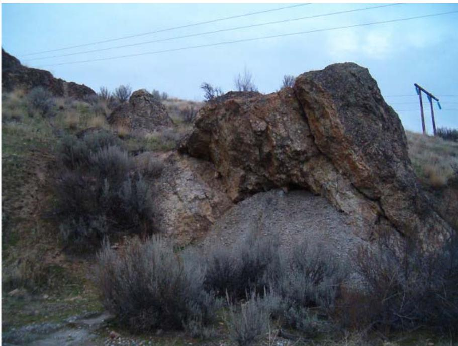
Photograph B-5 – Sealed adit at SR-02. The opening is filled with concrete.
