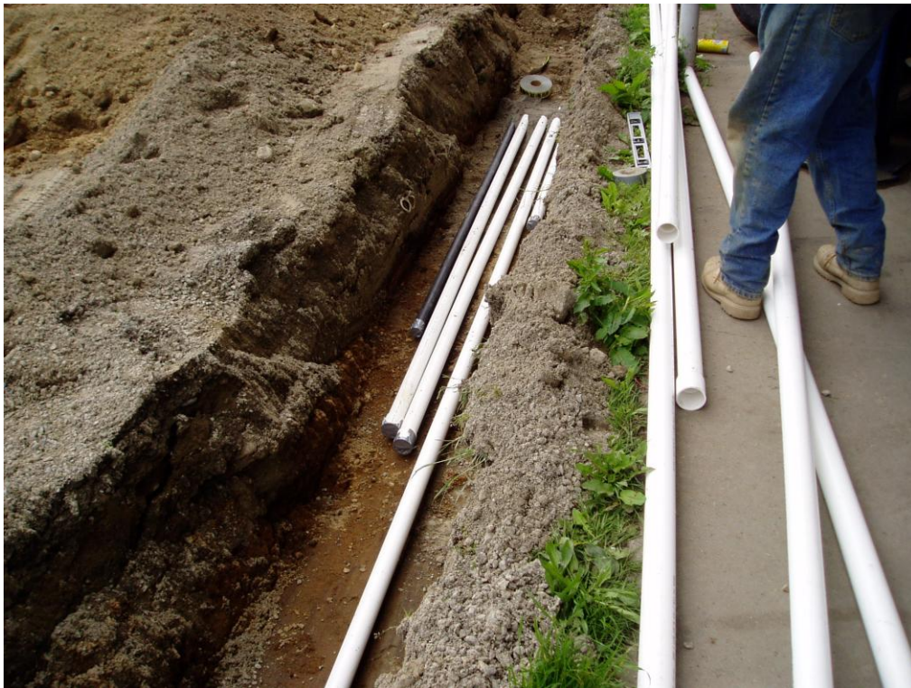
Photograph 5: Trench and SVE piping along the east property line
