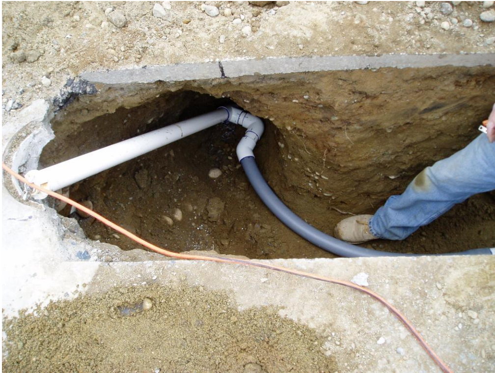
Photograph 4: SVE piping connection to angled SVE-3 well
