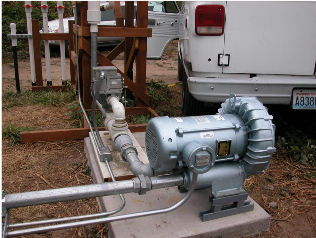
Photograph 10: SVE blower with water knock-out and SVE manifold in background
