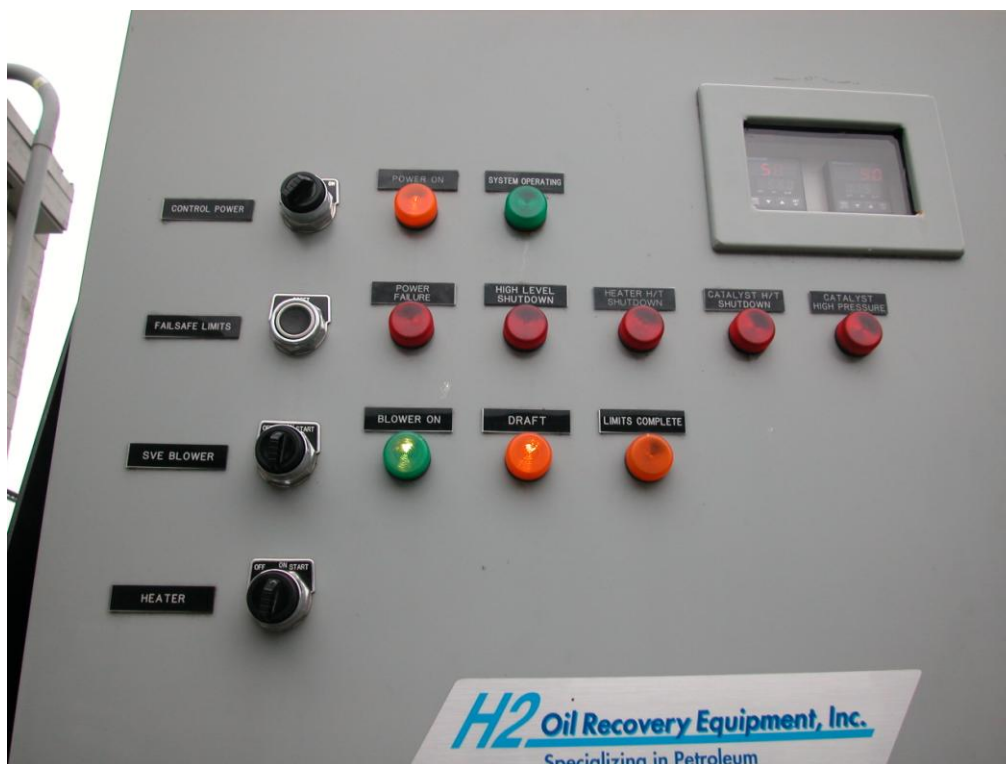
Photograph 12: Catox Control Panel
