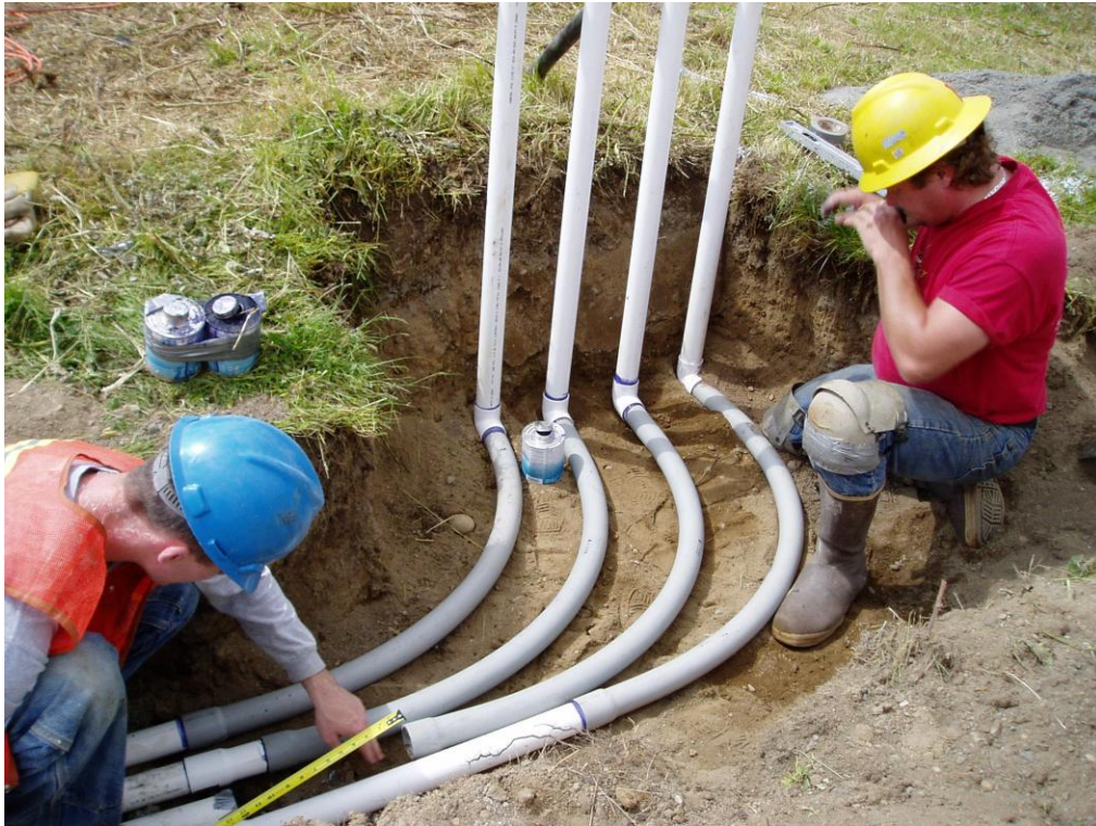
Photograph 6: End of SVE piping in trench
