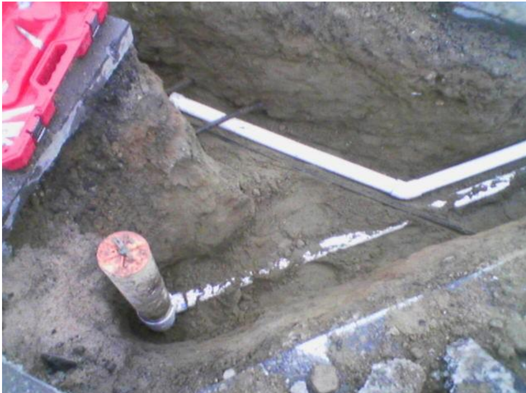
Photograph 2: SVE piping connection to 4-inch well MW-1/SVE-1
