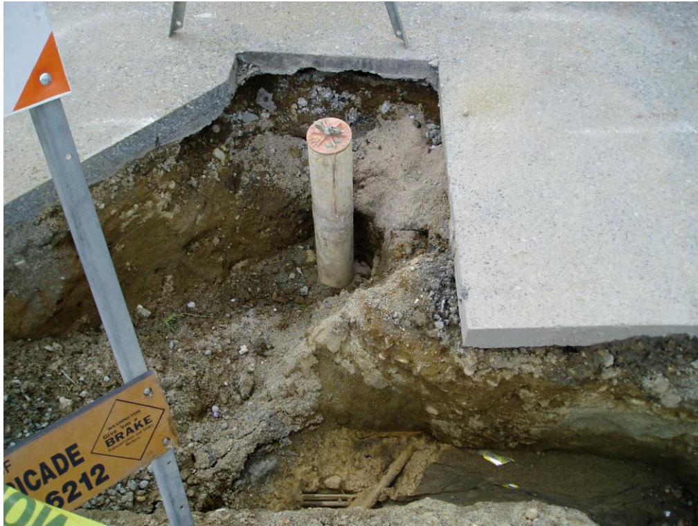
Photograph 1: MW-1/SVE-1 (4 inch well casing)
