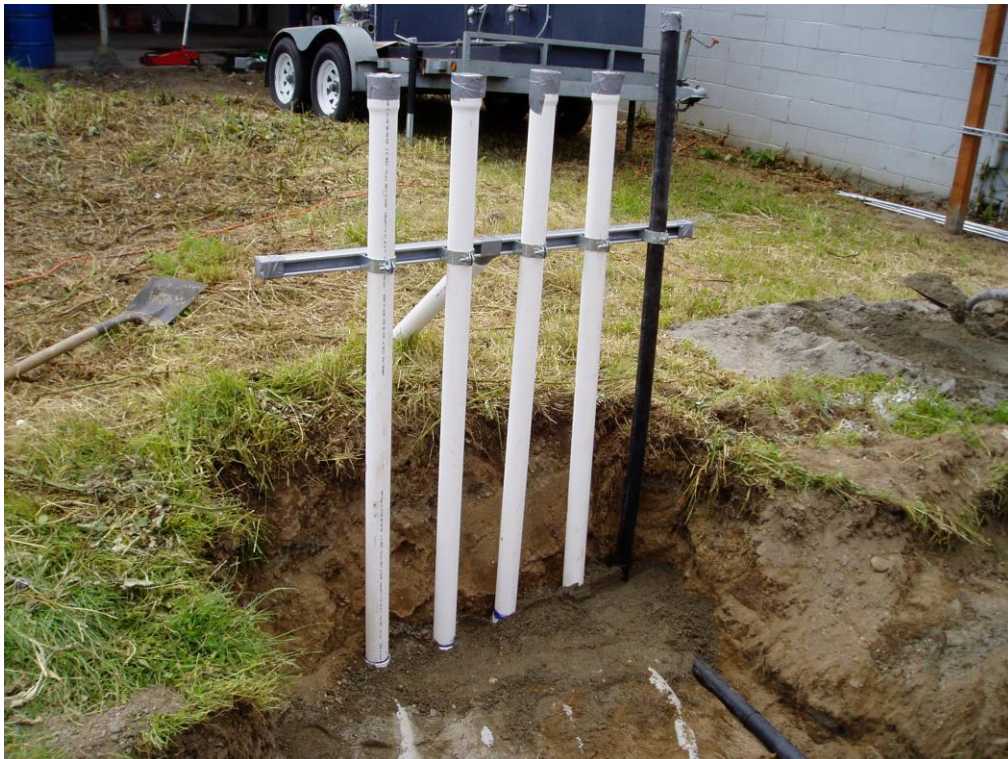
Photograph 7: SVE manifold, trench partially backfilled
