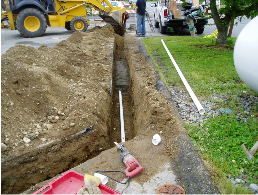
Photograph 3: Trench with line for SVE-3
