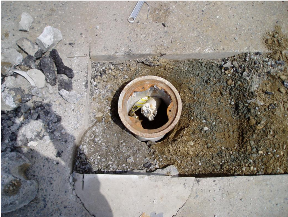
Photograph 8: Angled well SVE-3 backfilled and monument set over well head
