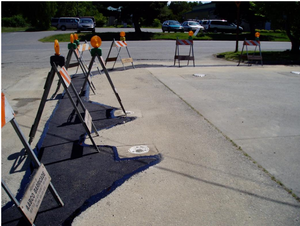
Photograph 9: Trench backfilled and paved, SVE-2S and SVE-2D in the foreground
