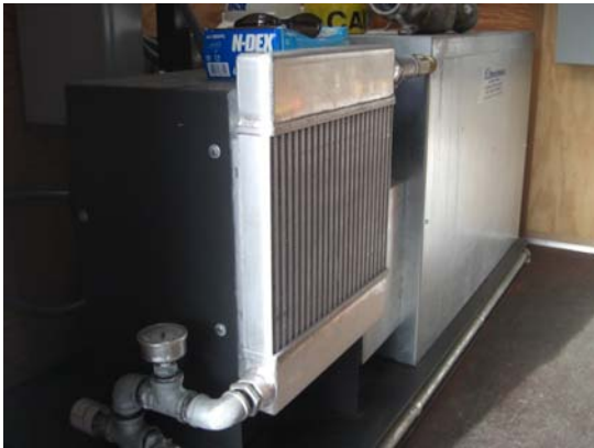
Sparge pump sound enclosure with Intercooler and pressure gauge.
